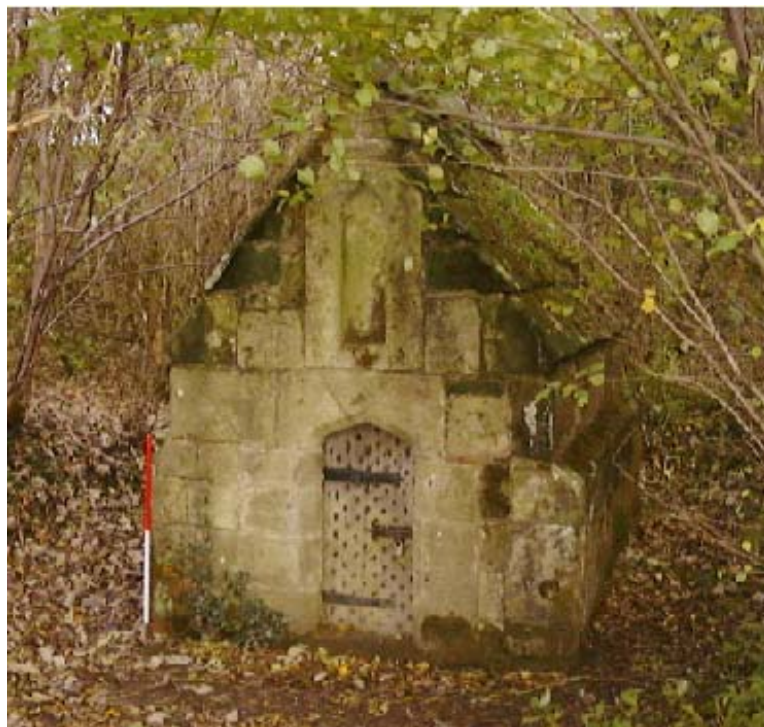
Figure 16. The conduit house viewed from the west
