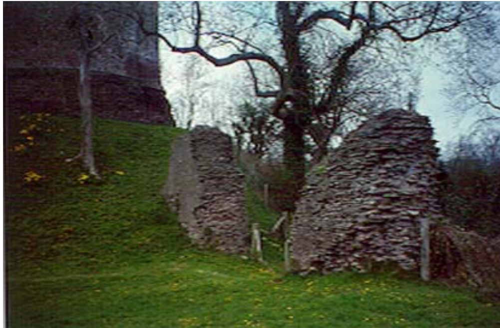
Figure 6: fragments of curtain wall on the eastern side of the inner bailey
