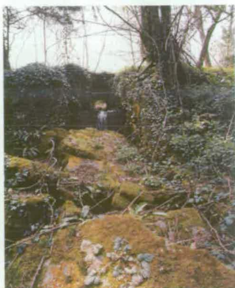
Figure 21 Wheel pit of incorporating mill [16], this feature is typical of the remains in this area (AA044432). (c) English Heritage
