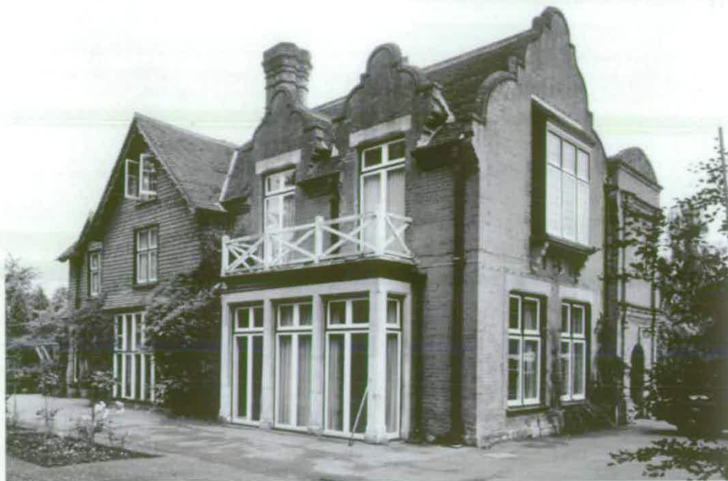
Figure 8 The Old Manor House (BB94/10124). (c) Crown copyright.NMR
