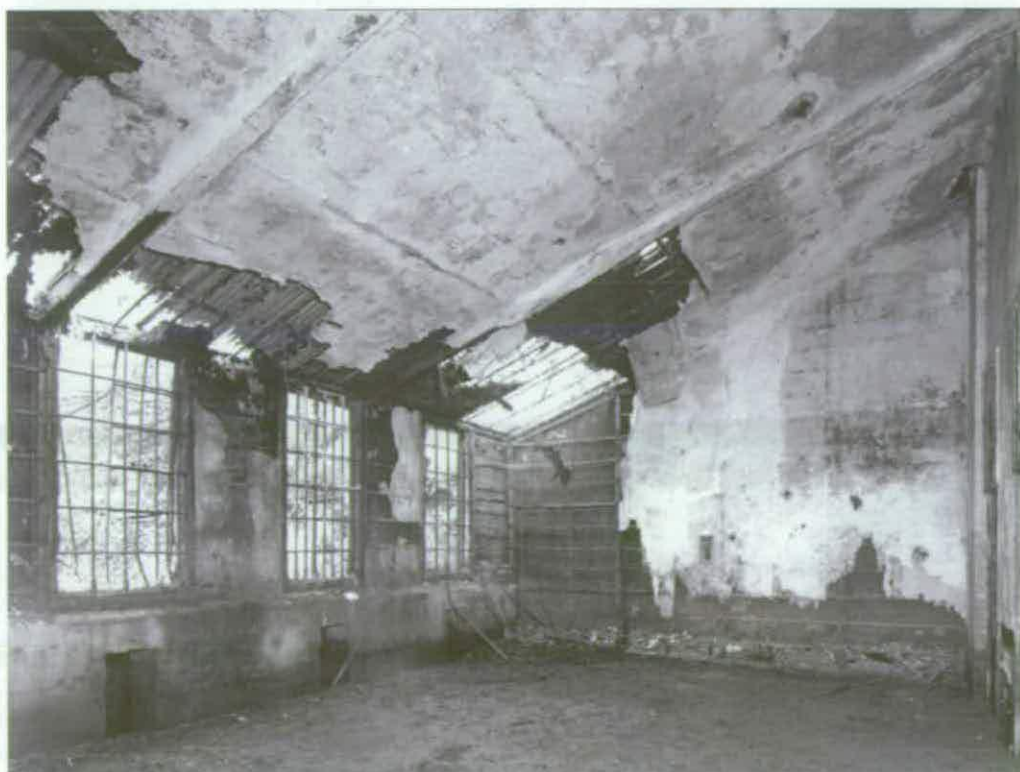
Figure 36 Interior of cordite drying stove (BB94/ 10120). (c) English Heritage
