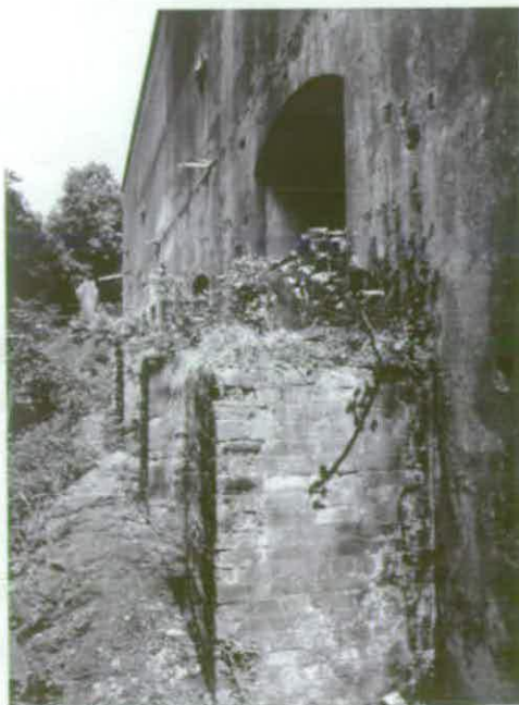
Figure 26 1880s incorporating mills [52], showing the piers that supported the rear drive shaft (BB94/10121). (c) English Heritage
