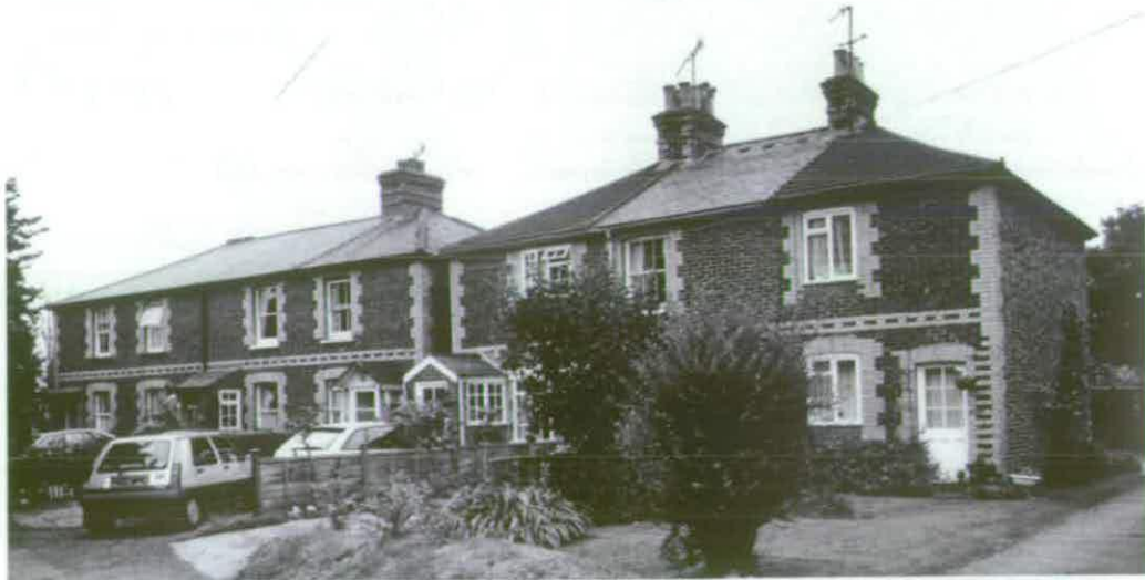
Figure 11 Magazine Cottages (BB94/10130). (c) Crown copyright. NMR
