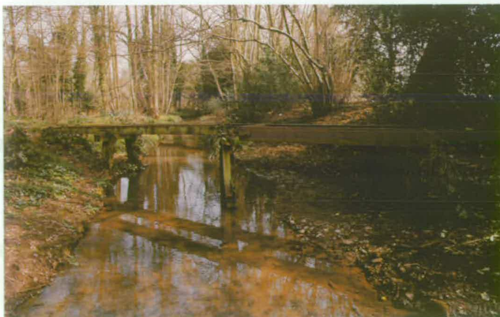
Figure 44 1880s tramway bridge [BR16] crossing New Cut (AA044439). (c) English Heritage
