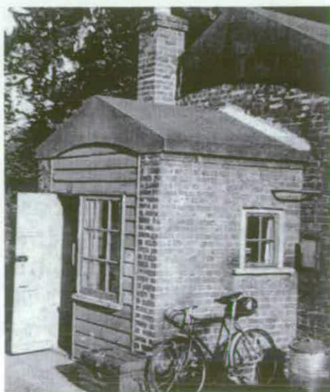
Figure 22 1950s view of ?magazine [60], showing its thick mass concrete roof. (c) Mr & Mrs Moseling
