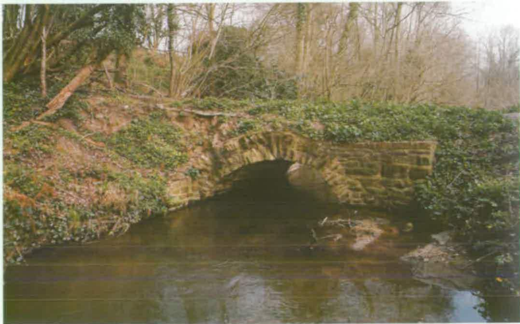
Figure 17 Packhorse bridge [BR 12] (AA04444). (c) English Heritage
