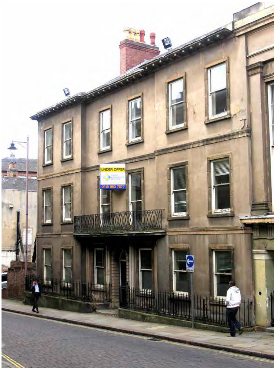
Fig. 11. County House, High Pavement. Remodelled Wood & Nicholson 1833, Pete Smith 2008.
