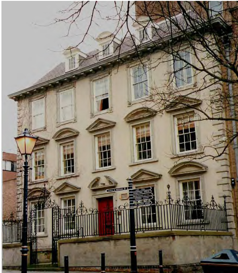
Fig. 8. Newdigate House, Castle Gate. Pete Smith 2005.
