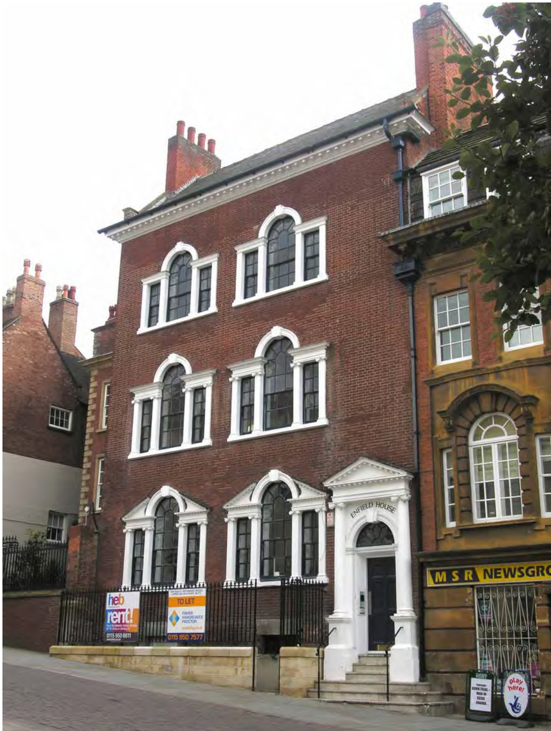
Fig. 18. Enfield House, No. 18, Low Pavement. Pete Smith 2008.
