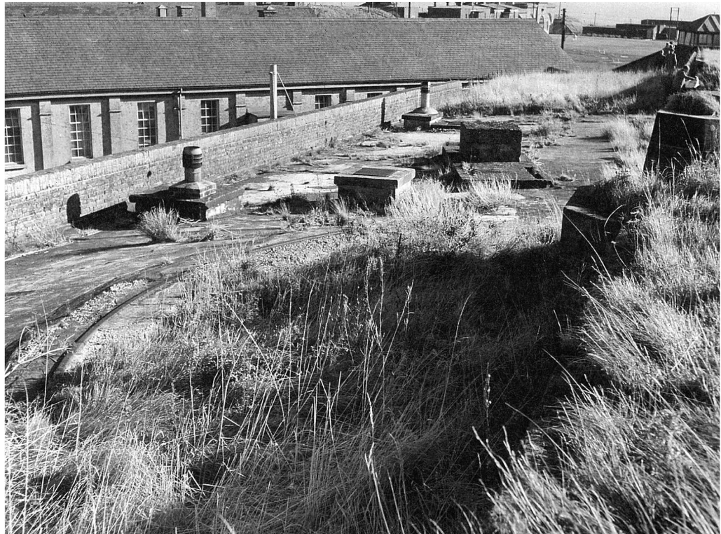
Figure 16 The terreplein of the West Face, in 1959, showing (at lower left) the racer from a late 19th-century traversing gun platform and (at top right) details of embrasures in the parapet. All of this detail is now lost or concealed (A5513/34 © Dover Museum)
