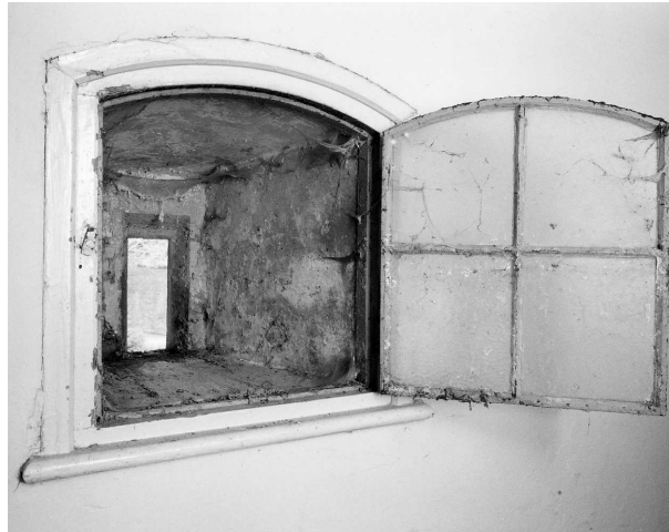
Figure 62 The Officers' Quarters; metal framed internal casement over a gun loop (NMR: AA043960 © Crown copyright 1998)
