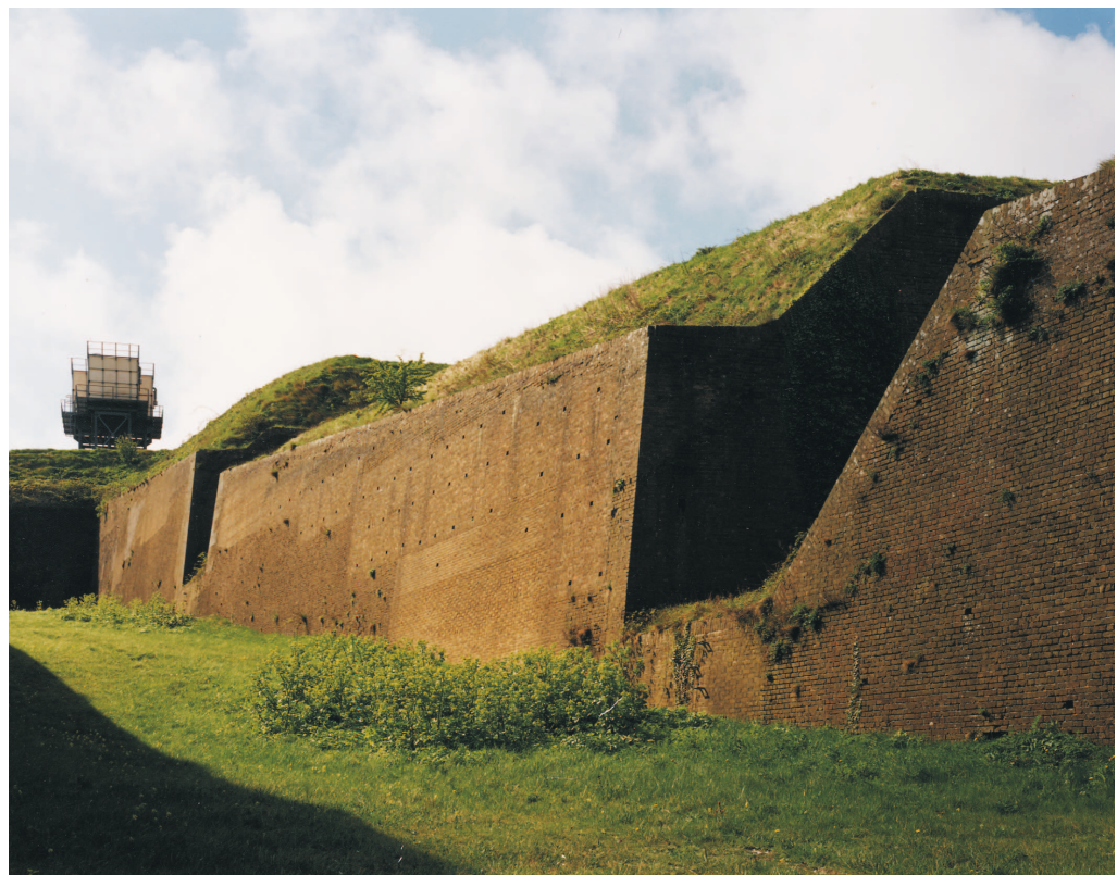
Figure 21 The eastern scarp revetment of the NW Bastion, showing the cross ditches and clear patching of the brickwork (NMR: BB03729 © Crown copyright 1998)
