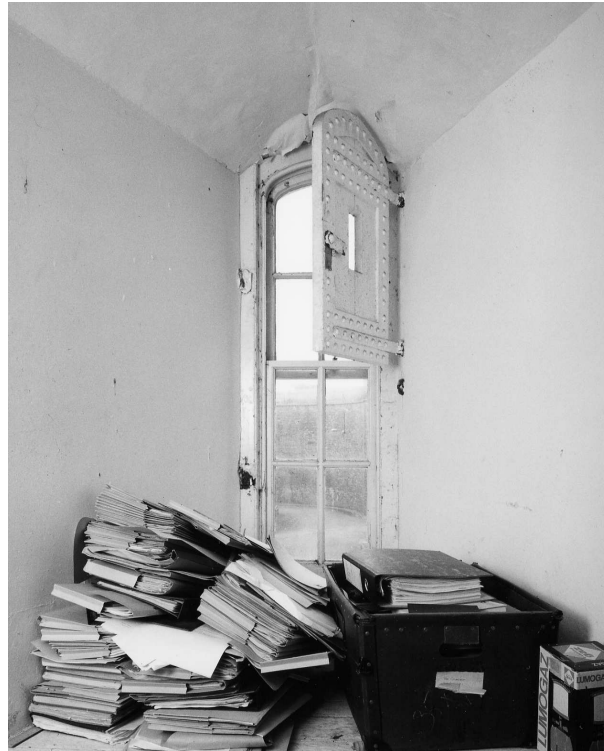
Figure 63 The Officers' Quarters; armoured shutter to a first-floor window on the west side of the north porch (NMR: AA043959 © Crown copyright 1998)
