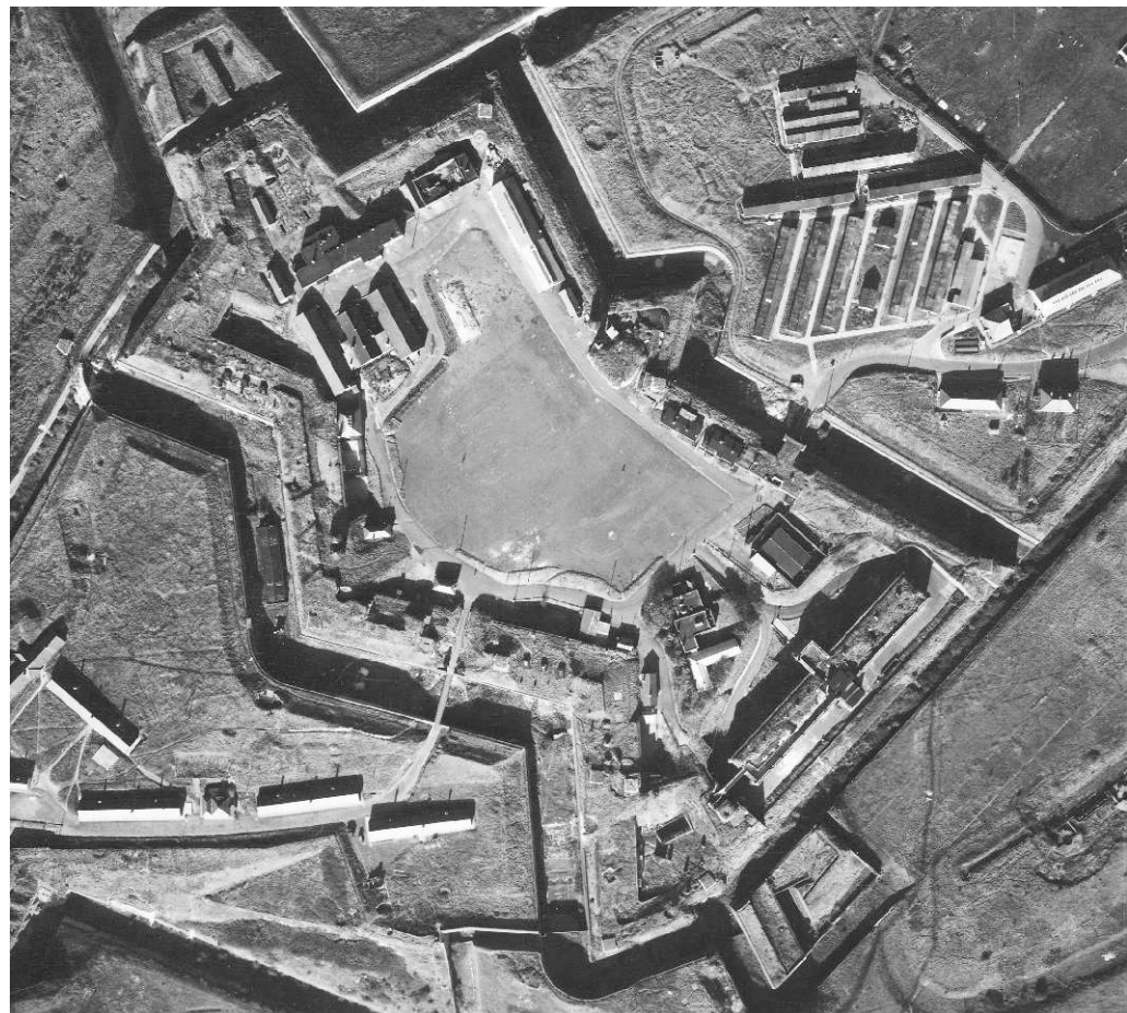
Figure 13 The Citadel from the air in 1945. Important additions include the hutment camp, built in 1939 (top right) (106G/UK944/6090-1 ©MOD)
