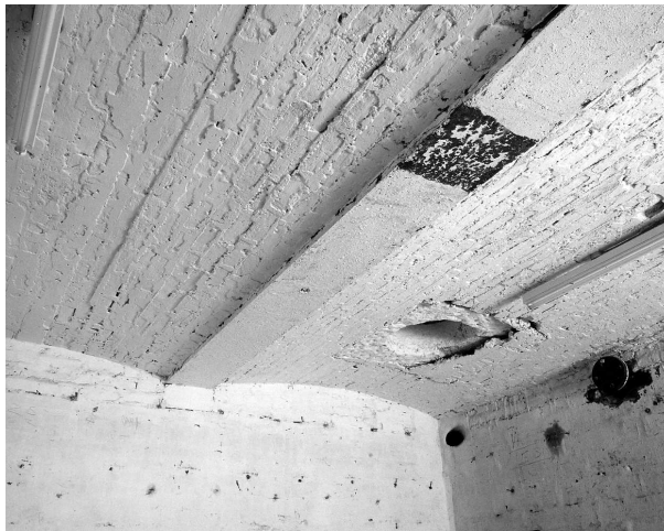
Figure 64 The Officers' Quarters; ceiling of one of the basement rooms, showing fireproof construction and circular inspection aperture (the room housed a water tank) (NMR: AA043963 © Crown copyright 1998)
