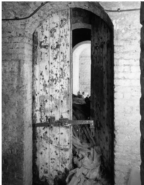
Figure 39 Gorge Casemates; detail of reinforced door, showing iron locking bar (NMR: AA043935 © Crown copyright 1998)
