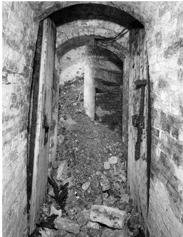
Figure 41 Inner NW Bastion; base of a newel stair shaft linking to a gallery leading to Centre and Outer NW Bastions (NMR: AA043964 © Crown copyright 1998)
