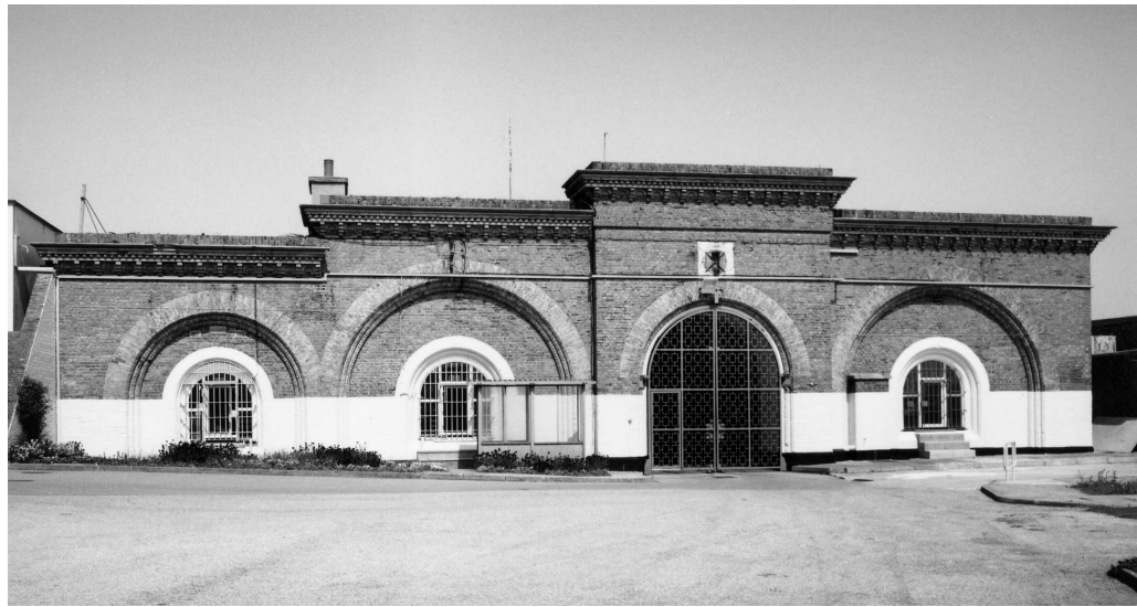
Figure 51 The Citadel; Main Entrance and Guard Room casemates, viewed from the Parade Ground (NMR: AA043941 © Crown copyright 1998)
