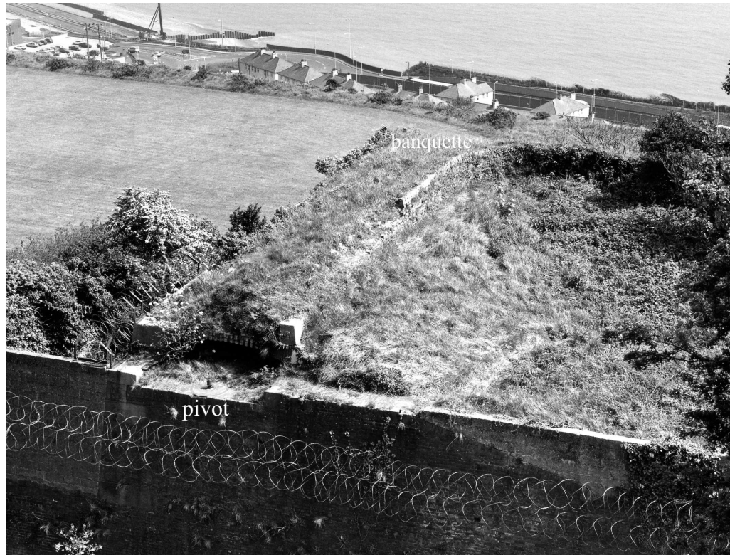
Figure 24 Part of the demi-bastion at the west end of the tenaille. Note the infantry banquette (centre) and pivot for a swing bridge (lower left) (NMR: BB043986 © Crown copyright 1998)
