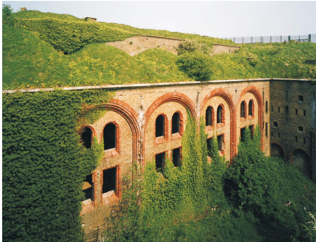
Figure 74 The South Flank Casemates of the Western Outwork, from the south. Above the capping course of the main elevation, earthworks protect a series of casemated gun positions, the front wall of which is just visible (NMR: BB032747 © Crown copyright 1998)
