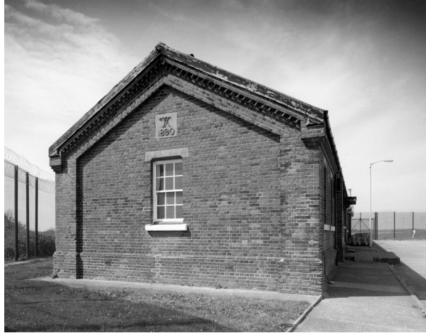
Figure 84 Barrack Hut No 1, in the Western Outworks, showing the royal cipher on the east gable (NMR: AA043992 © Crown copyright 1998)
