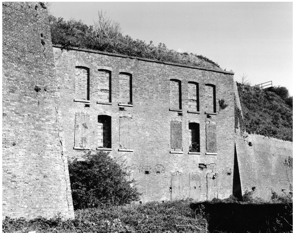
Figure 30 The Long Casemates; south elevation forming the scarp revetment of the inner South Ditch (NMR: 032741 © Crown copyright 1998)
