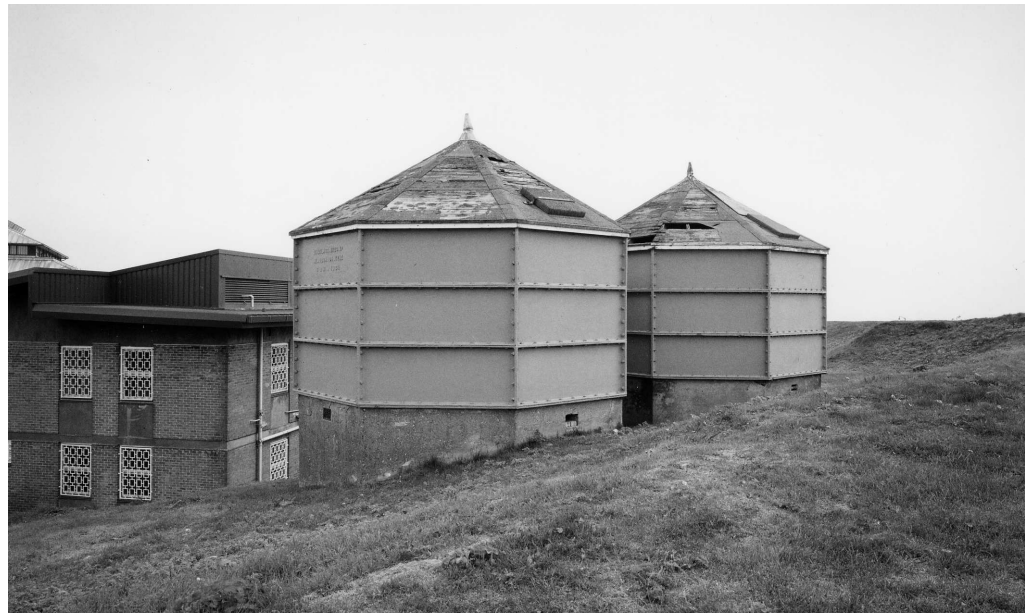
Figure 59 Twin water tanks set into the western rampart of the Citadel, erected in 1861 (nearest) and 1901 respectively (NMR: AA043942 © Crown copyright 1998)
