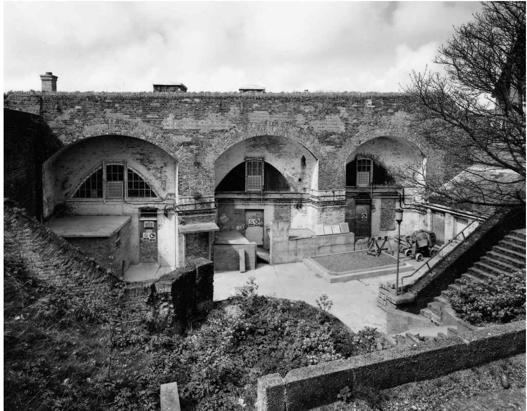
Figure 32 The rear elevation of the South-West Flank Casemates, from the south-east. Note the recessed façade of each casemate and the parabolic vaults. The sunken area incorporates an ablutions building with lean-to roof (right) (NMR: BB032719 © Crown copyright 1998)
