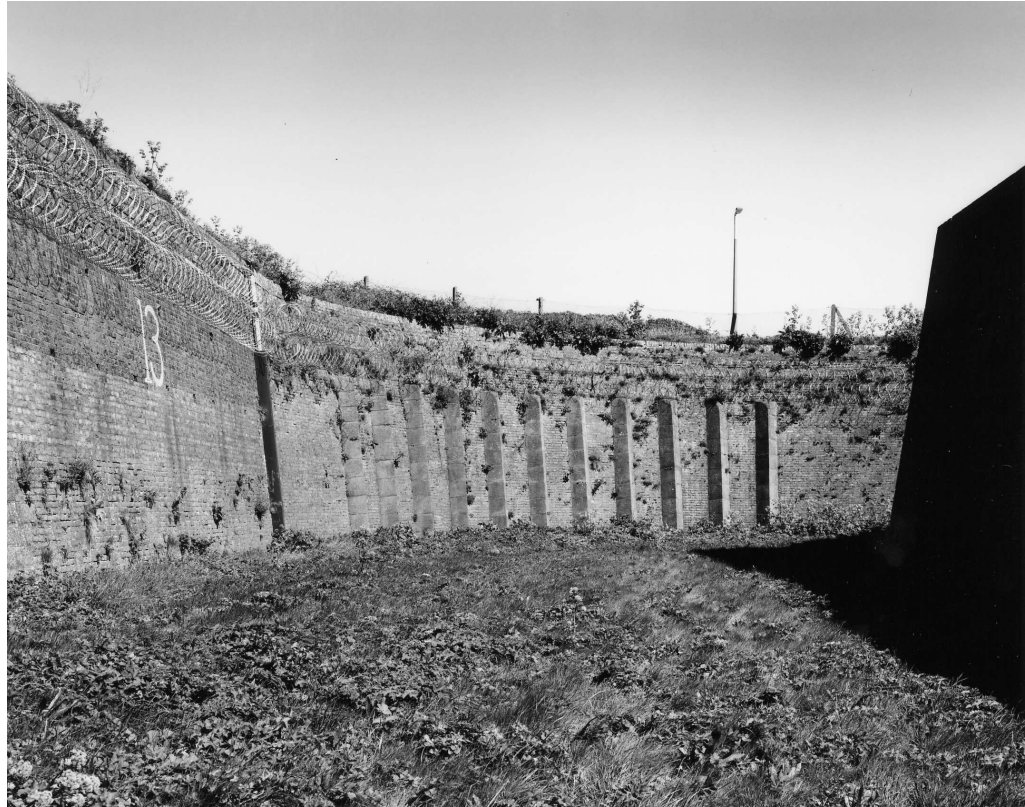
Figure 22 Anti-ricochet pilasters against the counterscarp of the Gorge Ditch, from the west (NMR: BB032731 © Crown copyright 1998)
