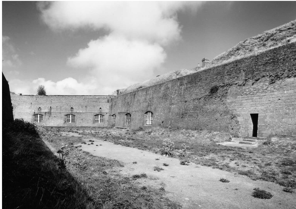
Figure 19 The West Ditch, looking north, showing the West Postern (at right) and the windows of the casemates of the West Face and West Flank (NMR: BB032743 © Crown copyright 1998)
