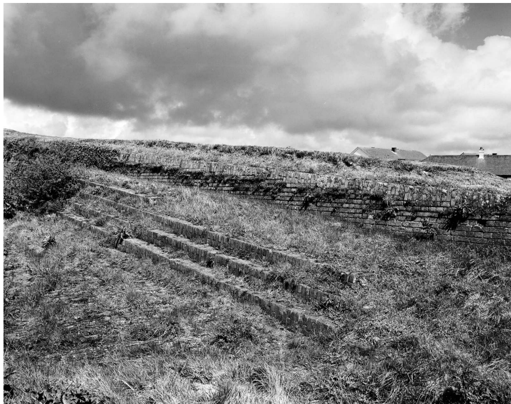
Figure 17 Overgrown infantry banquette and steps on the East Face, or south end of the gorge rampart (NMR: BB032736 © Crown copyright 1998)
