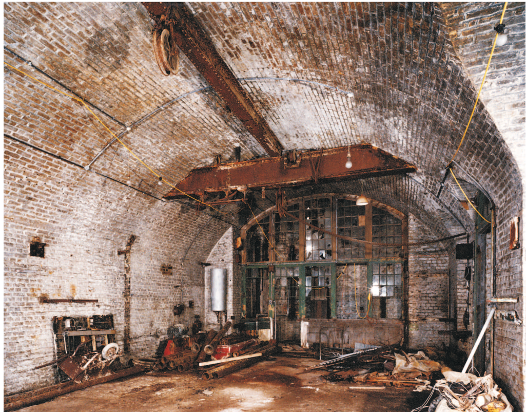
Figure 57 The Engine Room, showing the lifting beam and light well partition (NMR: AA044020 © Crown copyright 1998)
