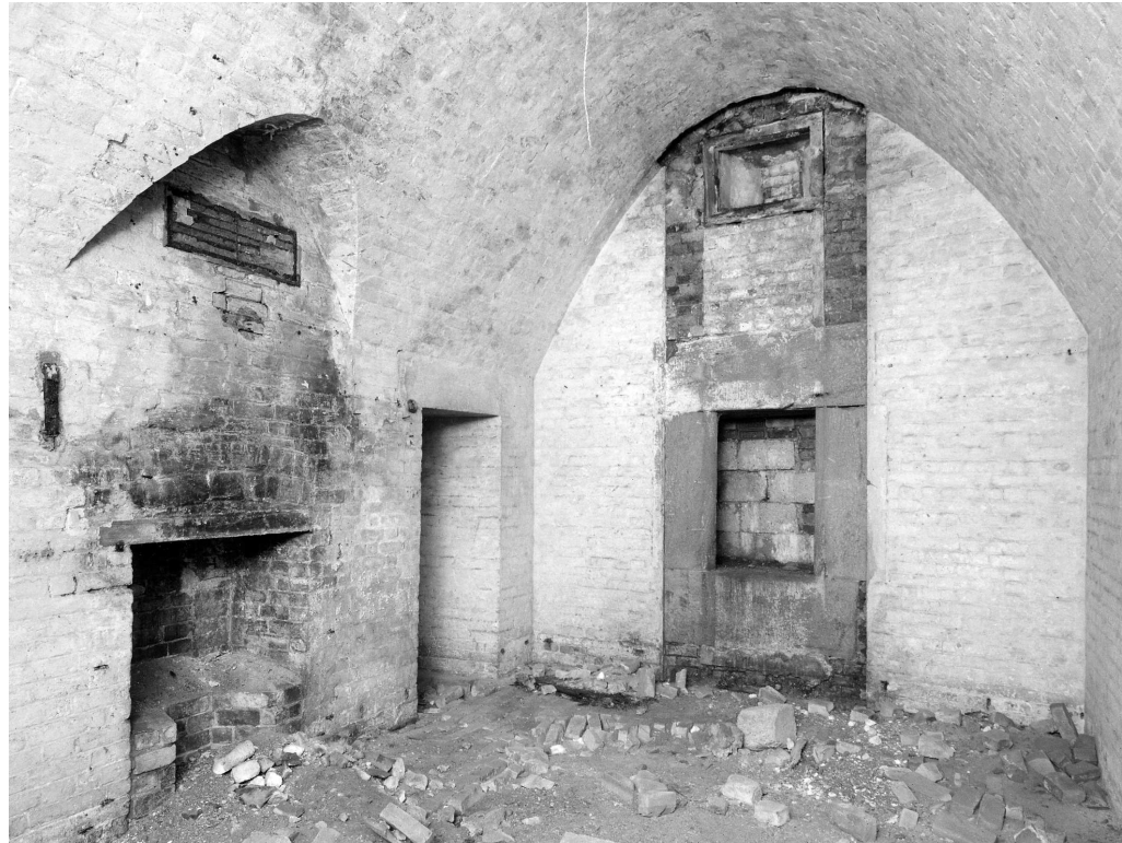
Figure 37 The Gorge Casemates; southern group, central casemate of the outer set, showing the blocked carronade embrasure and scar from the vertical sliding shutter in the ditch wall (at right), entrance (just left of centre) and fireplace (at left) (NMR: AA044007 © Crown copyright 1998)
