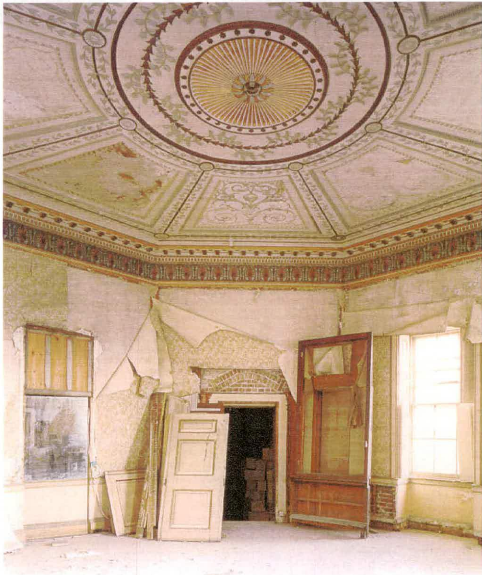
Figure 14, the saloon in 1995, prior to English Heritage's acquisition of the building. The wallpaper applied to the ceiling has either been removed or fallen away. Photograph: Paul Dixon for English Heritage.
