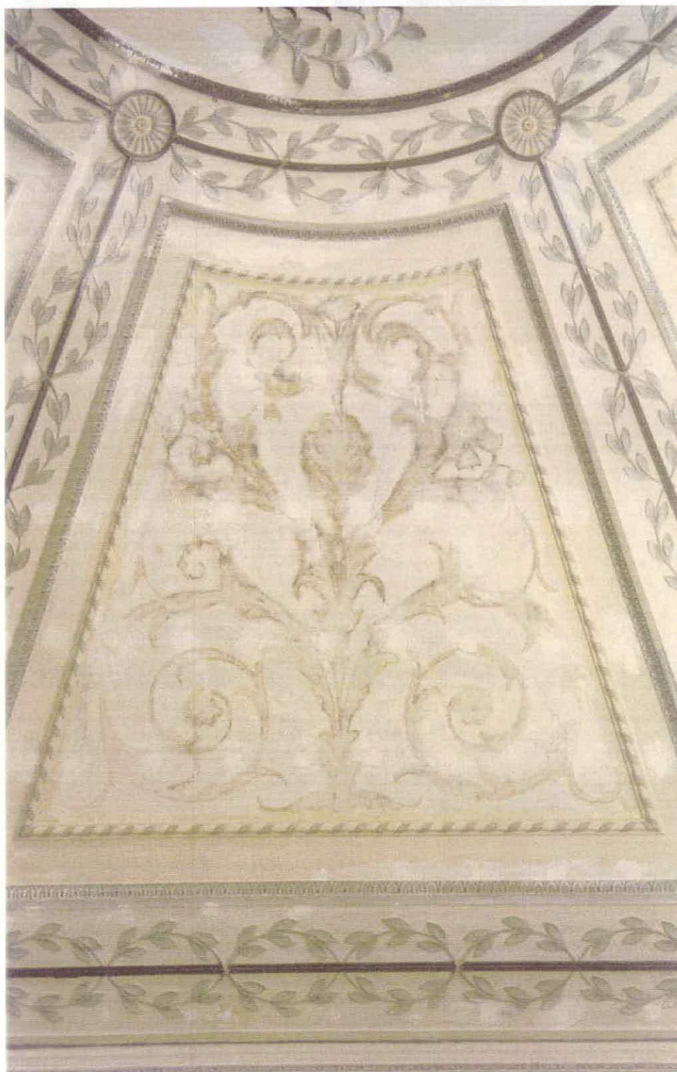
Figure 17, the ceiling panel above the door to the dining room, photographed in 1997 after the wallpaper had been removed and the plaster surface prepared for repainting. The decoration is pattern type B. Photograph: English Heritage, Historical Analysis and Research Team.
