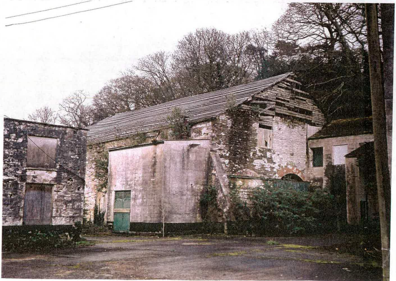
Fig. 28 Warehouse c.1865, (top) and Dry Sand Shop, in 2002.
