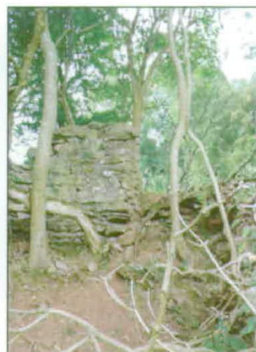
Fig. 6. Adcombe Chapel: the NW buttress
