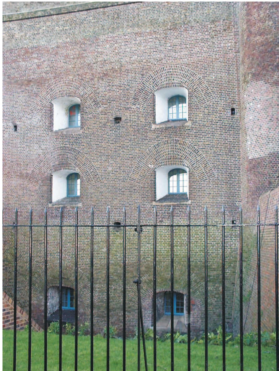
Figure 11 Artillery embrasures in the west elevation of Clarence Tower, at first floor, ground floor (centre) and basement levels, in December 2002 (author)
