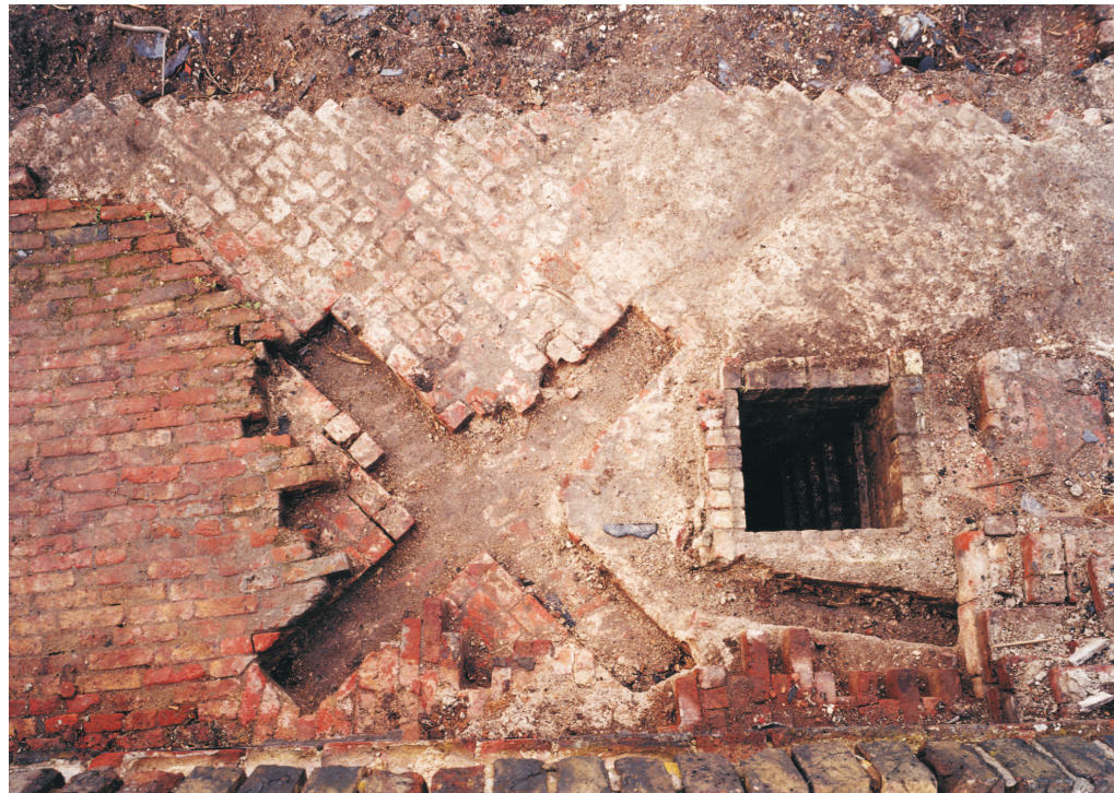
Figure 29 Clarence Tower; the eastern area of the roof, showing the cross-like rebate for the holdfast of gun no III, and the adjacent shaft to one of the roof cisterns (© NMR: AA021138)
