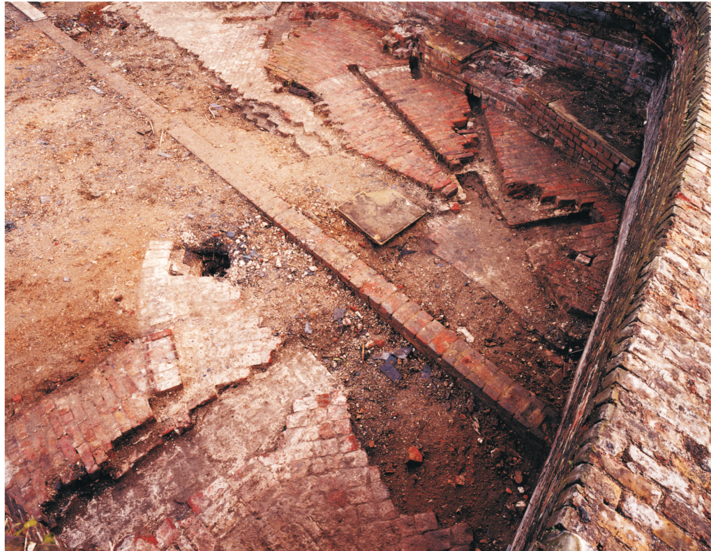
Figure 28 Clarence Tower; the south-eastern area of the roof, showing the position of gun no II, cut by a trench for the insertion of a 20th-century dwarf wall. The flagstone (at centre) covers the ventilator from the casemates below; to its right is the rebate for the holdfast and two radiating rebates for timbers which anchored the gun racers (© NMR: AA021137)
