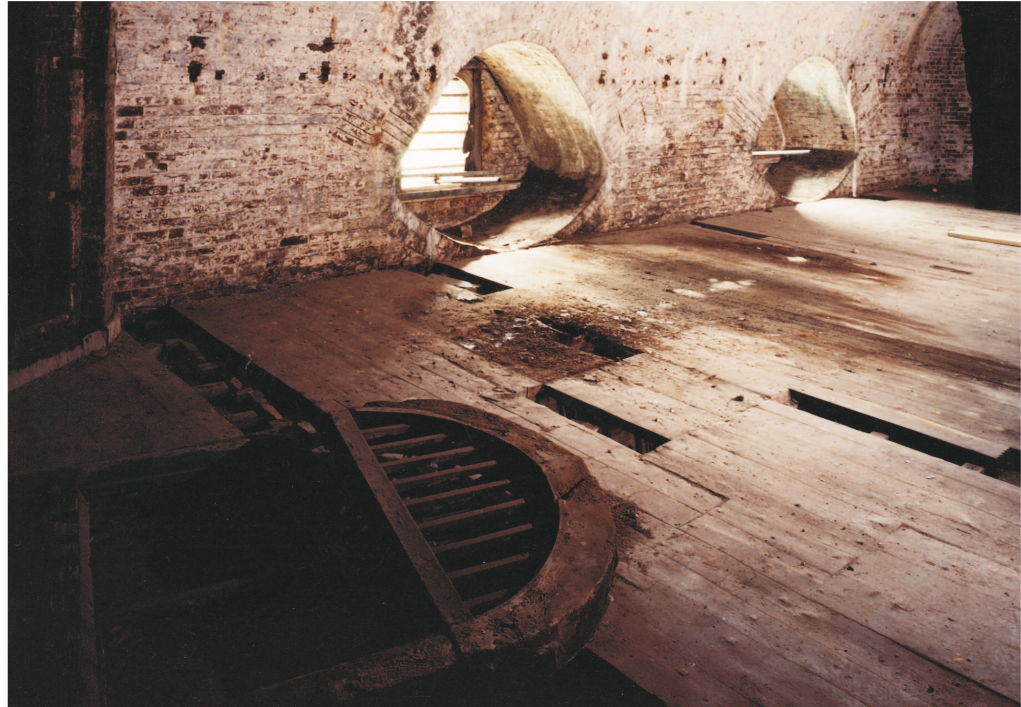
Figure 23 Clarence Tower; the first floor east casemate, showing the boards, window frame removed from the north elevation, and the ocular artillery embrasures in the east wall (© NMR: AA020009)
