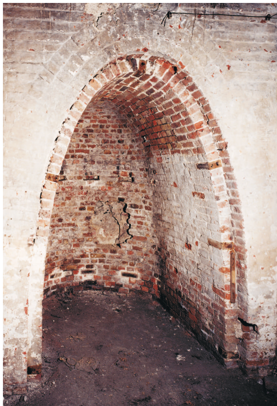
Figure 43 The West Casemates, ground floor; expense magazine in the east wall (© NMR: AA020018)
