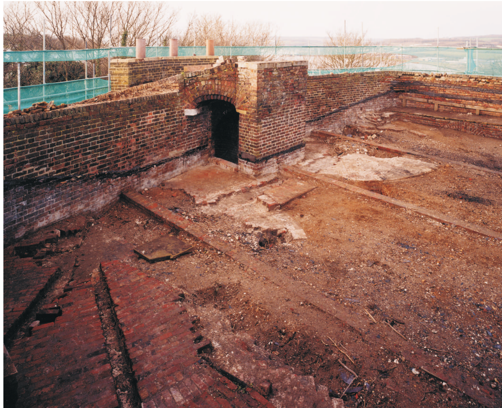
Figure 26 The southern end of the roof level on Clarence Tower, showing the porch to the ammunition shaft and the fragmentary original brick gun floor. Note also the three intrusive dwarf walls, built to support a temporary roof structure (© NMR: AA020032)
