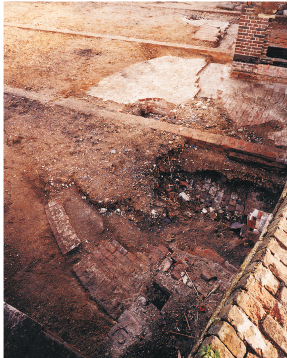
Figure 27 Clarence Tower; the south-western corner of the roof level, showing the emerging semi-circle of gun position no I, badly damaged by a broad trench cut for the insertion of a 20th-century dwarf wall for a later roof (© NMR: AA021135)
