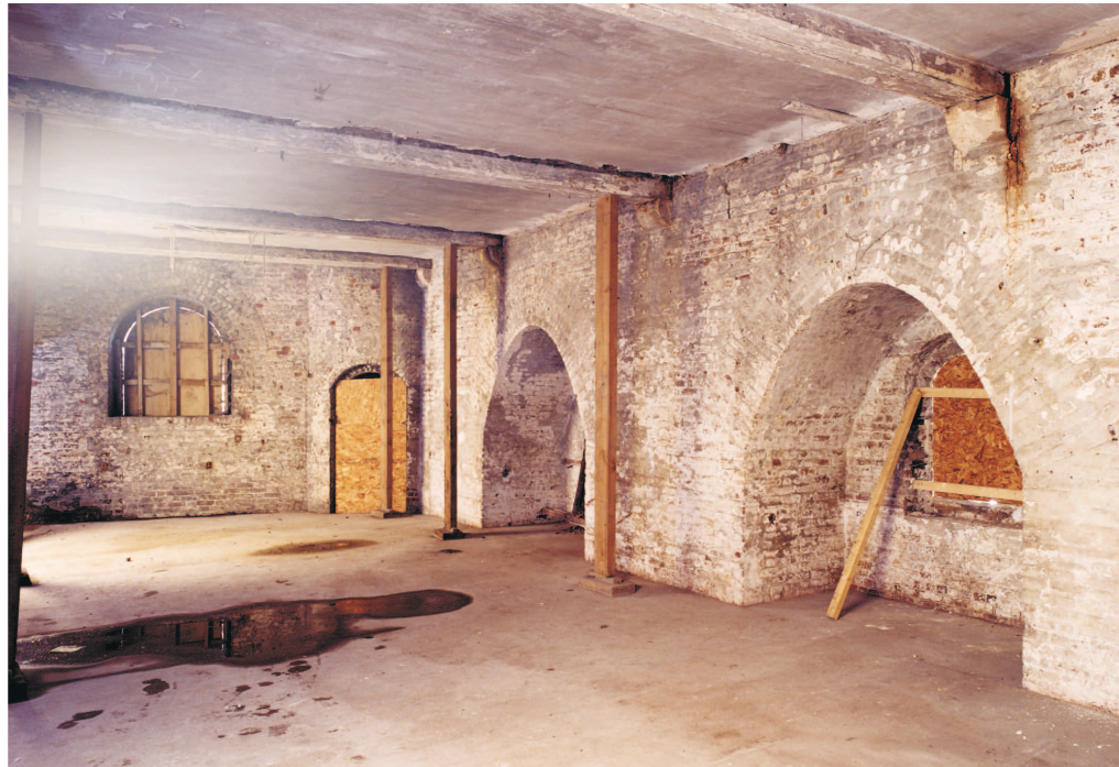
Figure 20 The interior of Clarence Tower, east casemate, showing the ground floor with original ceiling, artillery recesses (right) and window in north elevation (left) (© NMR: AA020013)
