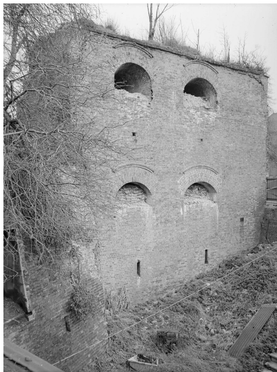
Figure 46 The Maidstone Road Guard House, south-west face of the salient, in 1961. The formidable nature of the gun complement facing along the Maidstone Road, only half of which is shown in this photograph, is immediately apparent (© Crown copyright NMR: AA61/2536)
