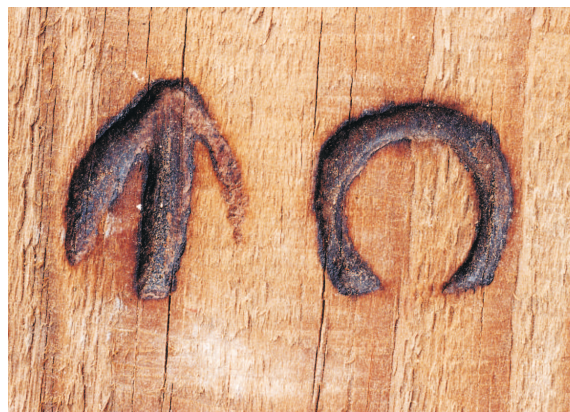
Figure 24 The Board of Ordnance symbol, as branded onto one of the first floor timbers in Clarence Tower. The symbols are each 3.5cms tall (© NMR: AA031469)
