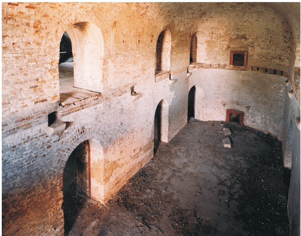
Figure 18 Clarence Tower, west casemate ground and first floor levels, looking south from the north-west turret. Shows the spine wall and the apsidal south wall with fireplaces on both levels (© NMR:AA021140)
