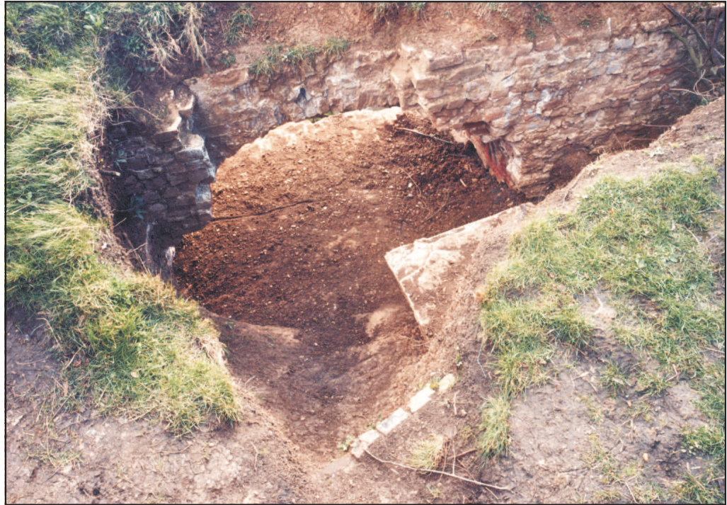
Figure 27 The rear face of a counterfort with a surviving stone of the gun floor in the west bastion (NMR: AA031332)
