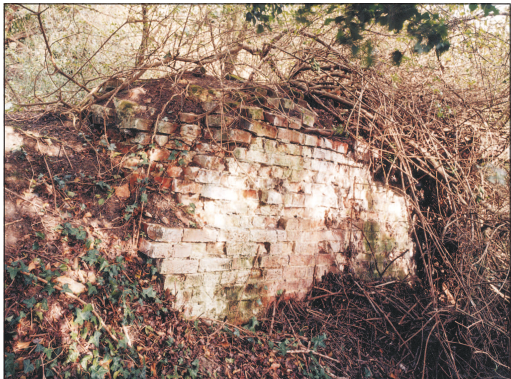
Figure 28 A section of the rear revetment wall of the lower gun line (NMR: AA031334)
