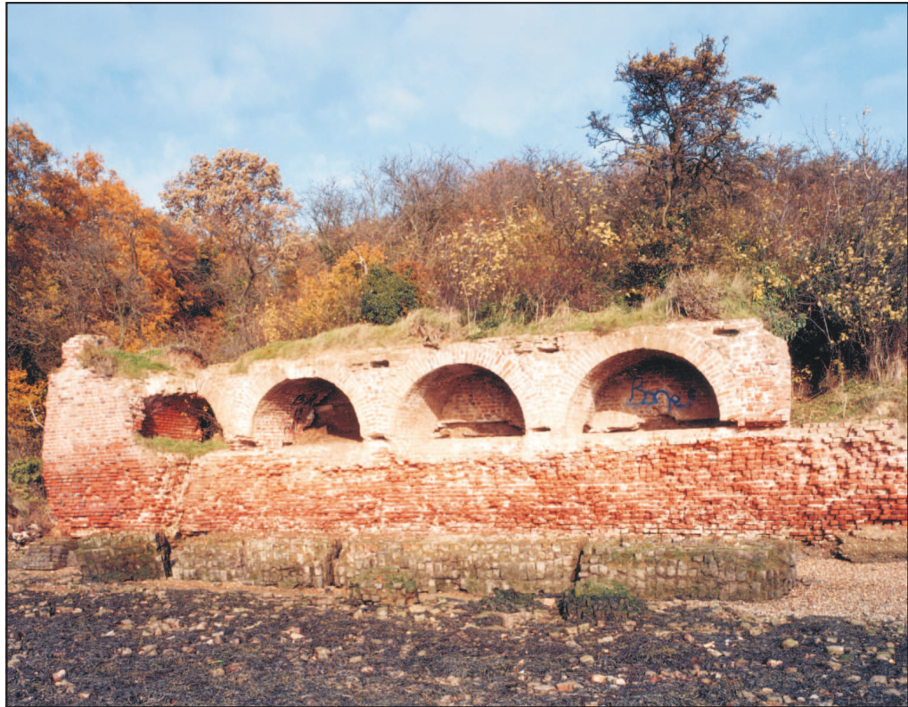
Figure 26 The counterforts of the west bastion (NMR: AA031340)
