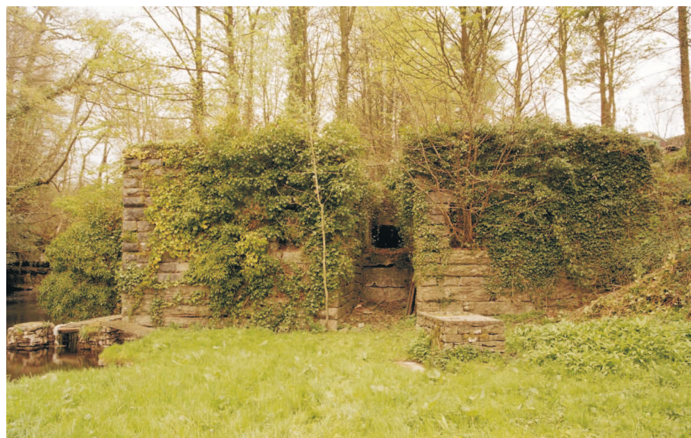
Figure 17. Middle incorporating mill group from the south (NMR: AA038844)
