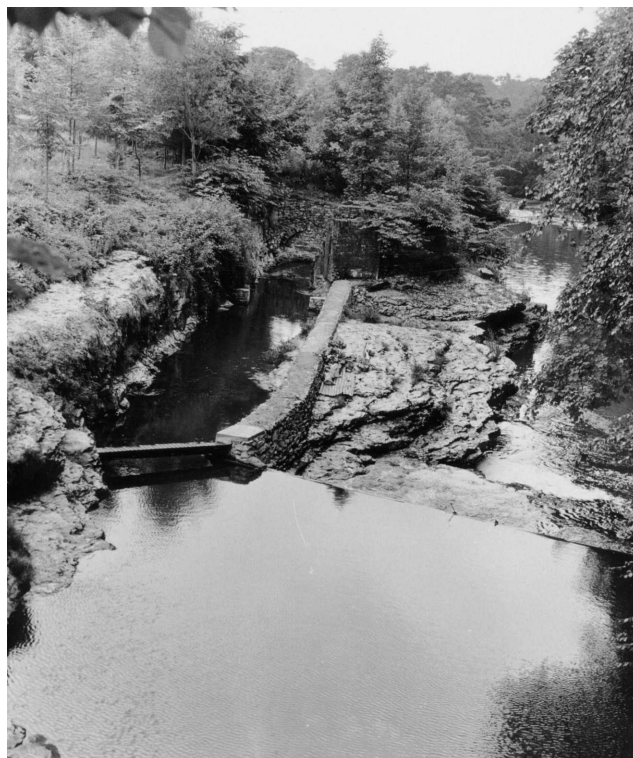
Figure 8. Basingill from Force Bridge looking south, probably taken in the 1960s (reproduced by permission of John Foster)
