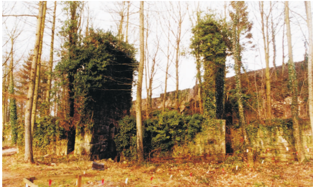
Figure 21. Southern incorporating mill group with blast walls in situ (reproduced by permission of Oxford Archaeology North)
