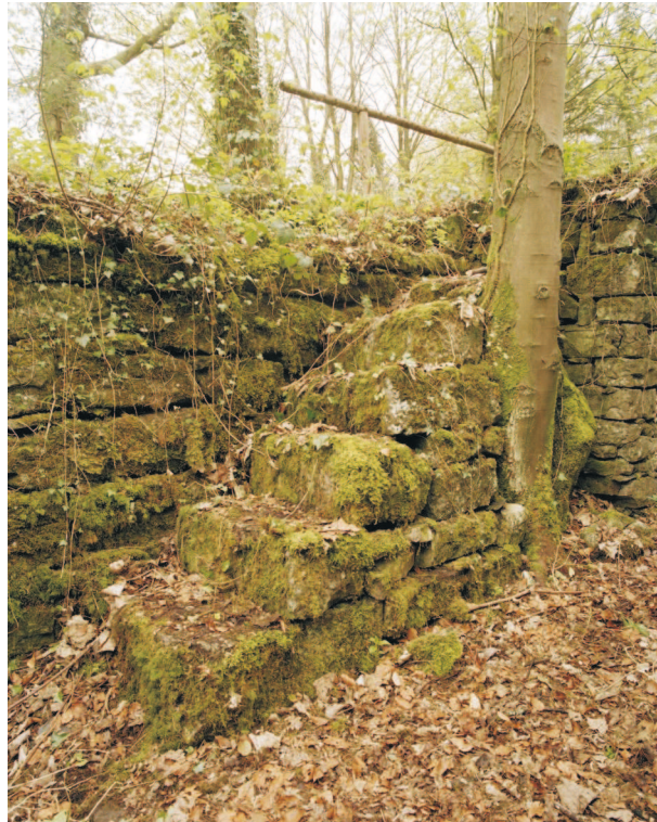
Figure 15. Flight of steps in mill 2 (NMR: AA038833)
