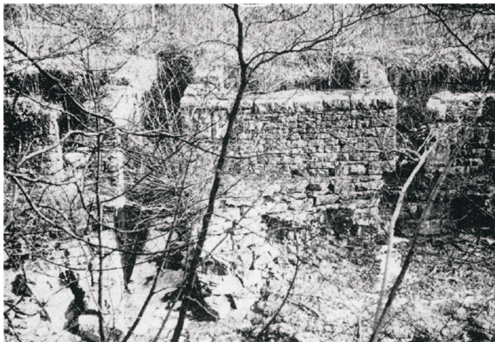
Figure 9. Northern incorporating mill group from the west bank of the River Kent, 1962 (reproduced by permission of The Newcomen Society)
