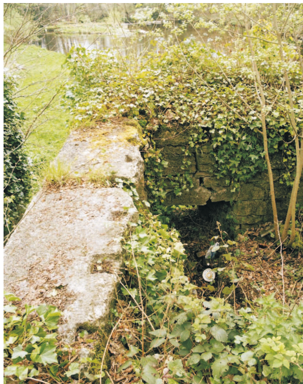
Figure 18. Floor-joist sockets In mill 4 (NMR: AA038842)
