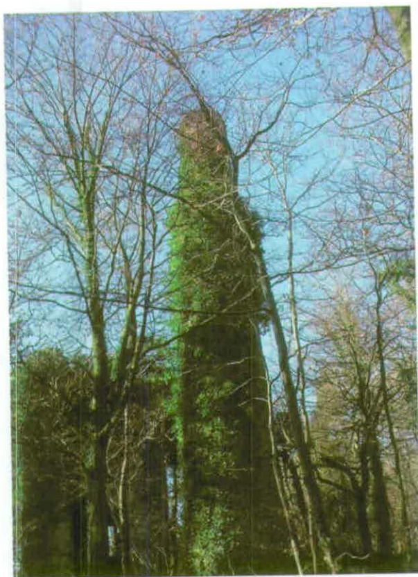
Plate 3 (left). The chimney stack.
