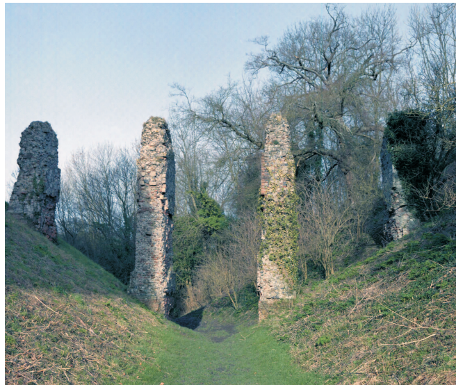
Figure 19 The brick-and-flint piers of the late 15 th /early 16 th -century bridge which provided direct access from the Inner Ward to the northern part of the bailey (NMR: AA028419)
