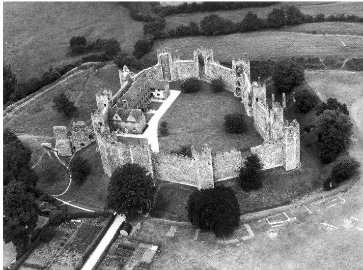
Figure 15 An aerial photograph of Framlingham Castle clearly illustrating the relationship between the curtain and the surrounding earthworks (EH Historic Plans Collection A397/9)
