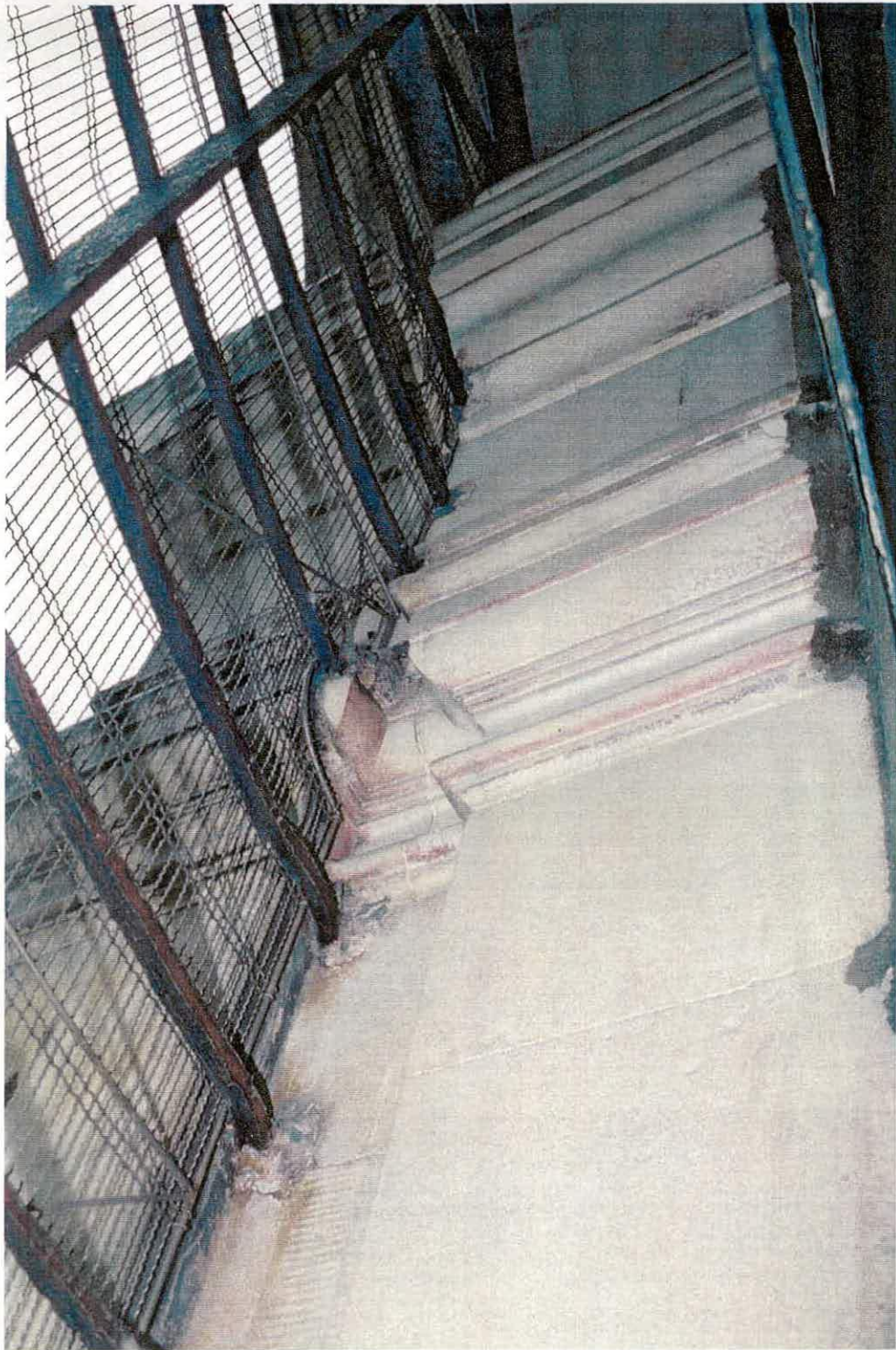
Fig. 15, the south jamb of the east window, showing how the original ferramenta is set in sockets cut into the masonry just behind the outer column, June 2002.
