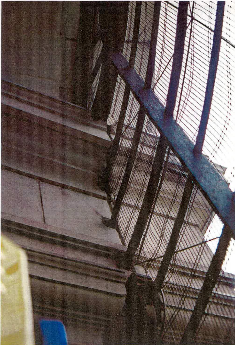
Fig. 21, a detail of the east window showing the mouldings of the cornice and capitals cut by a narrow rebate for the original glazing.
