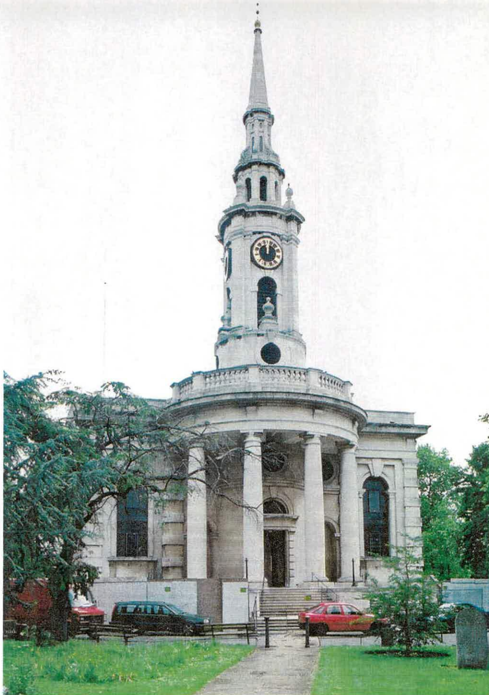
Fig. 8, St Paul, Deptford, the west front viewed from the west, June 2002.
