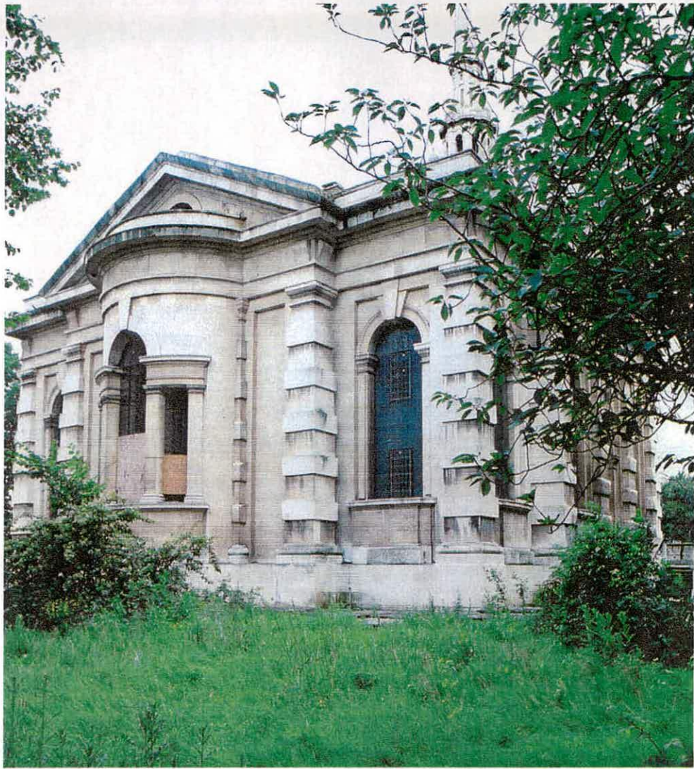
Fig. 10, St Paul, Deptford, the east front viewed from the north-east, June 2002.
