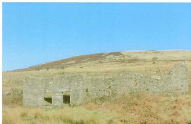
Plate 4:9. Golden Dagger mine. Dinah's House from the west.
