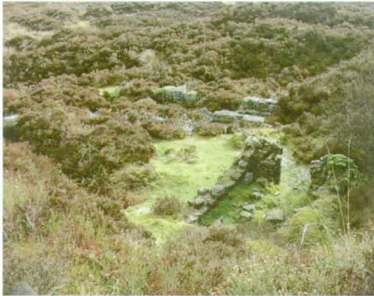
Plate 4:7. Birch Tor and Vitifer mine. The turbine house and wheelpit PW3.
