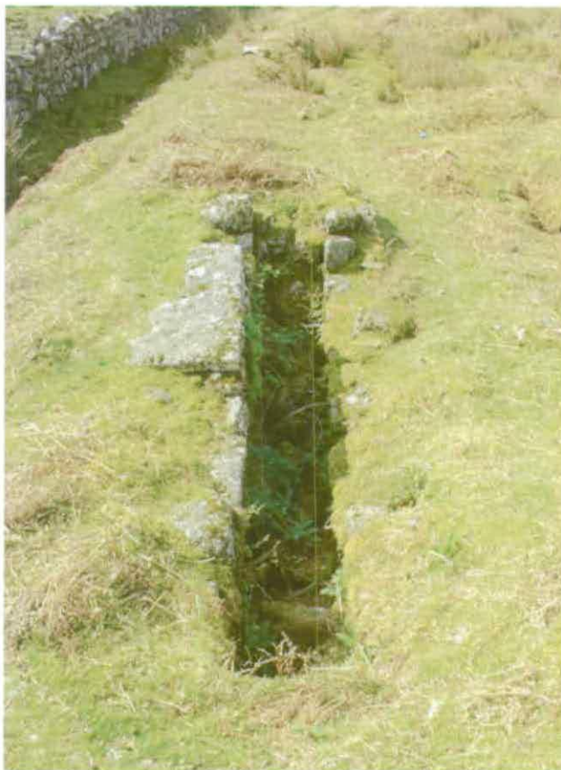
Plate 4:11. East Birch Tor mine. Stamping mill wheelpit at dressing floor DF9.
