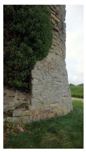
Fig 26: The robbing of the ashlar ends abruptly on the north tower because this was where the moat as it existed in the 19th century prevented access to the walls (Investigator Photograph)
