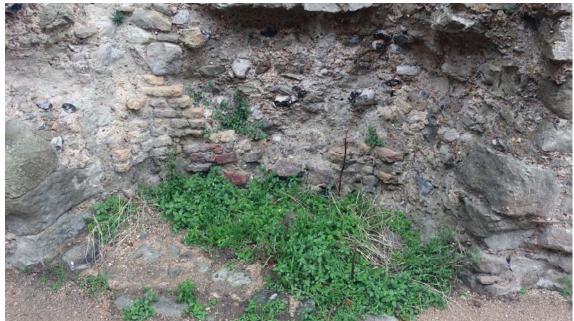
Fig 25: The north turret of the gatehouse also has bricks in its fireplace, though most of these have a distinctly reset quality (Investigator Photograph)
