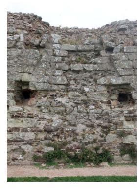
Fig 18: One of the fireplaces in the north wall of the medieval castle shows the typical arrangement of flanking holes where corbels were located (Investigator Photograph)
