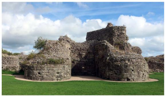
Fig 21: The keep from the west, showing the intact ashlar on much of its ground floor and the absence of any openings (Investigator Photograph)
