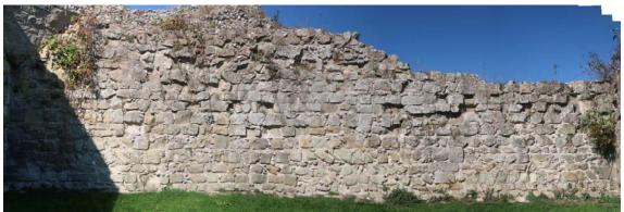
Fig 9: This panorama of multiple photographs shows the patching and perhaps a triangular shape in the west wall of the interior of the keep (Investigator Photograph)
