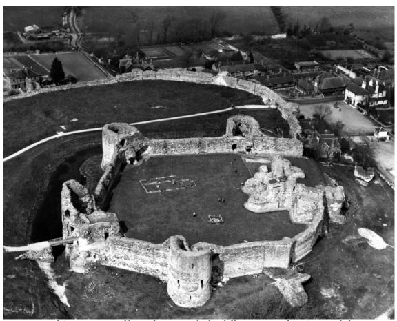
Fig 11: In this 1948 Aerofilms photograph the fallen Roman bastion and the replaced postern gate can be seen at the bottom of the image, to the east (right) of the 13th-century tower in the south wall EAW014356 ©Historic England Archive
