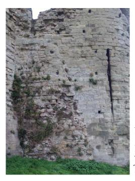
Fig 14: The fragment on the north side of the gatehouse looks confusingly both earlier, yet well integrated into, the fabric of the structure (Investigator Photograph)
