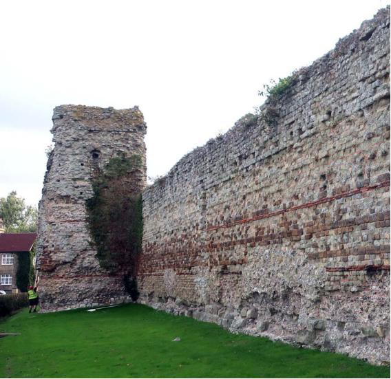
Fig 6: Bastion 3 of the Roman fortification is at the northern end of what was once thought to have been the line of the Norman palisade. It is possible that its raised storey may have housed a light to aid navigation (Investigator Photograph)
