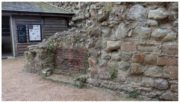
Fig 24: In the south turret of the gatehouse, the eastern room on the ground floor has bricks in the rear of its fireplace (Investigator Photograph)
