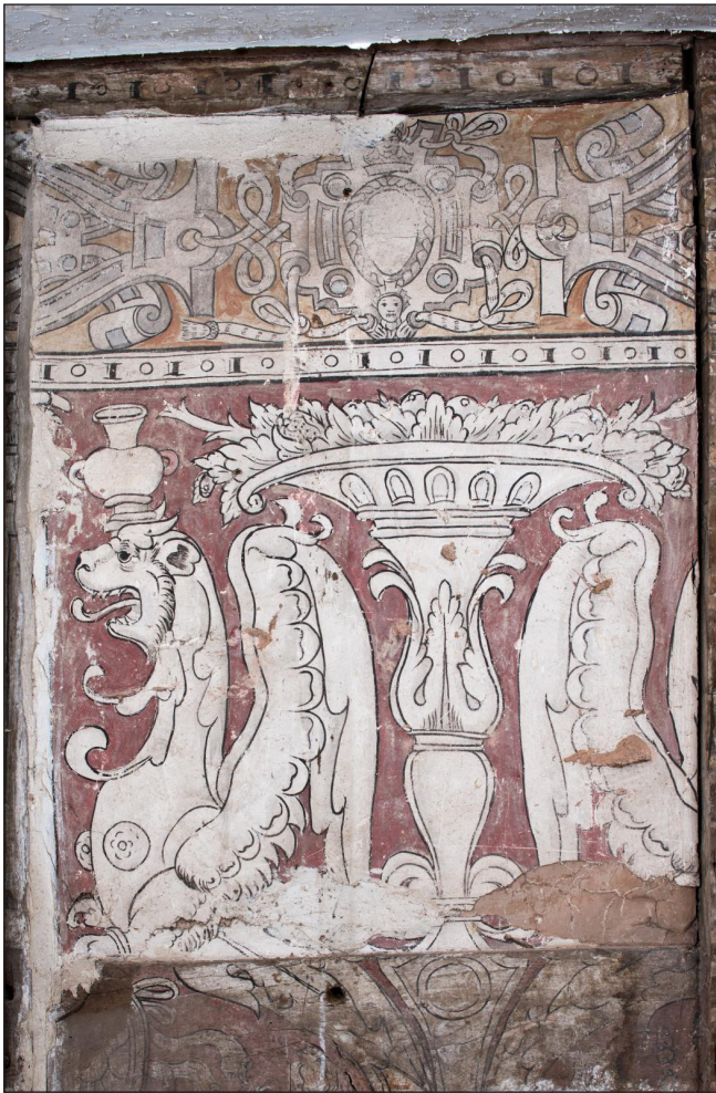
Figure 14 Detail of east elevation, northernmost surviving panel (DP221688)
