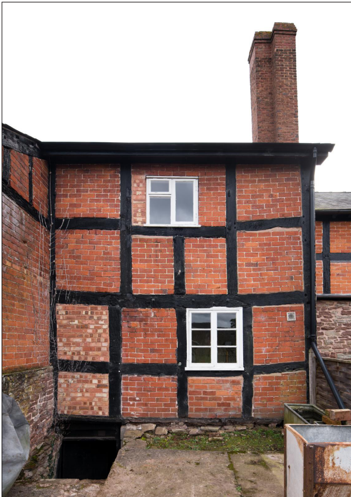
Figure 3 North elevation of cross wing (DP221702)
