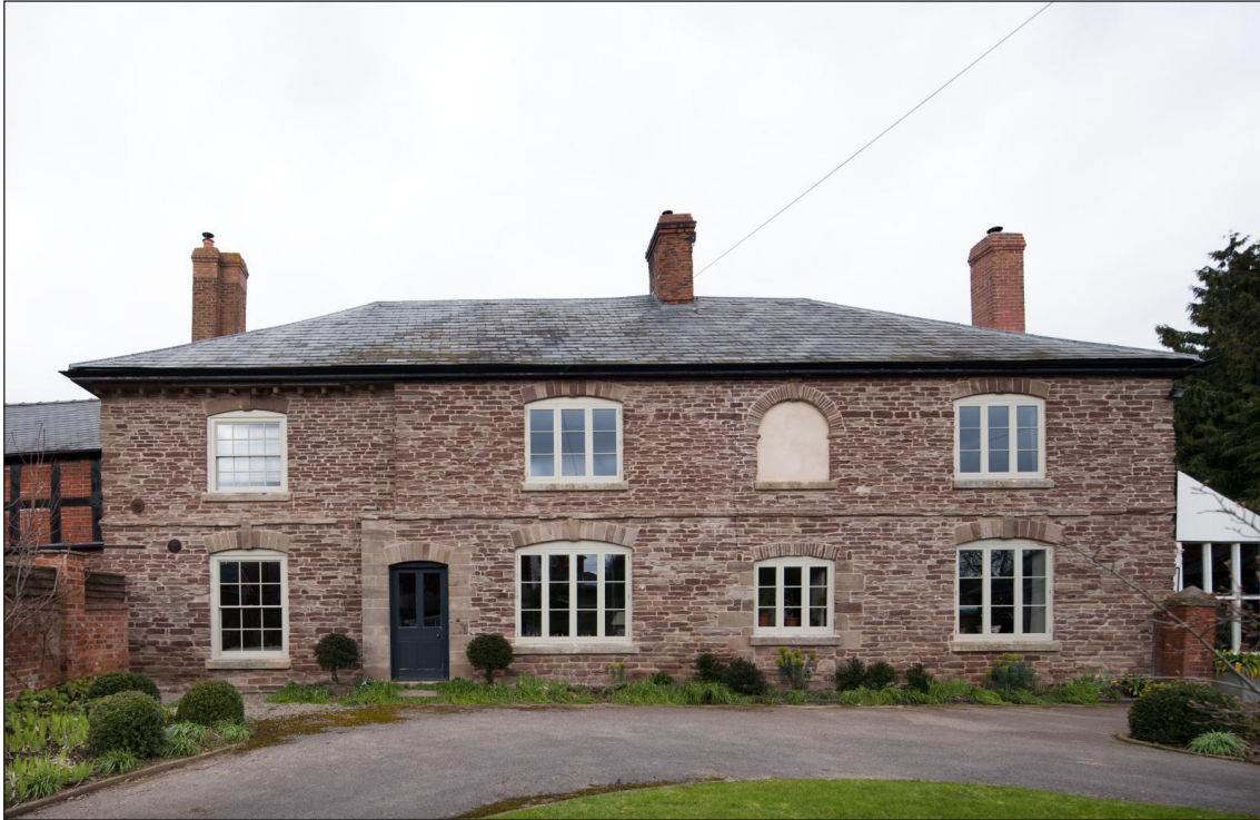
Figure 1 South elevation of Church House Farm (DP221705)
