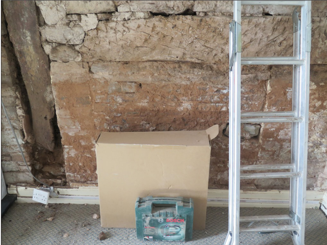
Figure 8 Inserted fireplace in the west elevation of the cross wing, with later blocking. Photo Stuart Mee
