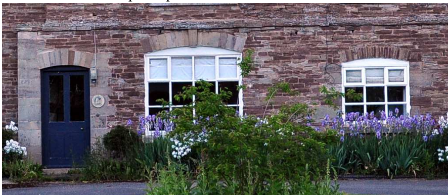
Fig.9. The south elevation showing the blocked doorway on the right and the later new position for the principal doorway on the left.
