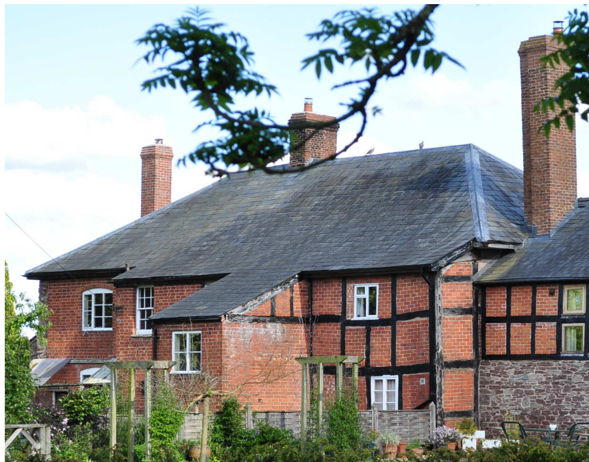
Fig.5. The rear elevation of Church House Farm seen from the north-west.
