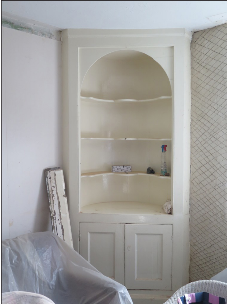
Figure 23 Fitted corner cupboard in ground-floor room of cross wing. Photo Stuart Mee
