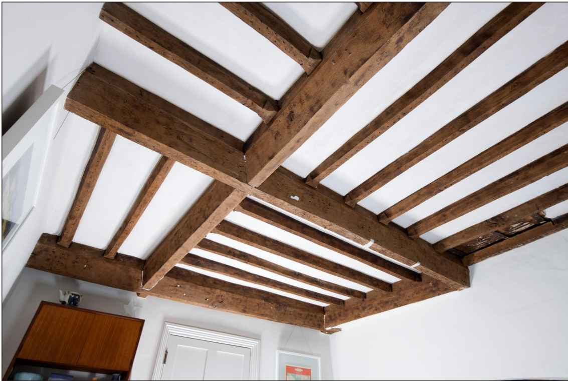
Figure 19 Counter change ceiling inserted into the original hall, and retained in subsequent rebuildings of the range (DP221699)
