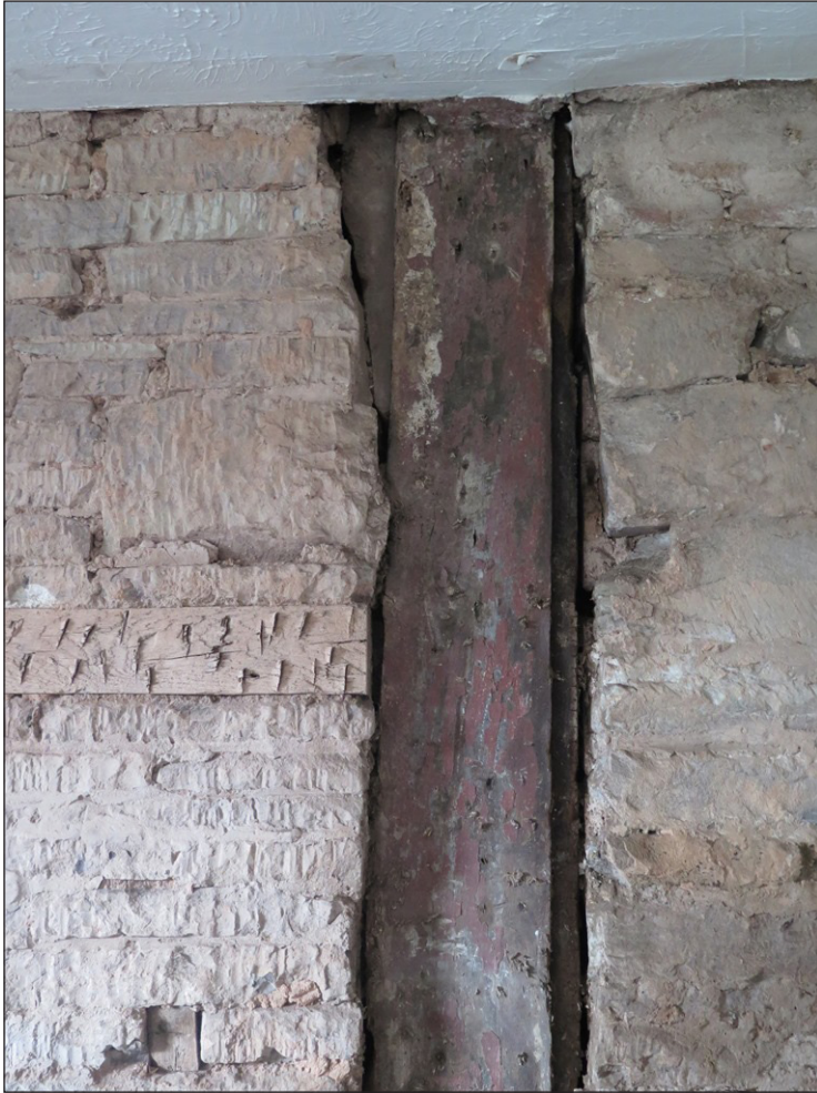
Figure 16 Detail of stud in west elevation of cross wing showing surviving fragments of dark red paint. Photo Stuart Mee
