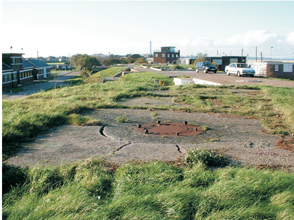
Figure 14 The 12-pdr QF gun platform, with the holdfast of the eastern gun in the foreground (NMR: AA008680)
