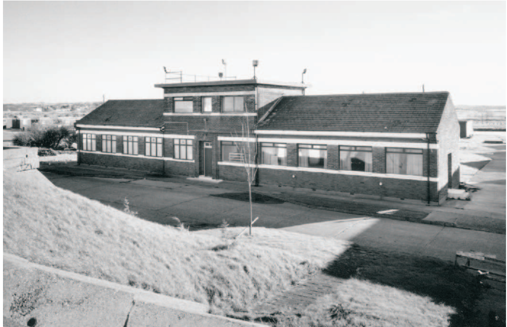
Figure 27 The naval offices, from the north (NMR: AA008694)
