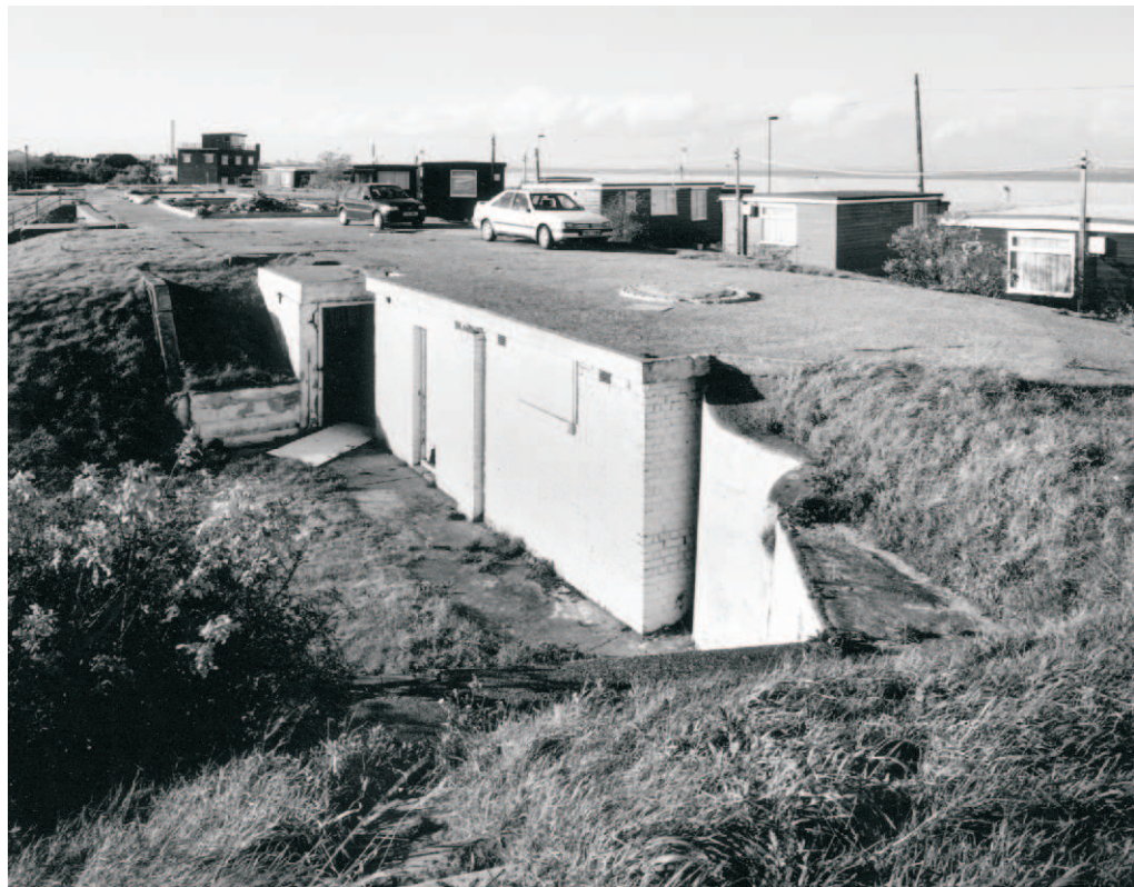
Figure 24 A naval building inserted to the rear of the old no II 6-inch gun pit, from the south-east (NMR: AA020005)
