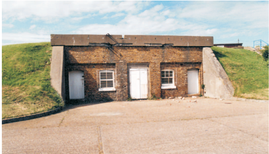
Figure 11 The entrance façade of the 9.2-inch magazine, showing the central entrance and identical storage rooms on each side
