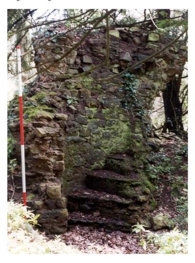
Fig 8: Remains of a newel staircase (n on Fig 5)
