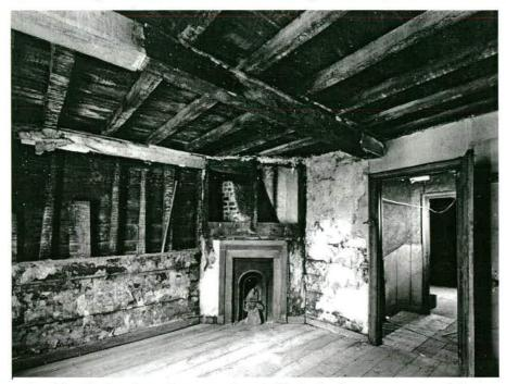
Fig. 30 – Timber-framed construction visible in the front room, second floor, No. 76 Bermondsey Street (English Heritage, BB000118).
