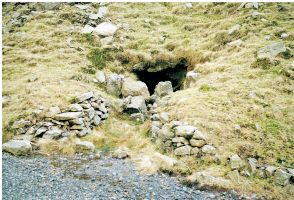
Figure 20. View of the entrance to Pave York Bottom Level from the north
