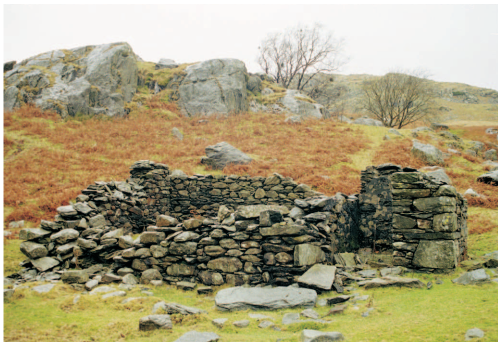
Figure 43. View of the dry store from the south
