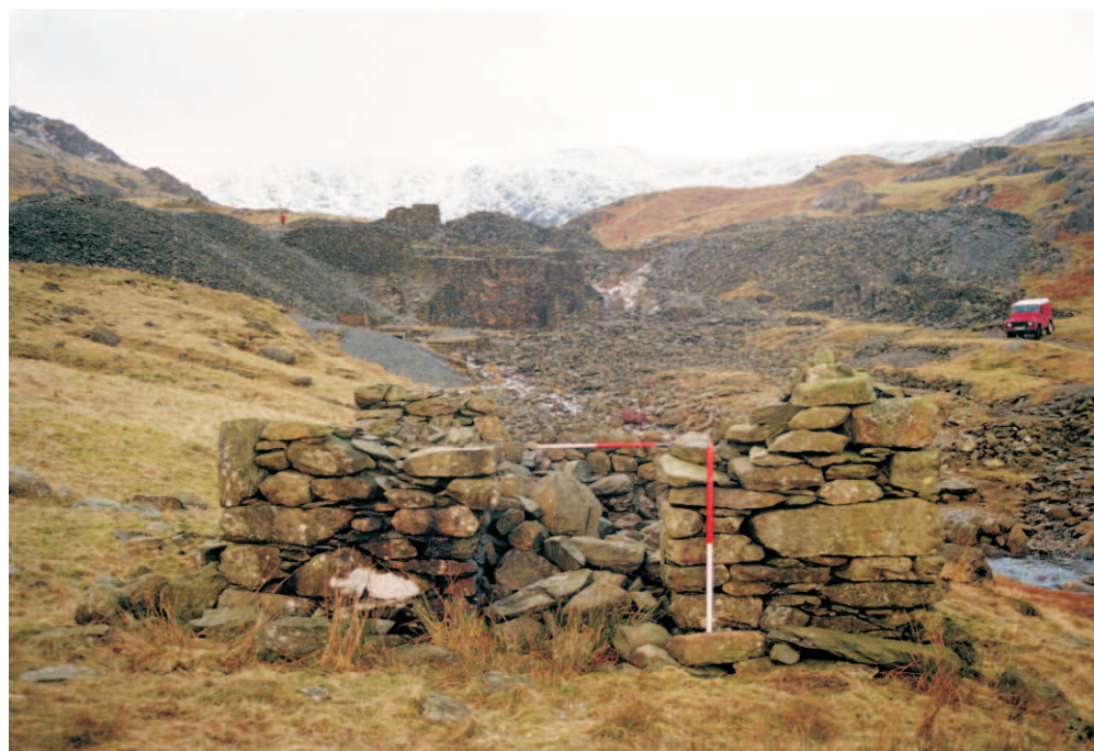
Figure 44. View of the explosives store from the east
