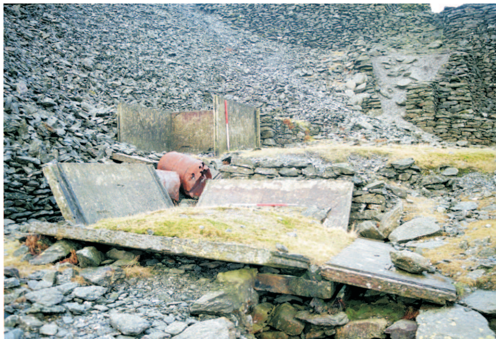
Figure 41. View of the precipitation tanks from the north-east
