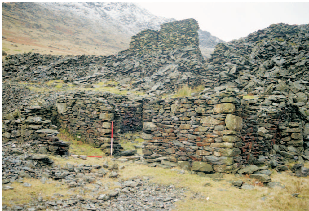
Figure 36. View of Building 7 from the north-east
