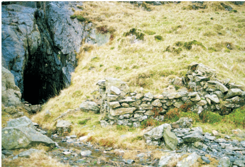
Figure 15 a. View of the entrance to Long Crag Level from the north-east
