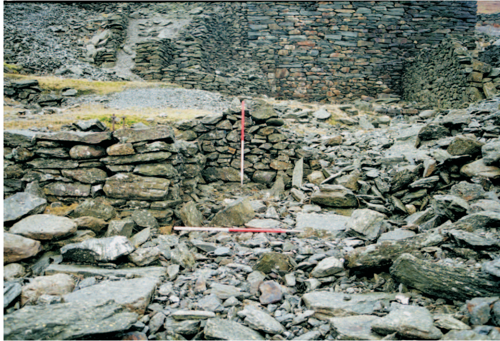
Figure 30. View of the wheel-pit of Water Wheel 5 from the east
