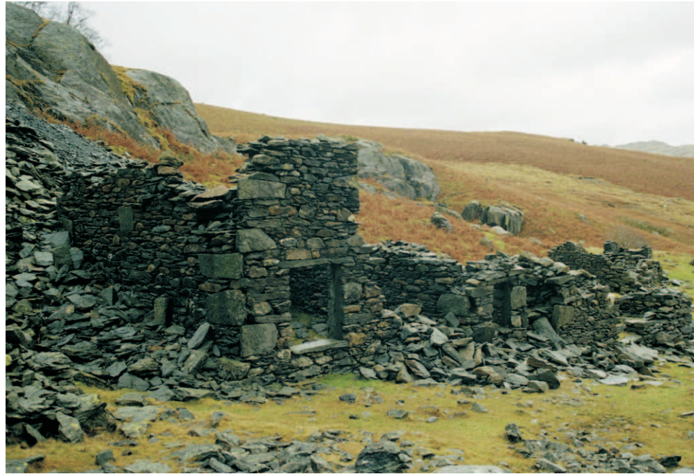
Figure 42 b. View of the accommodation, office and smithy from the south
