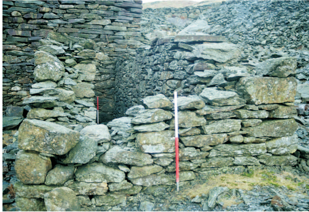
Figure 29. View of the wheel pit of Water Wheel 4 from the east
