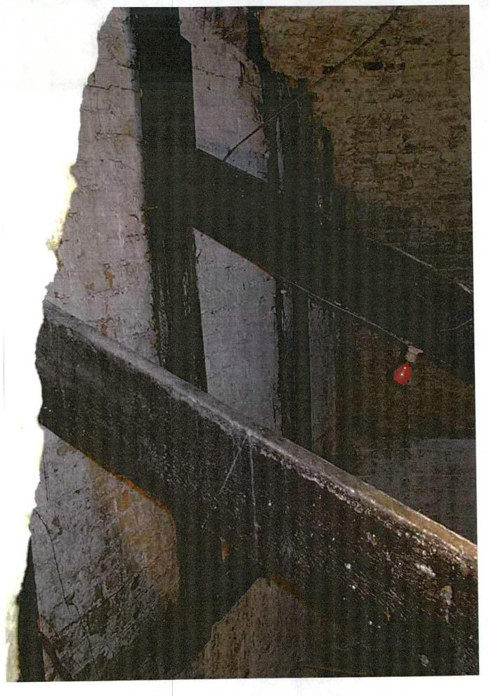
Figure 8; Photograph of the vertical wall which was added at the north-east of the ice house when it was part demolished
