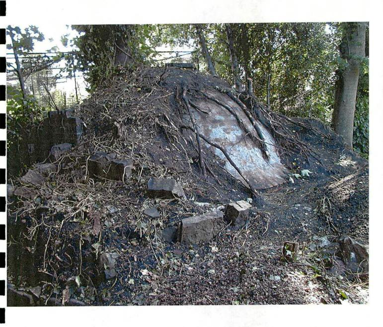
Figure 4; Photograph of the ice house from the west, showing an exposed area of its rendered brick dome
