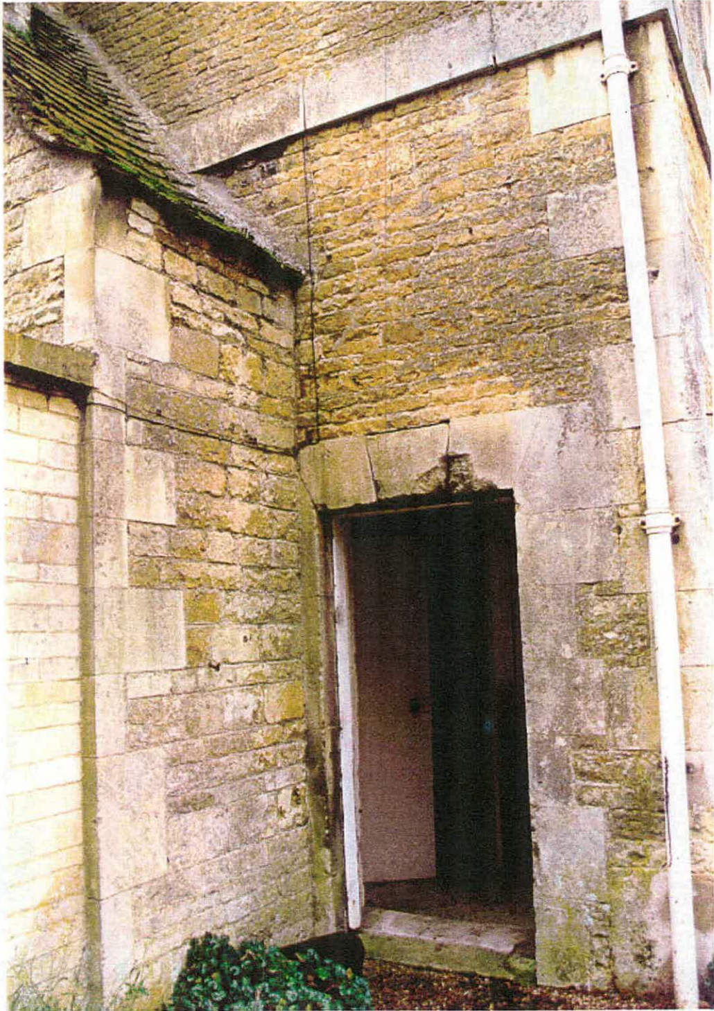
Fig. 21 The doorway with plain dressed jambs and head in the north elevation of the brewhouse. The left jamb stones are in part obscured by the base of the large chimney-stack.
