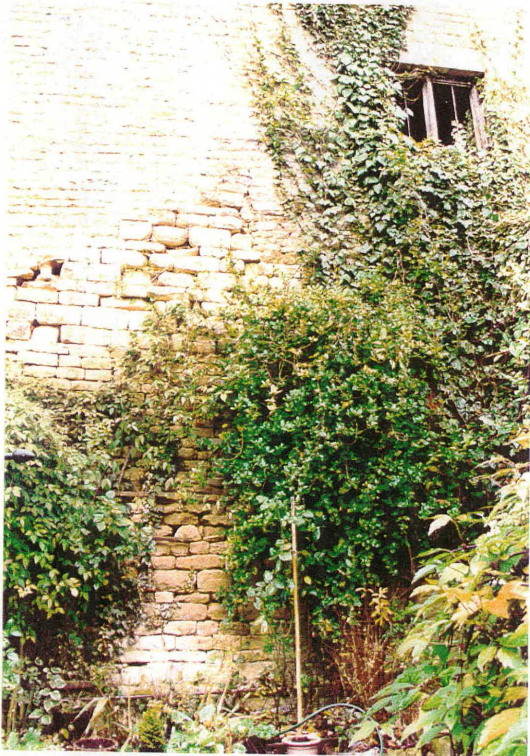
Fig. 26 This section of random coursed rubble walling on the east side of the brewhouse marks the position of a pre-Brown privy block with a lean-to roof, sloping here from right to left.
