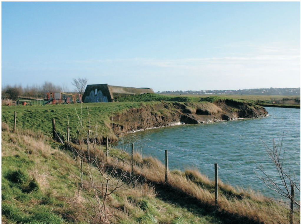
Figure 7 The eastern flanking position, with a magazine of the 1860s set back into the rampart. Note the severe erosion at the interface of rampart and ditch
