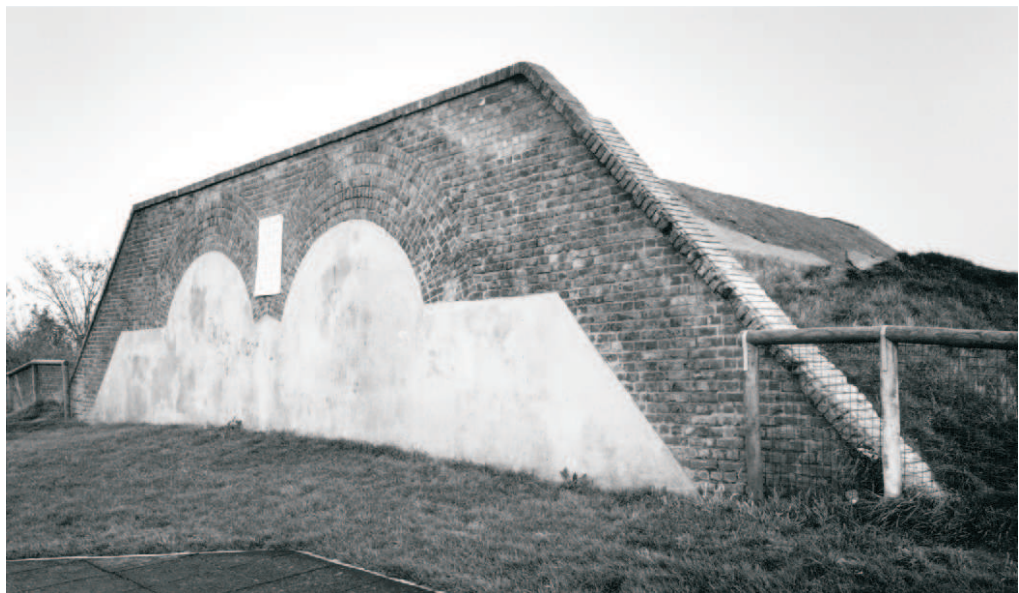
Figure 9 The blocked entrance façade of the eastern magazine, built in the mid 1860s. Note the erosion of the profiled earth covering at top right (NMR: AA008692)
