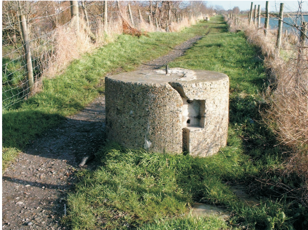
Figure 12 Second World War concrete cylinder, possibly for a searchlight or light weapon, on the rampart east of the A250 crossing
