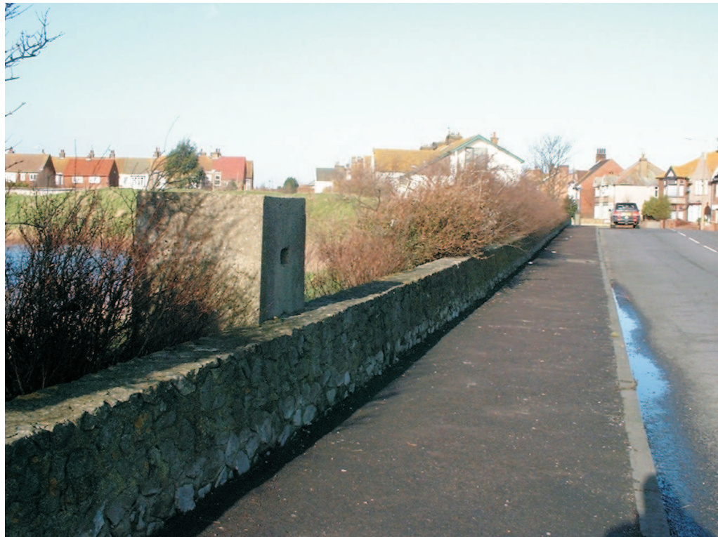
Figure 11 Second World War holding block, with a socket for a road barrier, at the crossing of the A250, looking north-west into Sheerness
