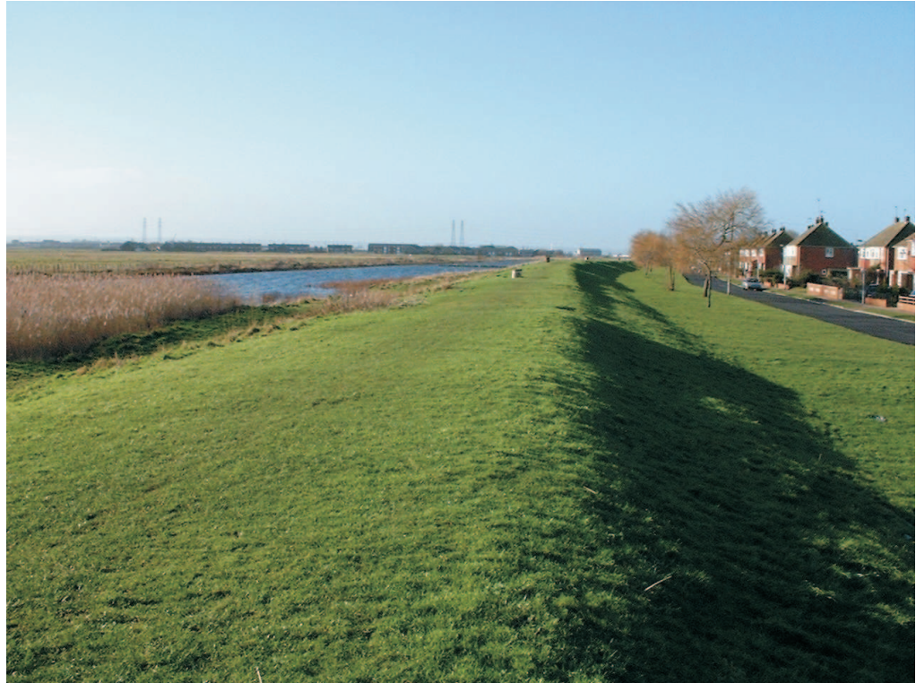
Figure 6 The rampart, central section, looking south-west from near the A250 crossing. The fire step is visible as a break in the shadow (middle distance) to the rear face
