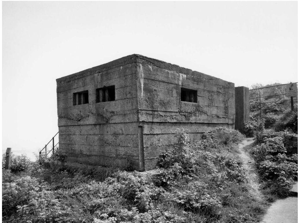
Figure 18 Photo of pillbox 12, from the north-west (NMR: AA99/09723 © Crown Copyright 1998)
