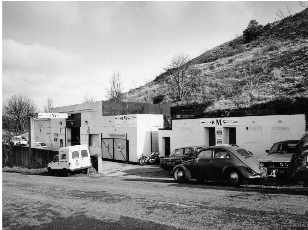
Figure 20 Photo of the REME workshop, from the north-west (NMR © Crown Copyright 1998)
