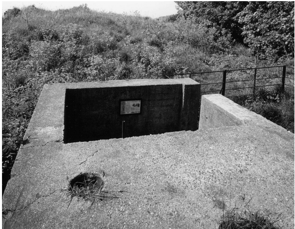
Figure 19 Photo of pillbox 12, showing a detail of the AA pit, from the north (NMR: AA99/09725 © Crown Copyright 1998)
