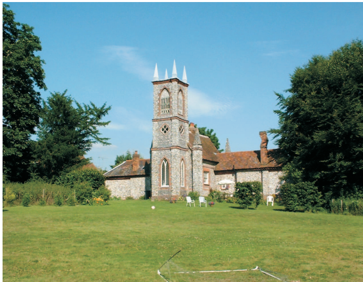
Plate 9: The miniature gothic church of St Crispin's. The tall tower provided an eyecatcher from the direction of the gardens some distance to the south-west.
