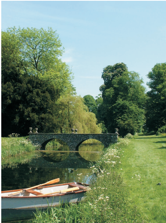
Plate 17: This 18th/19th-century footbridge connects the southern island with the shore.
