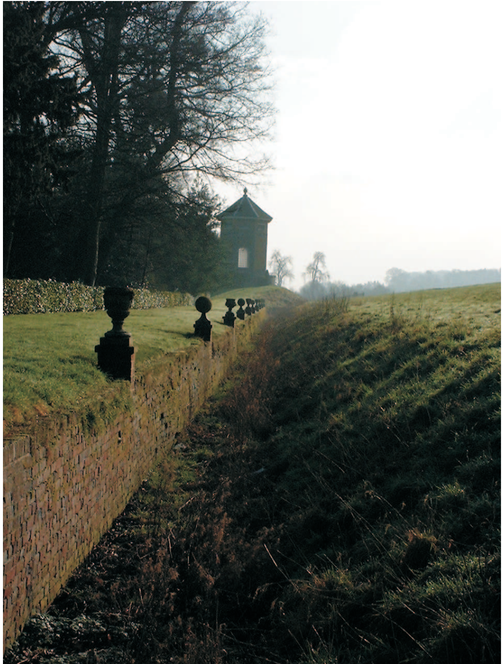
Plate 11: The line of the ha-ha to the south of West Wycombe House as it approaches the Temple of the Winds.
