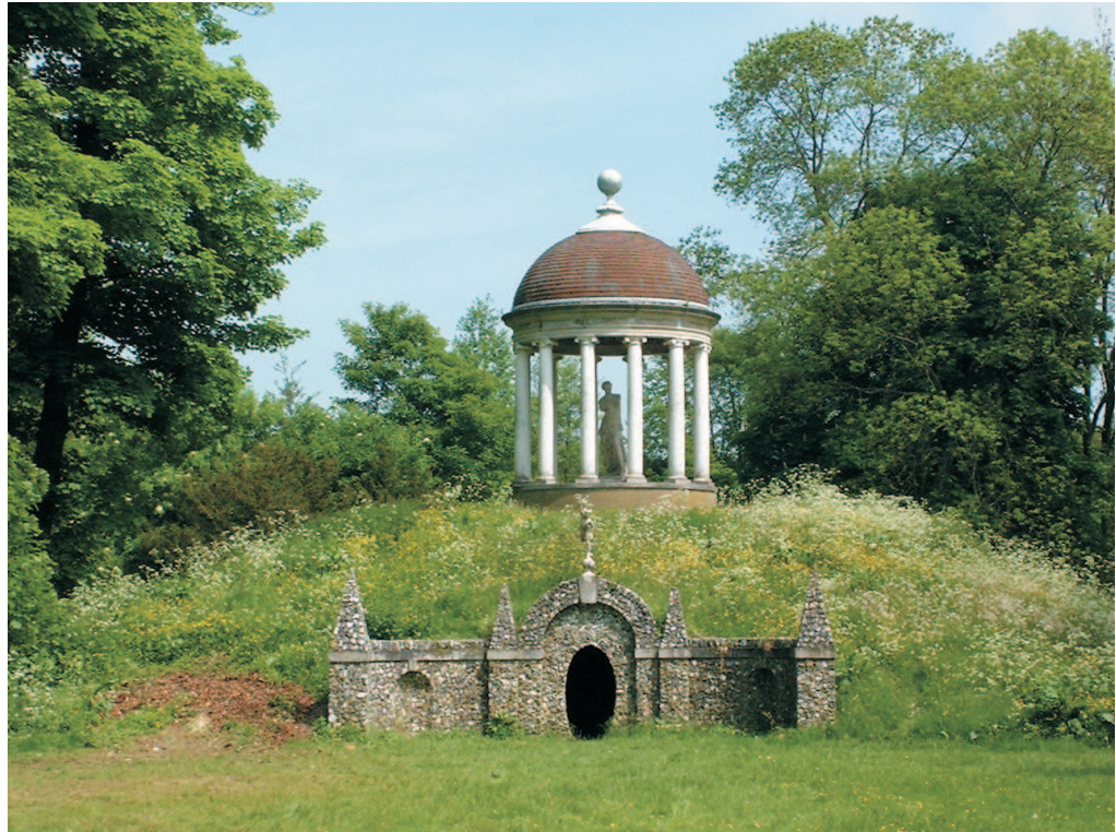
Plate 10: The Temple of Venus and its associated mound and niche seen from the south.
