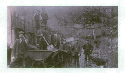
Figure 3: Colton Pits: working the west adit in 1908. Iron ore was tipped from the mine tramway wagons into these wooden bins. A light railway then took the ore up the incline (Hole Collection).
