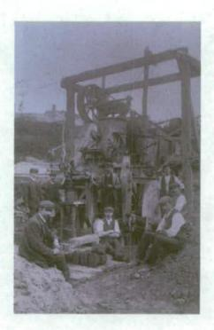
Figure 4: Washford briquetting plant c 1909. The poor quality ore from Colton was made into briquettes before shipping to the blast furnaces in south Wales, but the venture was short-lived (Hole Collection).
