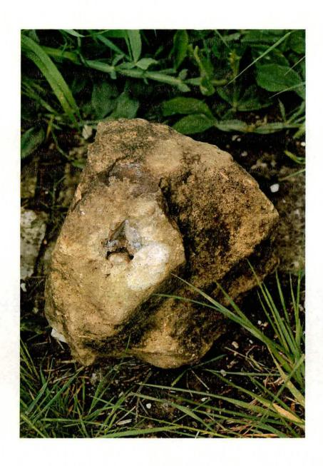
Fig. 12 A socket for a loose slate dowel
