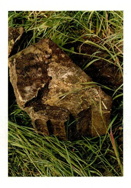
Fig. 10 Roll-and-fillet moulded window jamb
