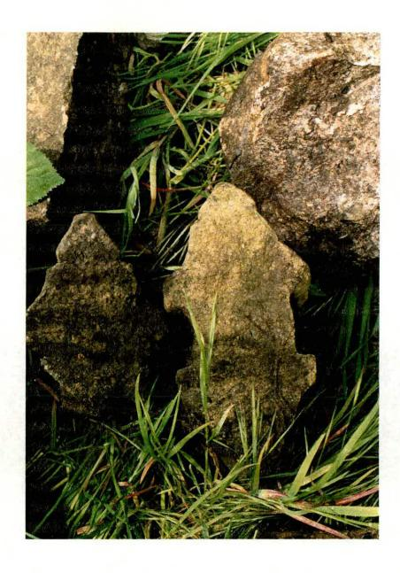
Fig. 9 Roll-and-fillet moulded window mullions
