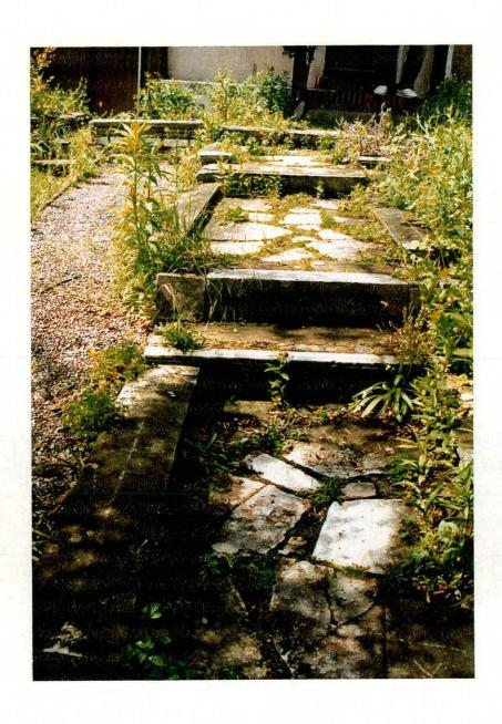
Fig. 3 The front garden path, composed of marble slab fragments and baluster rails
