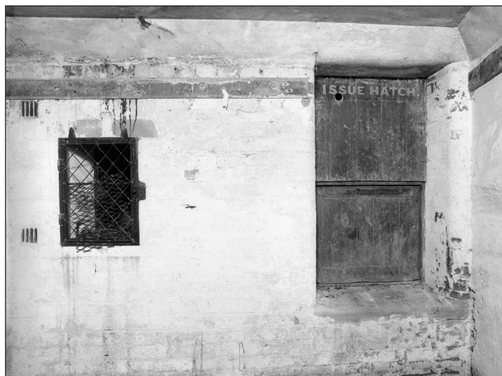
Figure 28 Grilled lamp recess and issue hatch of shell store (room 4) (AA00/8504)
