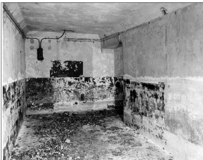
Figure 31 Surviving paintwork in gun casemate (room 15) (AA00/8509)
