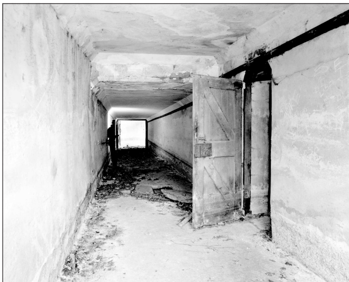
Figure 18 View along east gallery with entrance to shell store (room 18) on the right (AA00/8520)
