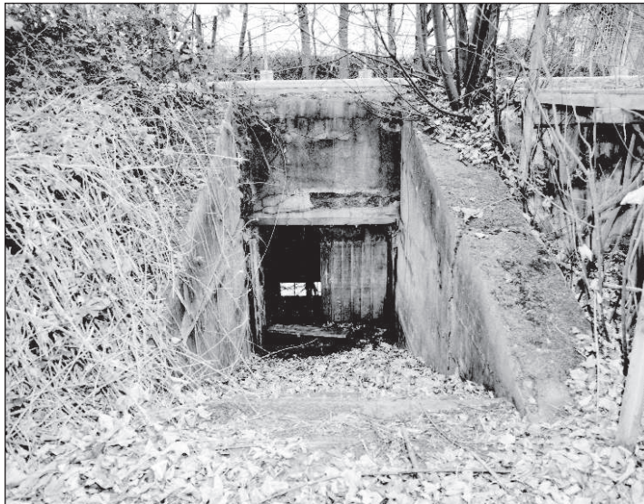
Figure 11 Eastern entrance to the gorge casemates (AA00/1071)
