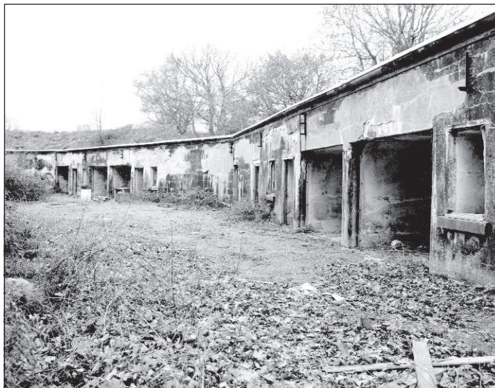
Figure 16 The front casemates and marshalling yard from the south east (AA00/8517)
