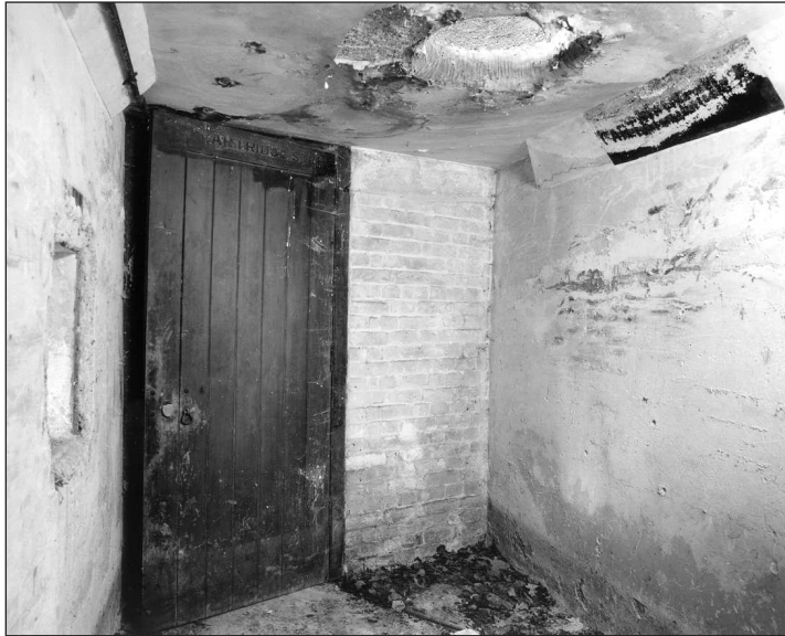
Figure 30 Door and lift shaft of room 12b (AA00/8503)
