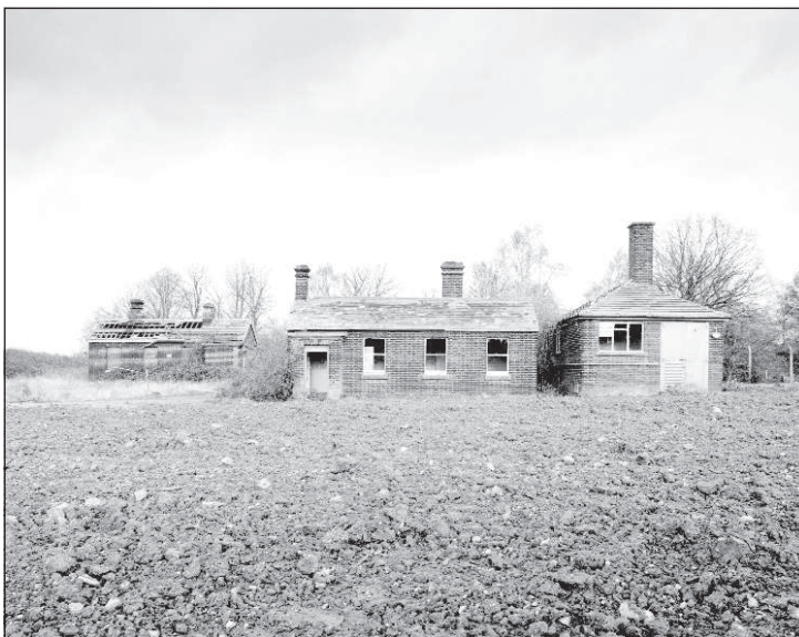
Figure 20 The Caretakers Quarters and structure associated with the ? tent and blanket store (AA00/1093)
