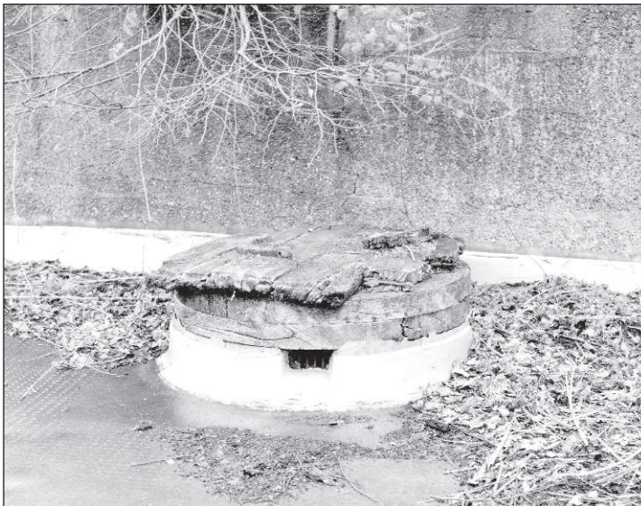
Figure 9 Ammunition lift hatch on the roof of the Front Casemates (AA008522)
