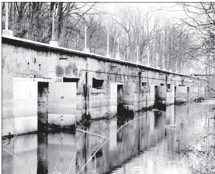
Figure 10 The gorge casemates (AA001081)
