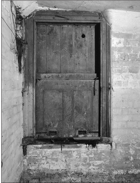
Figure 27 Issue Hatch of Cartridge Store (room 3) (AA00/8514)
