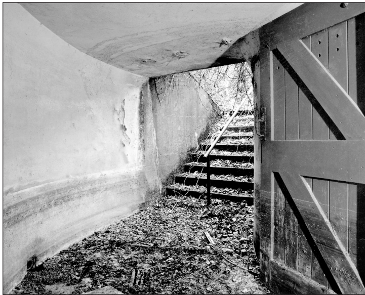
Figure 19 Stairway leading to the infantry positions on the gallery from the east gallery (AA00/8519)
