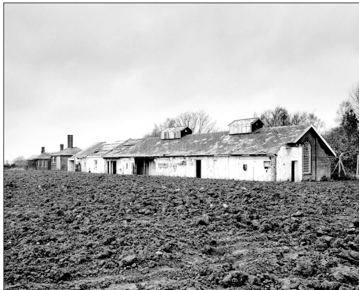
Figure 22 Exterior of the radio station workshop incorporating the 1903/04 Shell and Cartridge Stores (note the original large round headed window in the gable) (AA00/1085)
