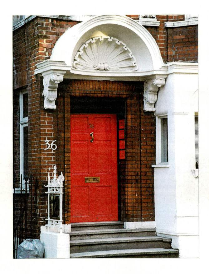
Fig. 29 Detail of the shell-hood porch of 1895-96 at No. 36 Bruton Street.
