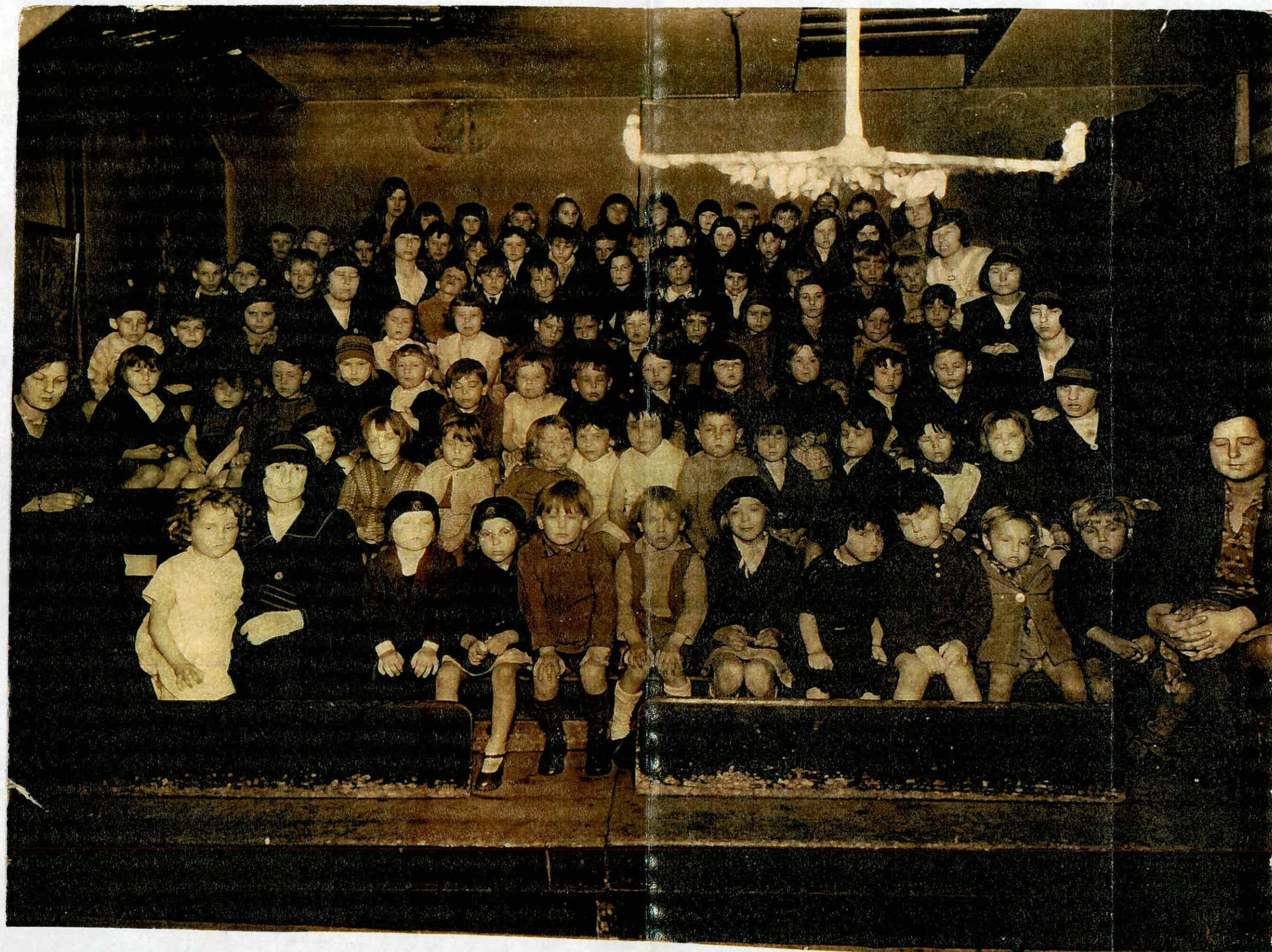
Fig. 11 Photograph taken c. 1945 showing a class of children in an unnamed room, clearly in need of repair.
