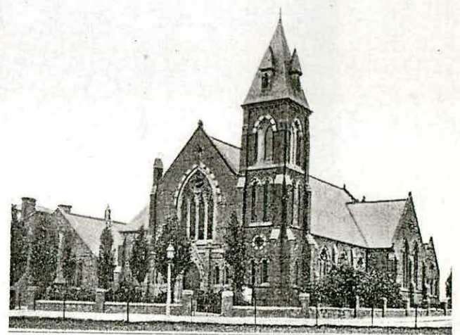
Fig. 20 Thomas Worthington's Brookfield Unitarian Church, Gorton, Manchester ( above ) built in 1871 is a good example of the style Sulman went on to develop in a more modest form. A Sunday School and hall preceded the church here, being built in 1863. Photograph of Wallington Baptist Church, Surrey) ( below ). Built in 1888, the church is extremely similar to Trinity Presbyterian Church (compare Fig. 4).
