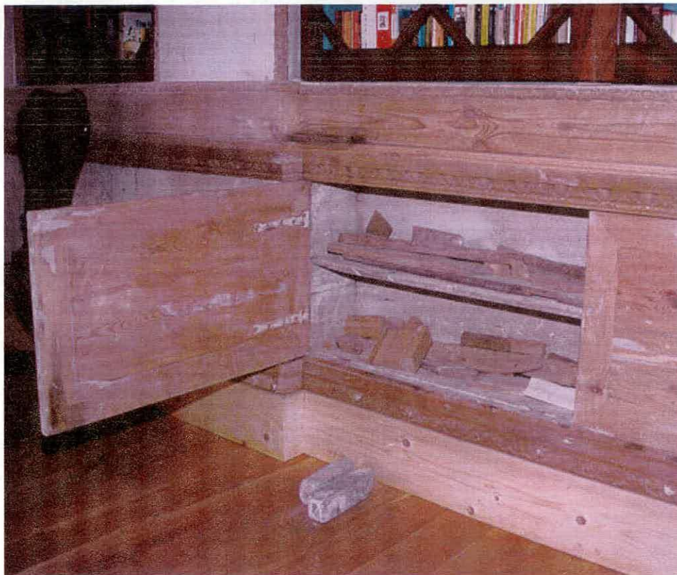
Figure 15, a cupboard door at dado level in the library at Barlaston, during restoration. Note the flush panel construction and long hinges.
