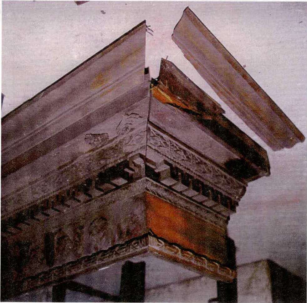
Figure 31, detail of the box cornice from the centre bookcase on the south wall, BC4.
