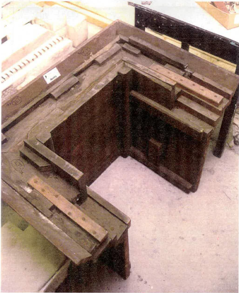
Figure 10, the back of the block pediment showing the crude Victorian method of assembly using glued battens and screws.
