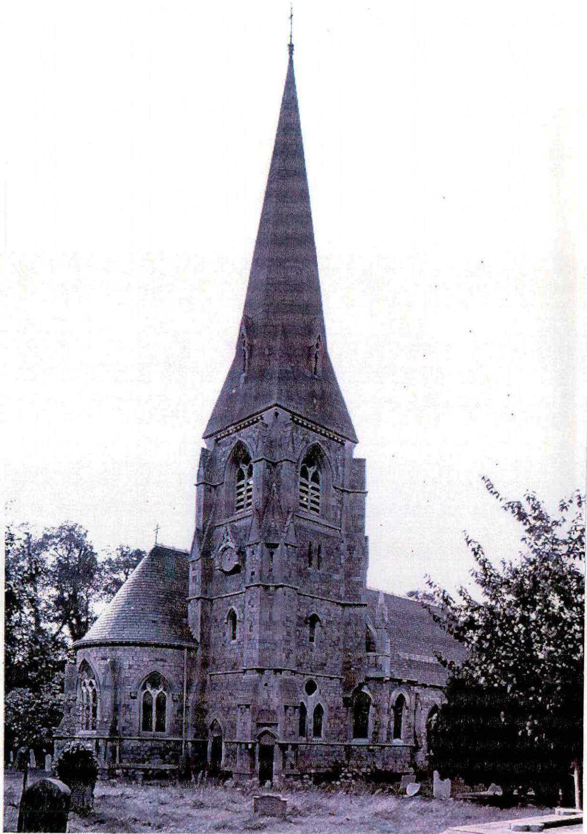
Figure 8, the church viewed from the north east, in 1991 (photograph English Heritage)
