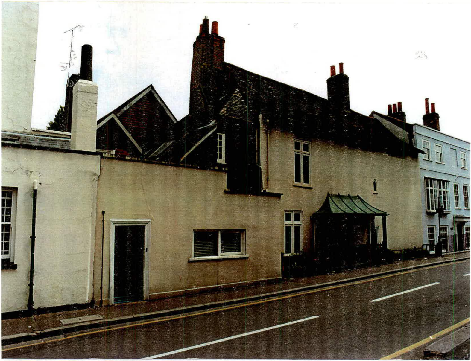
Figure 20: Wolsey Cottage viewed from the north west.
