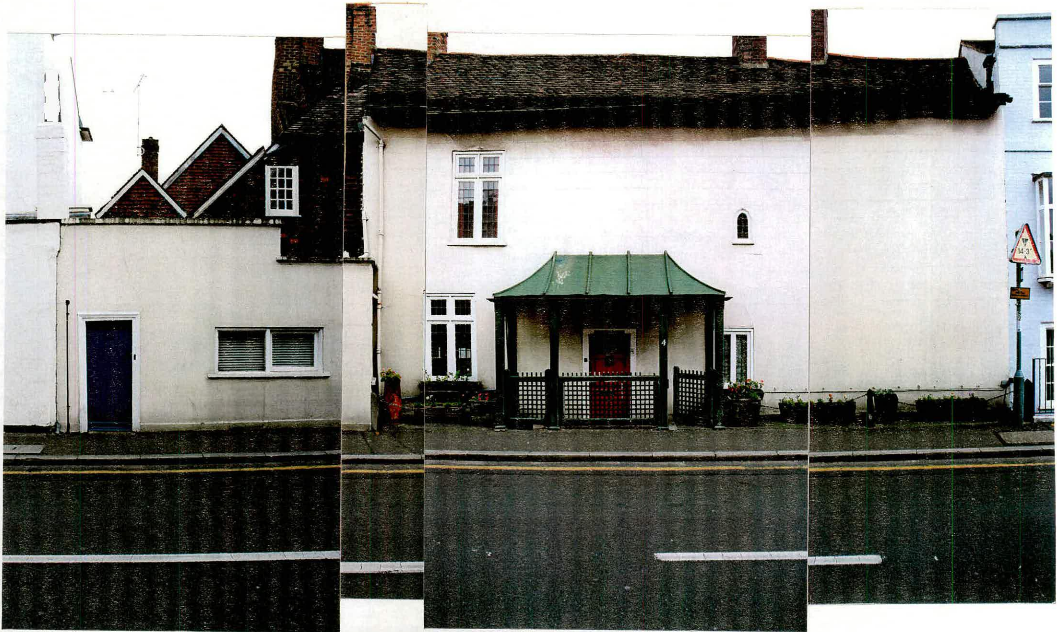
Figure 29; a composite photograph of the west façade
