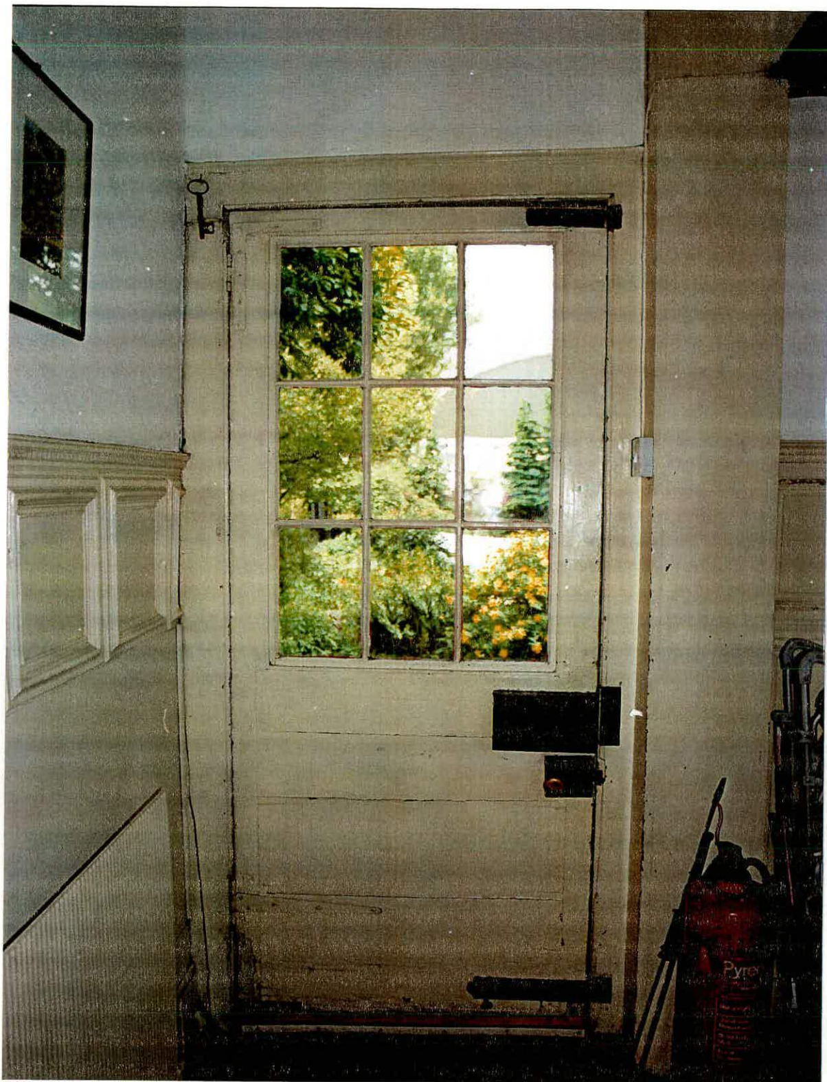
Figure 23; the inside of the back door.
