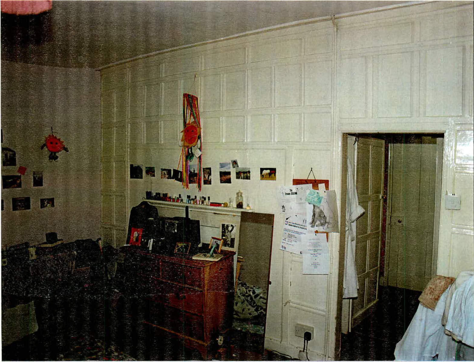
Figure 24; first floor bedroom above the dining room, looking north west.
