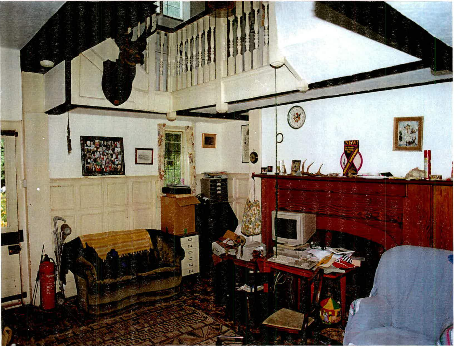
Figure 21; the hall looking south east. The difference between two first floor levels can be seen either side of the large black beam in the left of the picture.
