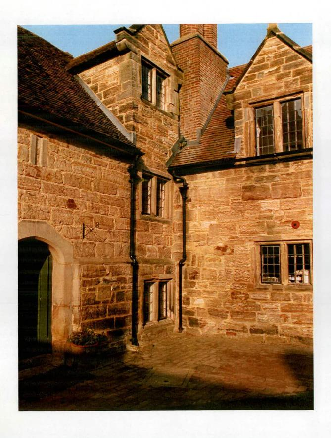
Fig. 15: The north-east corner within Old Stable Court. The plinth and string of the north range are cut by the addition of the east range.
