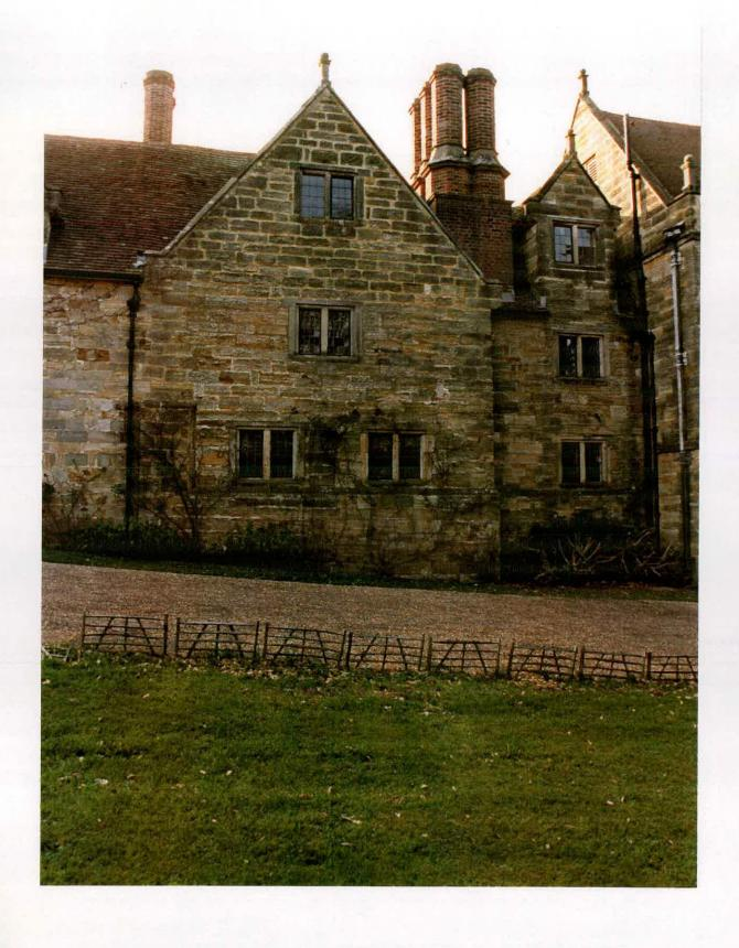
Fig. 14: The east gable of the north range in Old Stable Court. Note the plinth and its string which continue on to the projecting one-bay extension to the right. To the left, there is a straight joint with the east range of Old Stable Court, where the plinth and string disappear.
