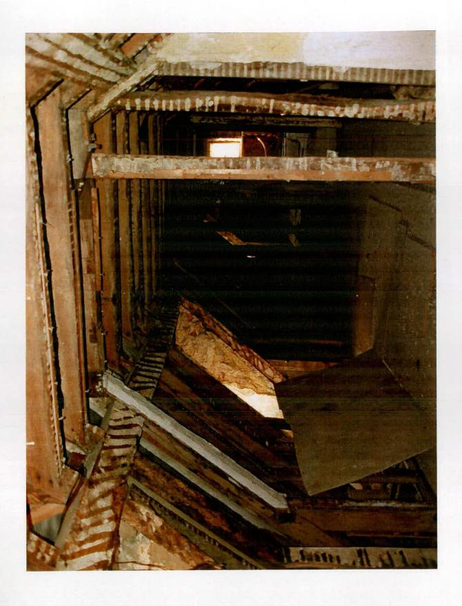
Fig. 7: A general view of the roof timbers in the north range of Old Stable Court, looking west. The construction employs tenoned purlins, with staggered detailing.
