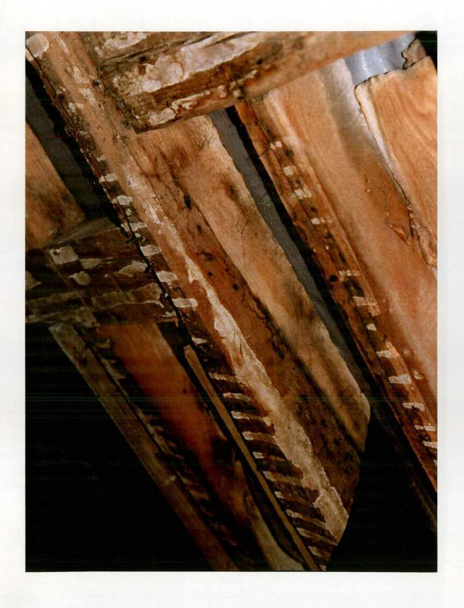
Fig. 8: Detail of staggered purlins in the roof of the northern range in Old Stable Court.
