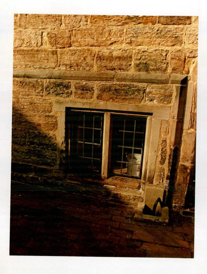
Fig. 13: One of the two-light windows which open from the southern side of the north range in Old Stable Court. Although the mullion has been renewed, there is enough evidence to suggest that the plain chamfer detailing is original.
