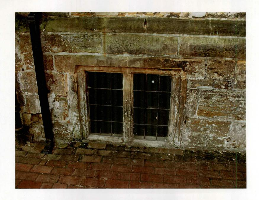
Fig. 12: Two-light window looking into the basement on the north side of the main house. The mullion and jambs appear to be original and feature sunk chamfers.
