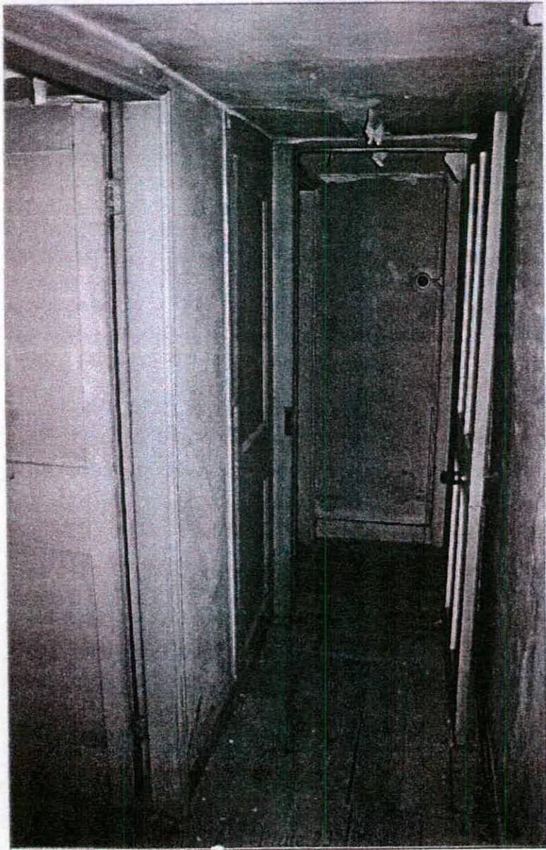
Late 18th century accommodation in roof space, accessed by private back stair. Rooms of basic form clearly intended for domestic use (1999)
