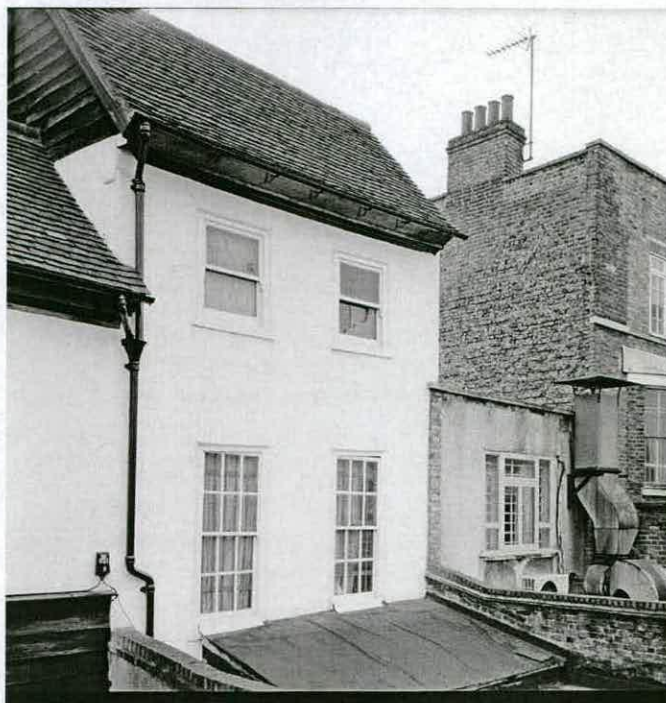
Fig. 12 - No. 58 Peckham High Street, view from over shop extensions showing upper-storey façade in 1998 (RCHME, BB99/00123).
