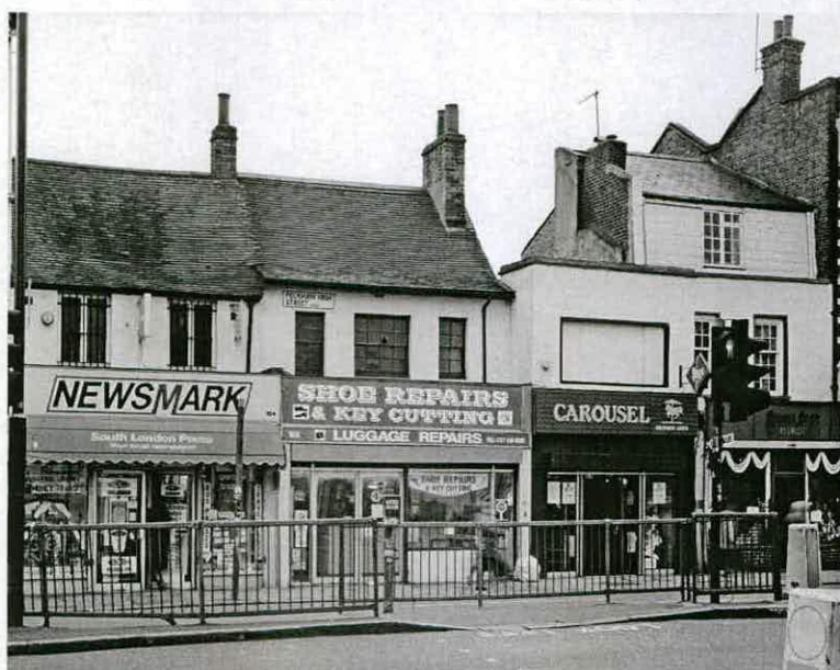
Fig. 16 - Nos 98-104 Peckham High Street, view from the north in 1998 (RCHME, BB99/00120).
