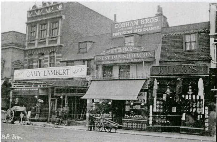
Fig. 18 - Nos 100-104 Peckham High Street, view from the north in 1928 (RCHME, NMR inventory card).
