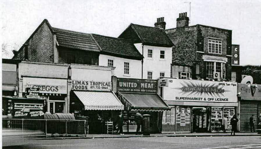
Fig. 4 - Nos 58, 60 and 62 Peckham High Street, view from the northeast in 1998 (RCHME, BB99/00122).
