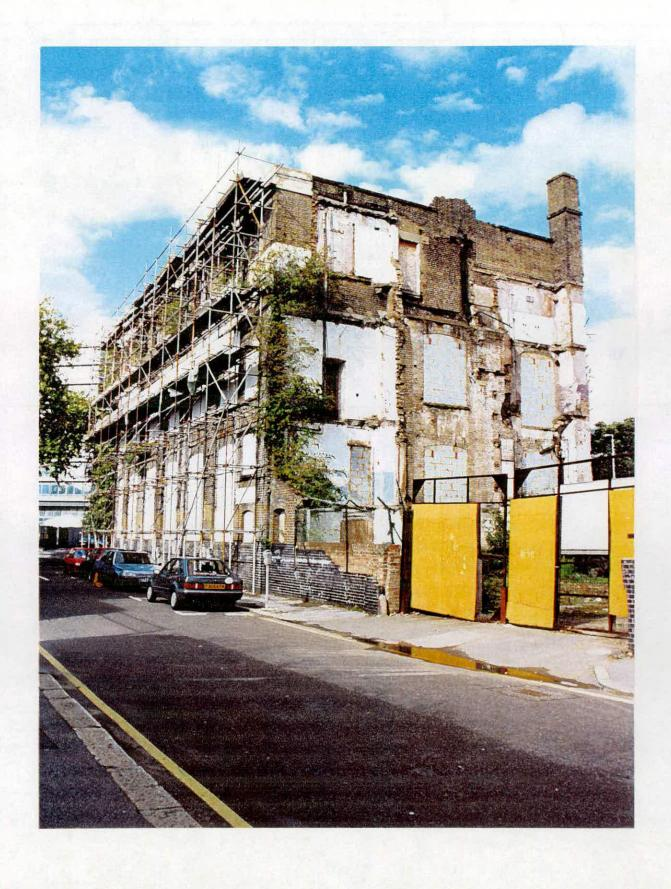
Fig. 13 The south side of the chapel showing scars marking the removal of the post-1901 extensions. At the centre and to the right the large blocked openings are presumably windows of the original chapel.
