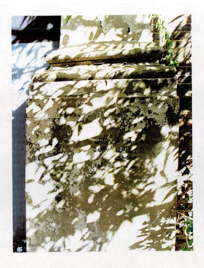
Fig. 7 Corner pilaster plinth and base at the north-west corner of the chapel. The base is of perfectly correct Doric form.
