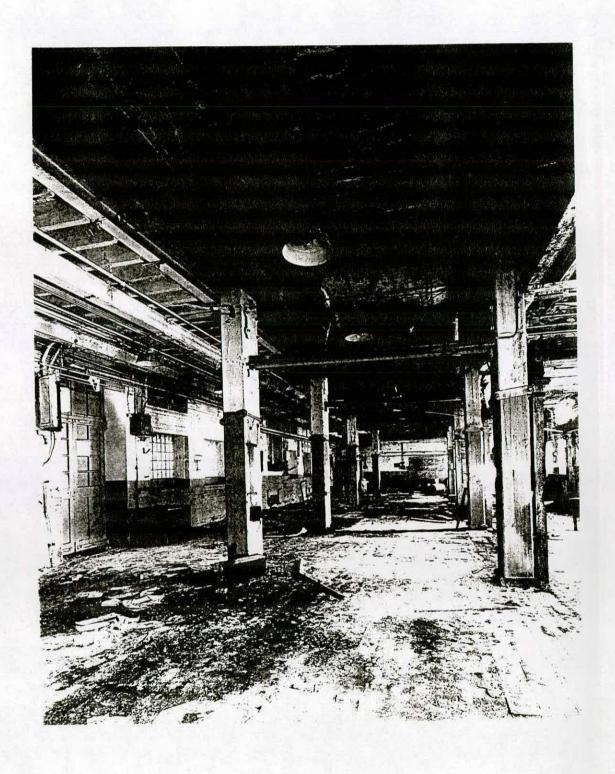
Fig. 15 The interior of the 'chapel' looking south, as it appeared in 1977. It would appear that all trace of the original fittings had been removed by this time, with the heavy uprights supporting an upper floor in the later factory. To the sides, gallery-like features cannot be too far removed from the position of the chapel originals.
