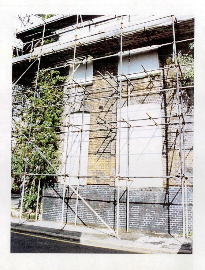
Fig. 11 Detail of window openings on the west side of the chapel, showing the narrower bay at the northern end. The brick used in the segmental heads was the same as that in the plinth.
