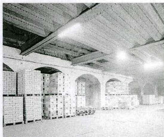
Fig. 9 - Low-level goods shed, rail access roofed-over in c.1915 with steel-trough flooring (RCHME, BB98/26506).
