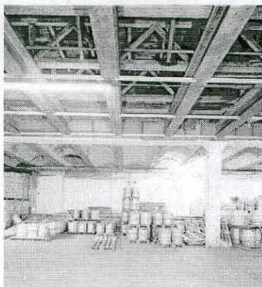
Fig. 8 .- Low-level goods shed, interior showing timber trusses supporting the platforms above (RCHME, BB98/26509)
