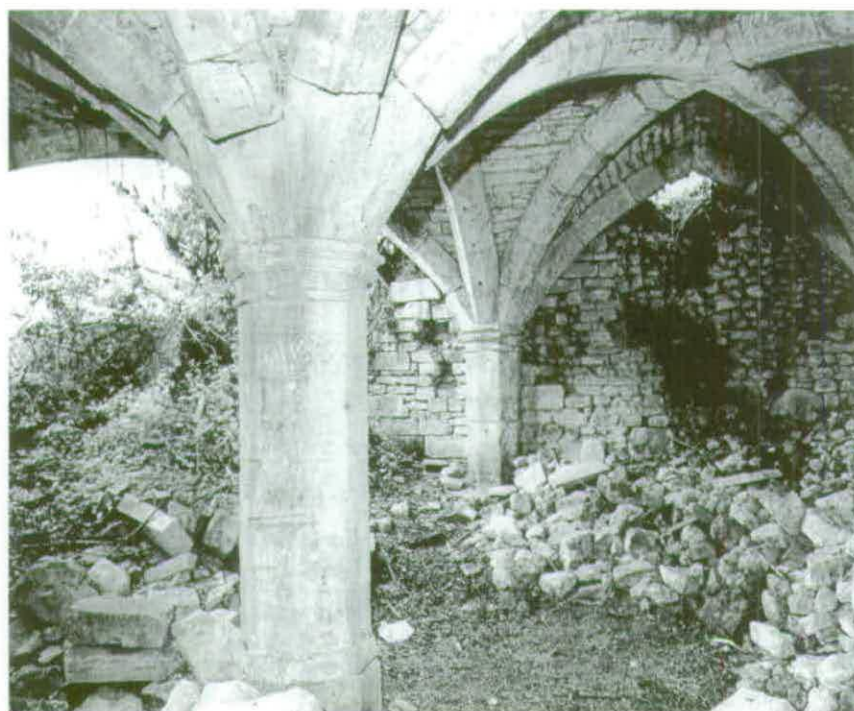
Plate 1. The undercroft in the West Range (NMR: 97/3474. AA97/7222)
