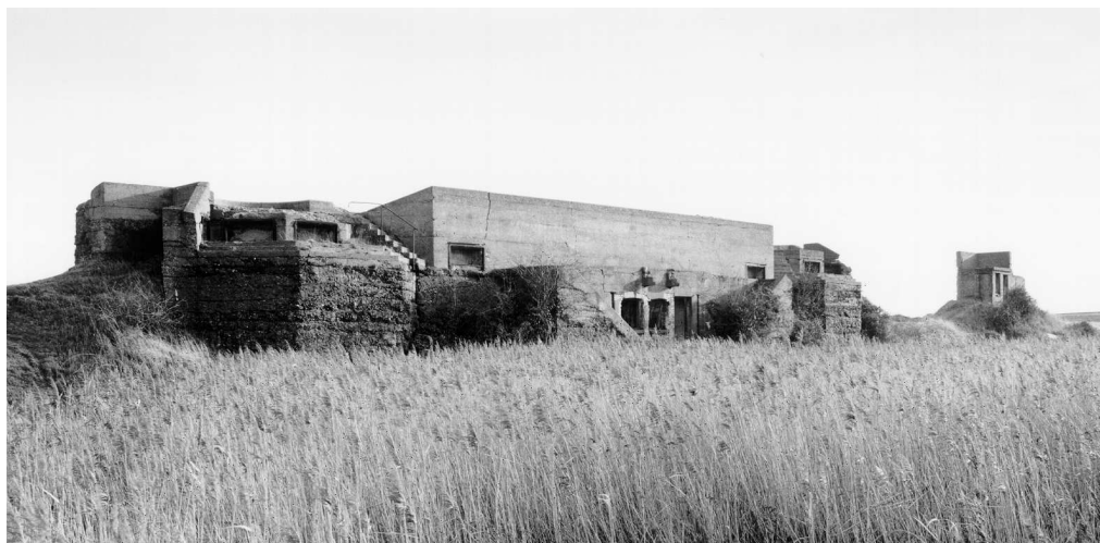
Figure 33 Dummy Battery showing the magazine entrance, steps to the gun emplacements and the BC post to the right (NMR: AA98/07945)
