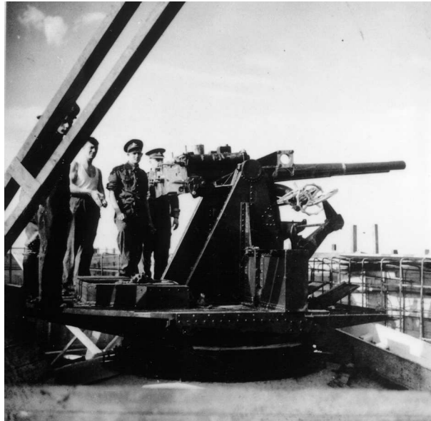
Figure 17 Contemporary photograph showing the installation of the Twin 6-pounder gun in 1941 (PRO: WO/192/223)
