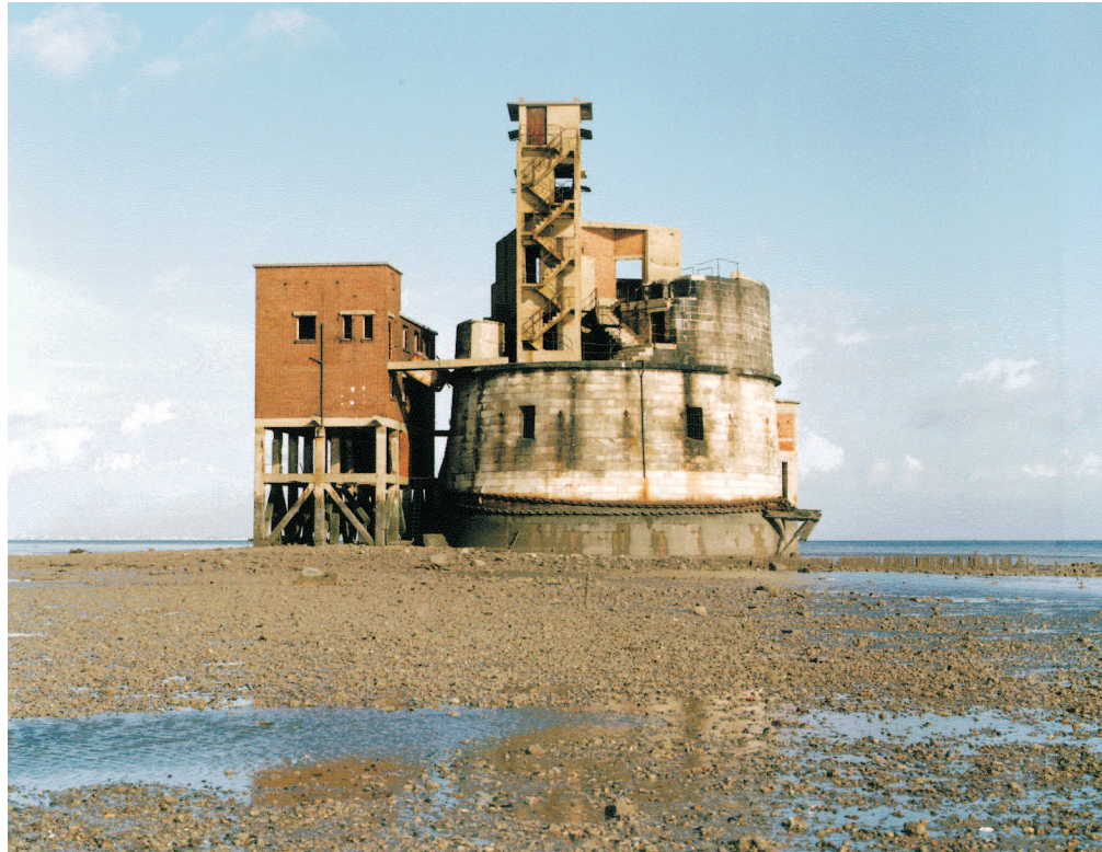
Figure 5 Grain Tower; view from the south-east across the mudflats (NMR: AA98/07914)
