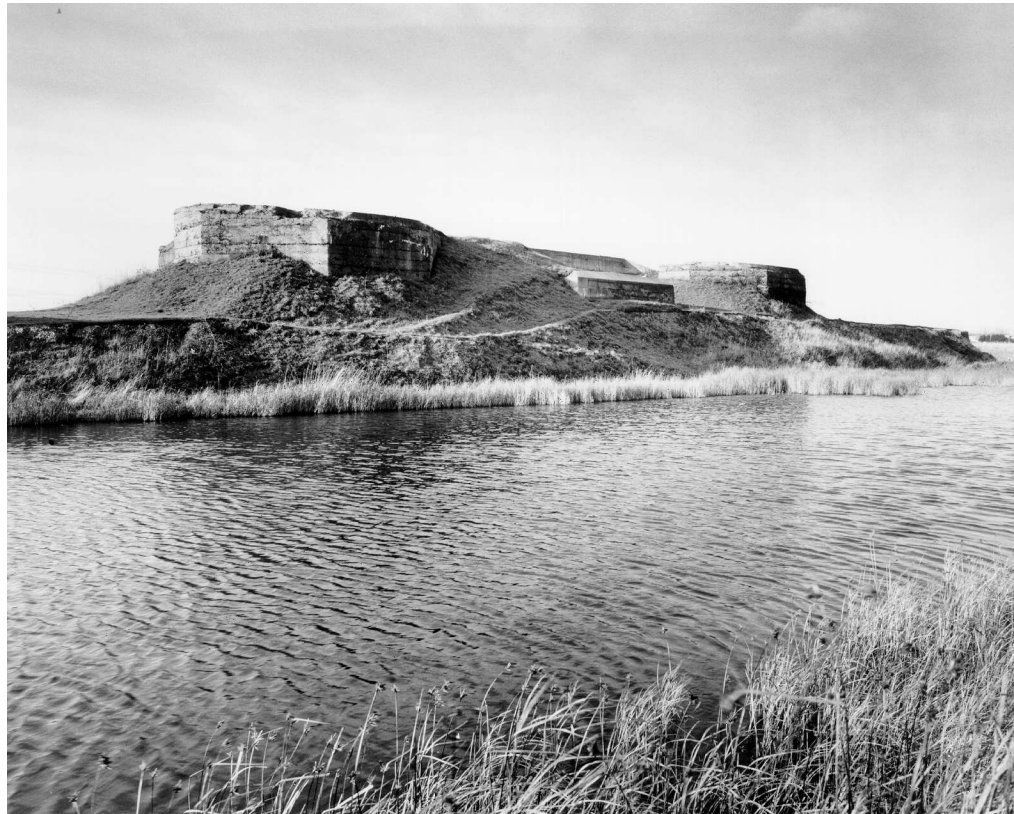
Figure 29 Dummy Battery from the south-east, showing the exposed concrete of the 4.7-inch QF battery and the standing water in front
