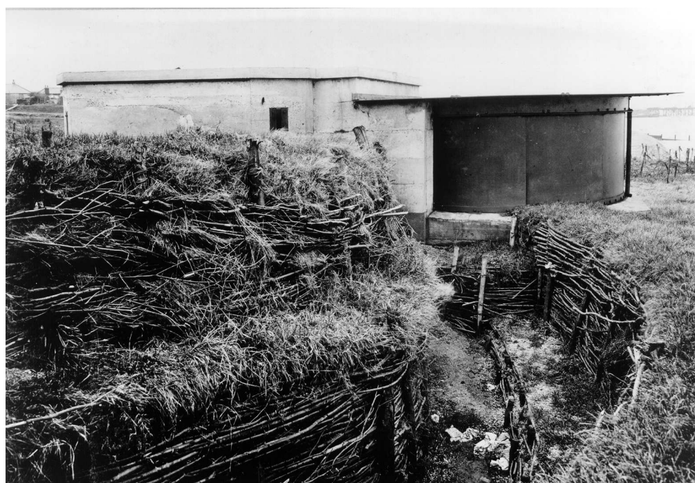
Figure 42 Electric searchlight emplacement at Grain during the First World War, with part of the extensive trench system in the foreground. Note the apsidal end with its steel shutters guarding the lights (reproduced courtesy of the Royal Engineers Library, Chatham: 779/940.3(42))
