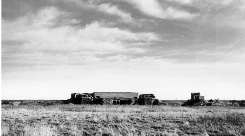
Figure 30 Dummy Battery from the rear showing the two 4.7-inch QF gun emplacements, the magazine between them, and the BC post to the right (NMR: AA98/07943)
