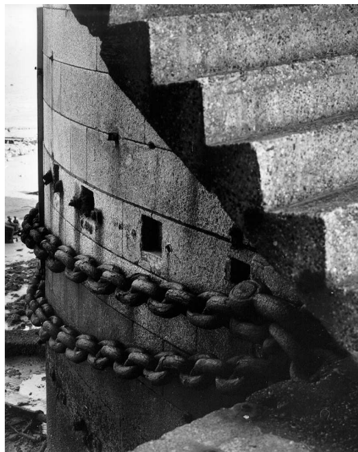
Figure 8 The anchor chain for the Medway Boom and sockets for the wooden supports for the landing stage (NMR: AA98/07892)
