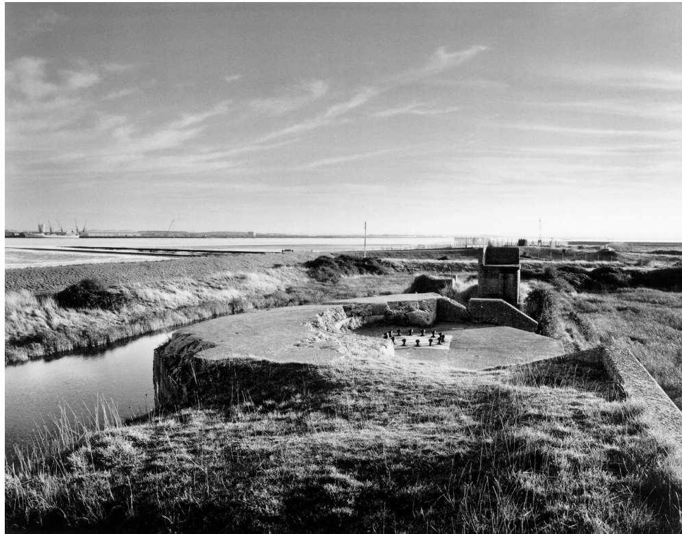
Figure 32 The southern 4.7-inch QF gun emplacement showing the holdfast bolts (NMR: AA98/07949)
