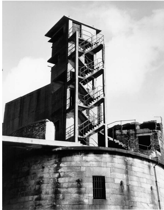
Figure 18 The Battery Observation Post from the south (NMR: AA98/07887)
