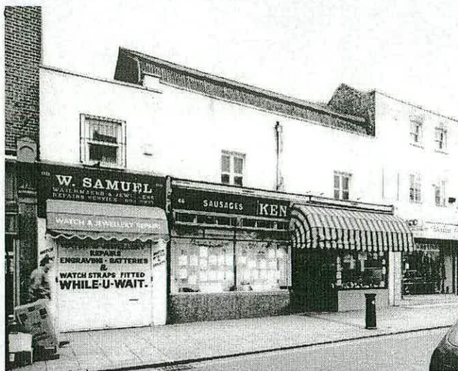
Figure 38 - Nos 62-66 Deptford High Street, 1790-1, front elevations from the northwest (RCHME, AA98/01665).
