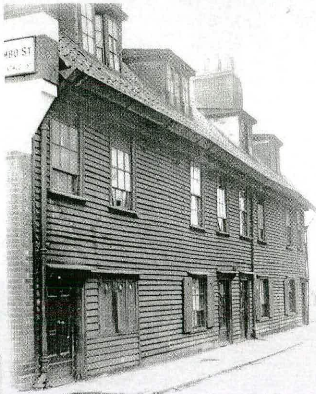
Figure 55 - Nos 72-80 Colombo Street, Southwark, one-room-plan houses of c.1700, demolished (NMR).
