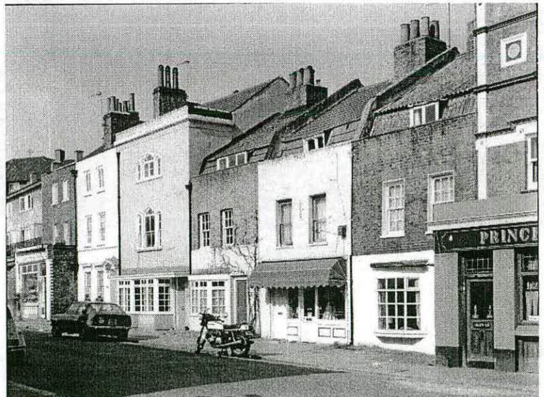
Figure 60 - Nos 74-78 Royal Hill, Greenwich, mid/late-18th-century centre-chimney-plan houses (NMR, P. Barkshire Collection, No. 2289, 1983).
