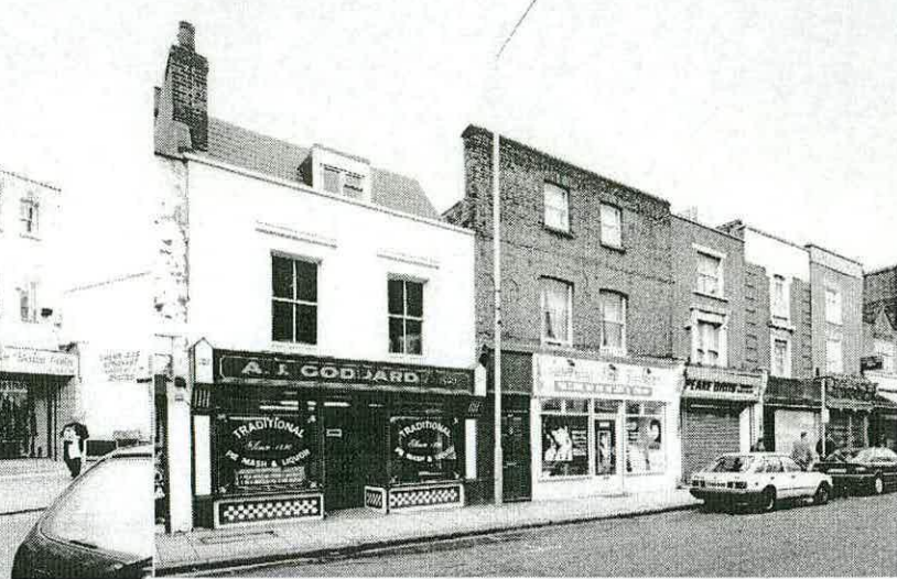
Figure 39 - Nos 203 and 205 Deptford High Street, 1775-6 and 1774-5, front elevations from the southeast (RCHME, AA98/01692).
