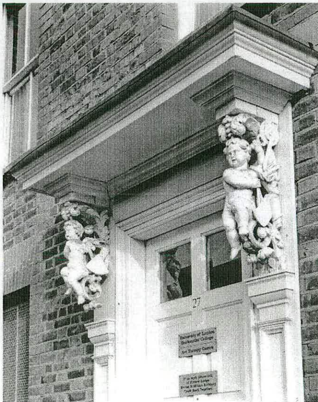
Figure 40 - No. 27 Albury Street, c.1710 doorcase detail (NMR, P. Barkshire Collection, No. 1401, 1981).
