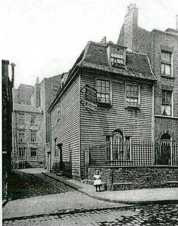
Figure 49 - Wellclose Square, Whitechapel, in 1913, 18 th -century timber house, demolished (NMR, BB74/806).
