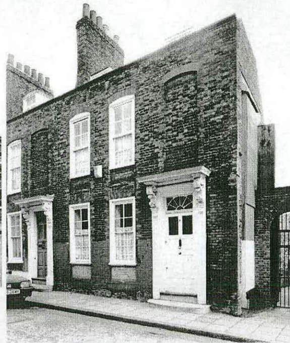
Figure 34 - No. 34 Albury Street, c.1710, front elevation (RCHME, BB97/1642).
