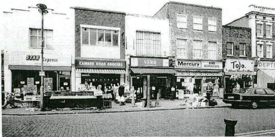
Figure 62 - Nos 53-61 Deptford High Street (RCHME, AA98/01679)
