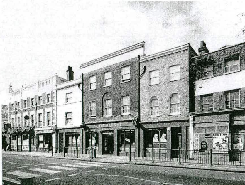
Figure 68 - Nos 217-227 Deptford High Street (RCHME, AA98/01697).
