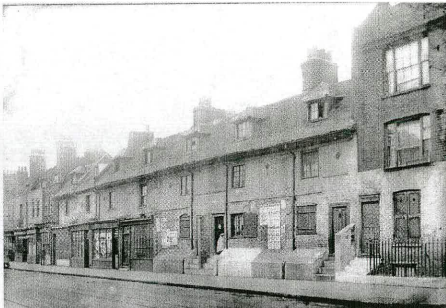
Figure 54 - Dog Row, Cambridge Heath Road, Bethnal Green, one-room-plan houses of c.1678, demolished (NMR, BB60/1202).
