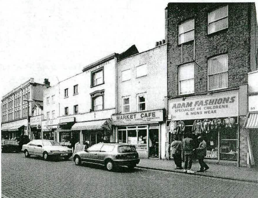
Figure 64 - Nos 73-79 Deptford High Street (RCHME, AA98/01681).
