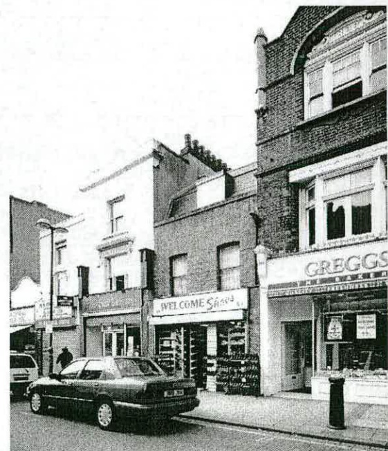
Figure 65 - Nos 85-89 Deptford High Street (RCHME, AA98/01685).
