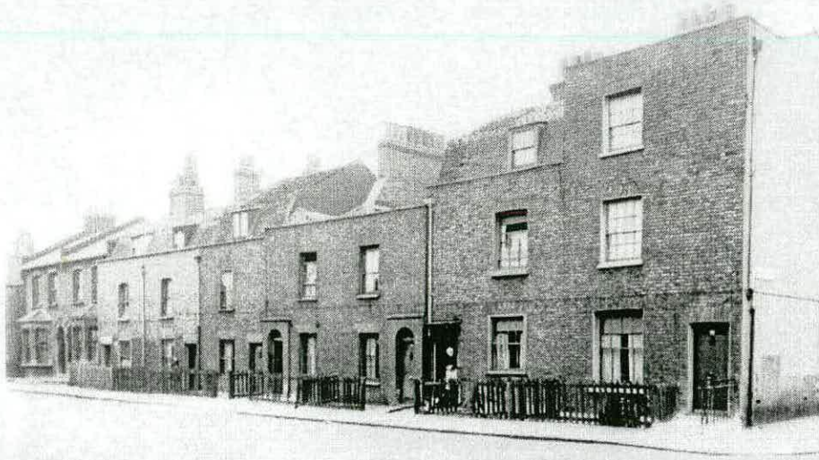
Figure 17 - Nos 14-26 Edward Street of c.1790 in 1949 (London Metropolitan Archives, 98/048).
