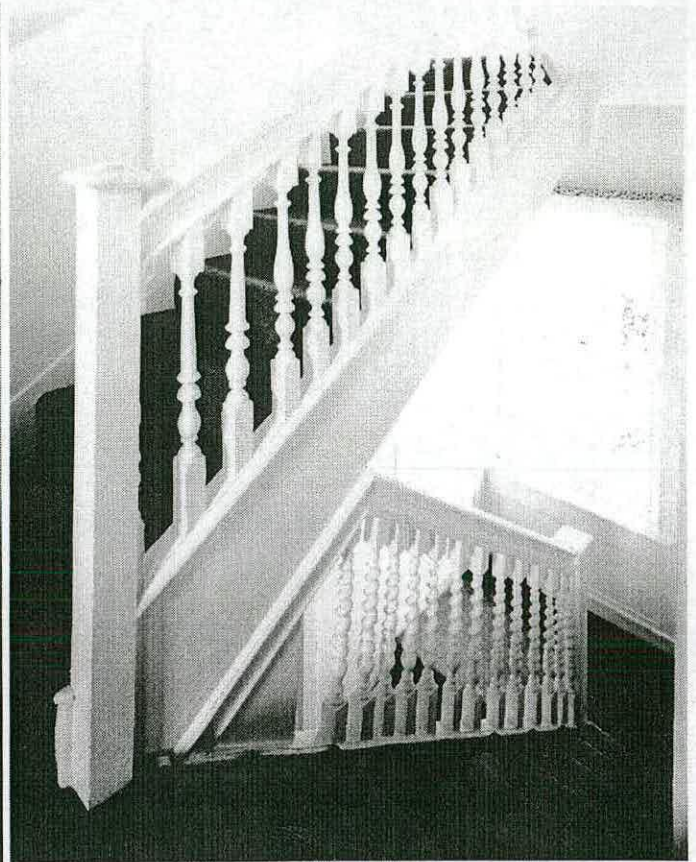
Figure 45 - Albury Street, c.1710, staircase detail (RCHME, BB97/1483).
