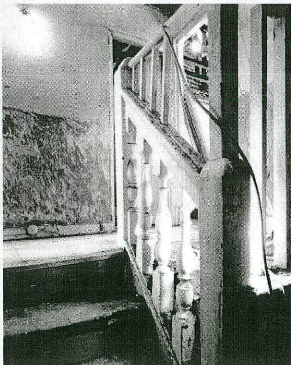
Figure 43 - No. 20 Deptford Broadway, late-17th-century staircase detail (RCHME, BB98/03090).
