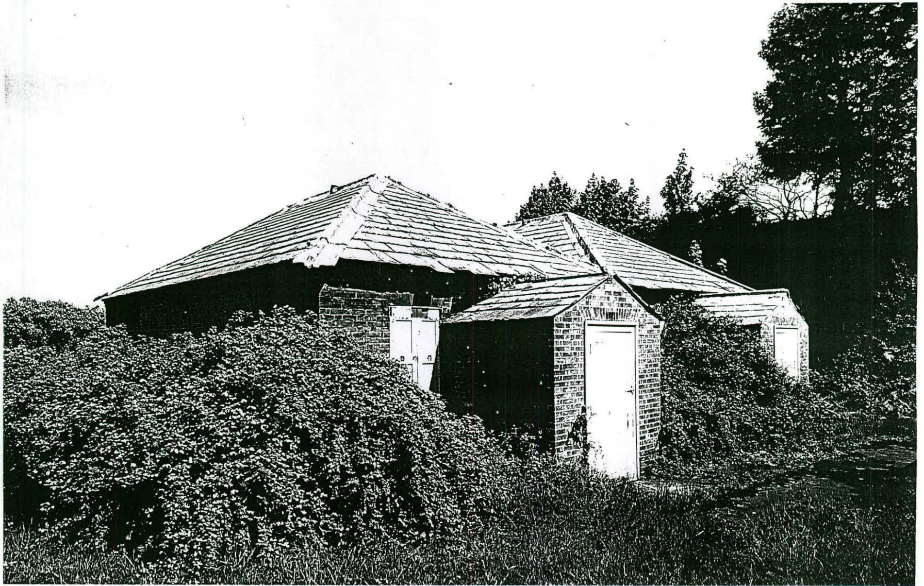
12e. Marchwood: former shifting house, to north-east. 1972
