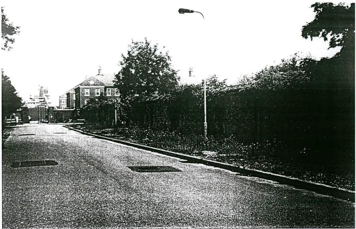
Marchwood: outer walls of former E Magazine (along Quayside Walk), to north
