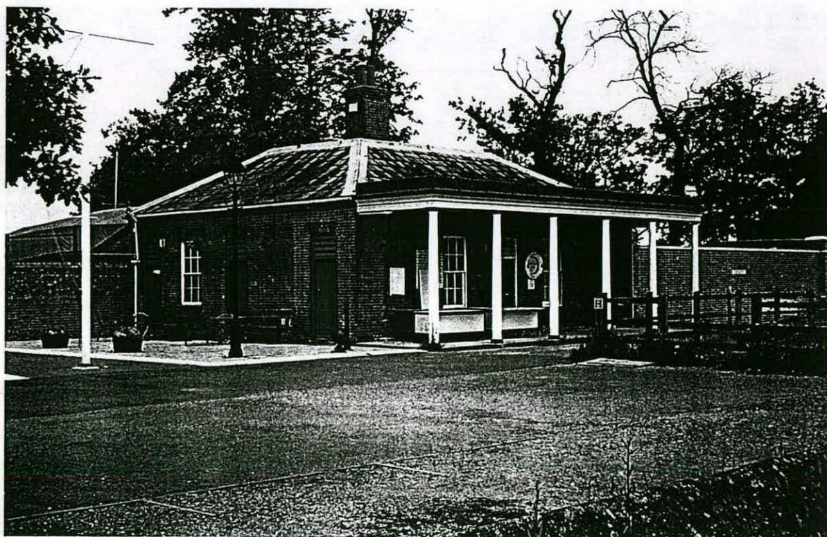
Former guard room, to north-west
