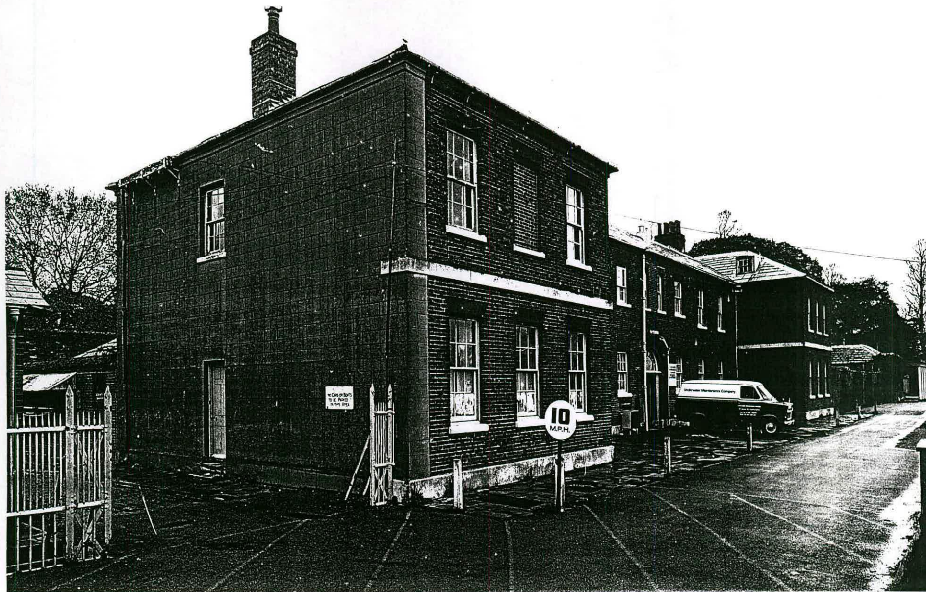
12a. Marchwood: Former barracks to North. 1972
