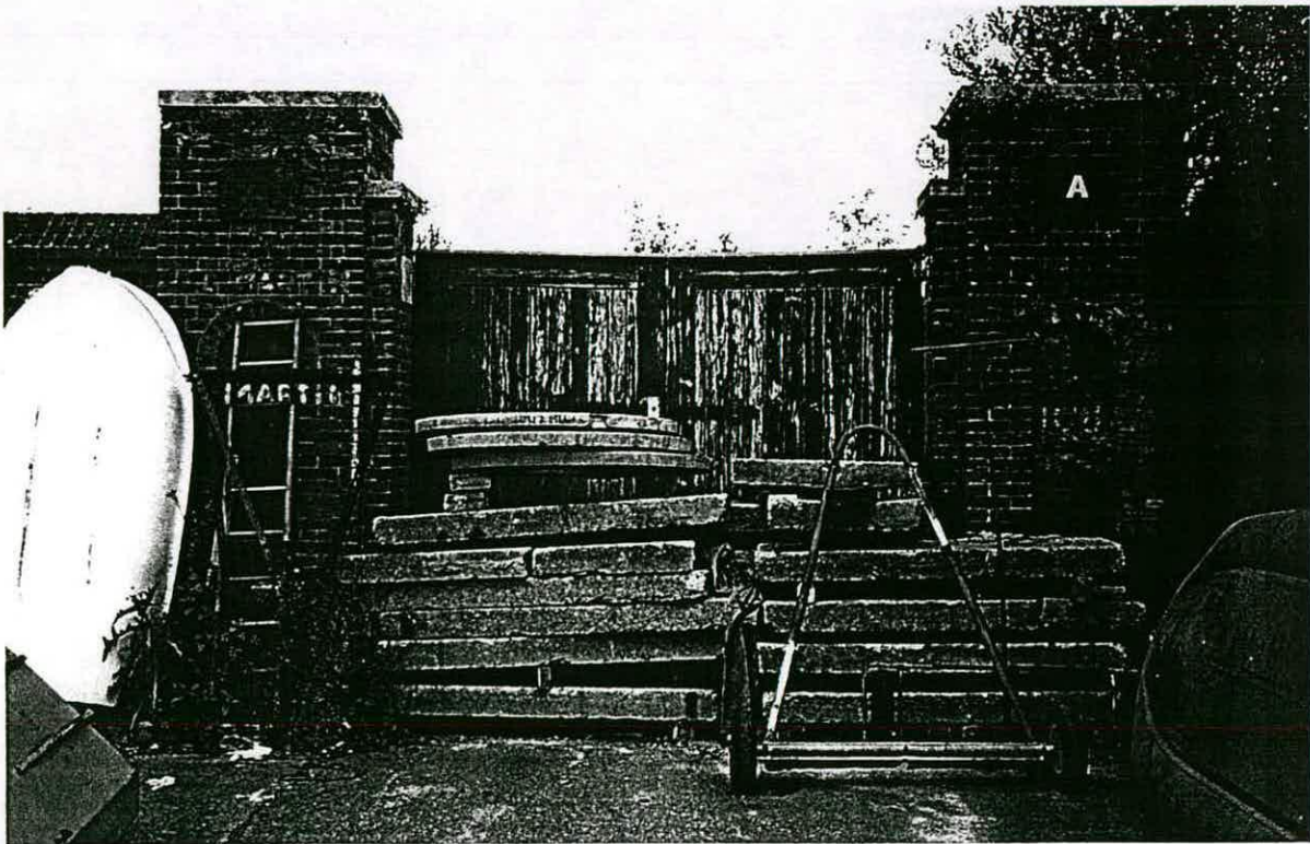
Gate piers to A Magazine, to north
