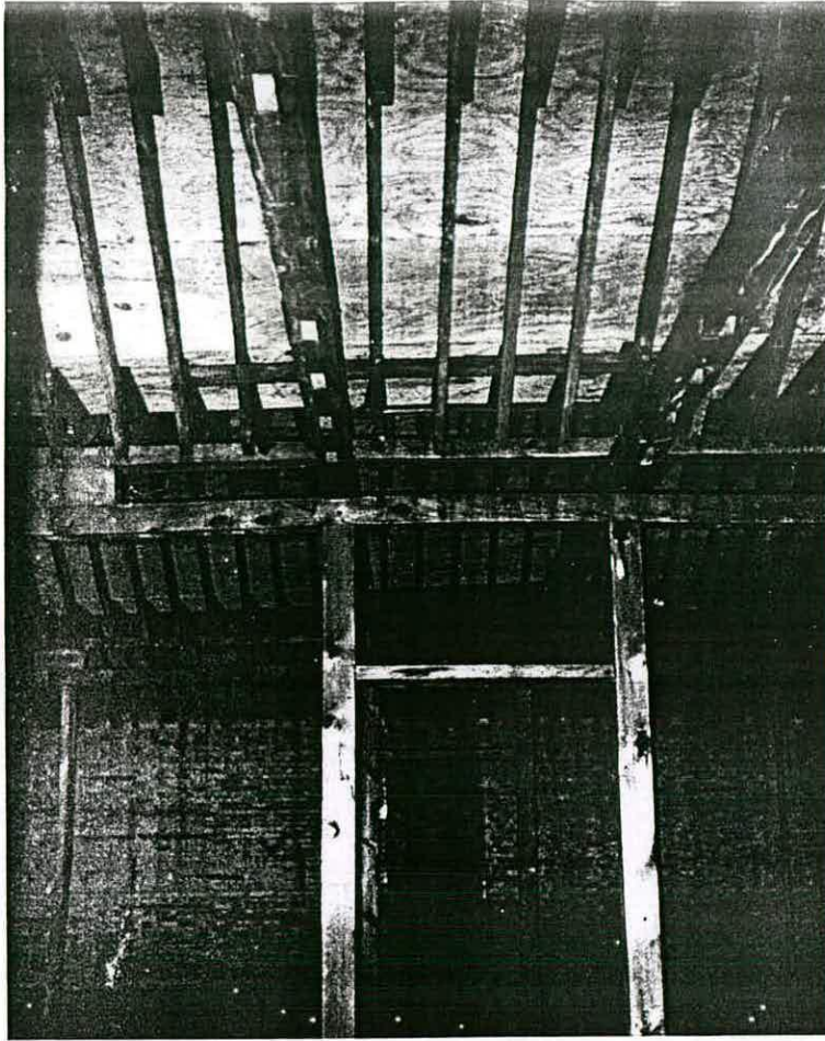
Marchwood: C Magazine, interior showing remains of barrel racks
