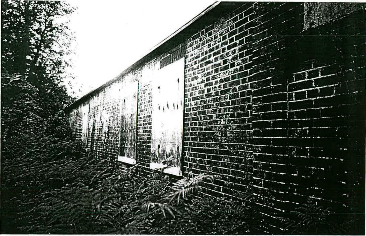
Marchwood: receiving rooms, inner side, to west
