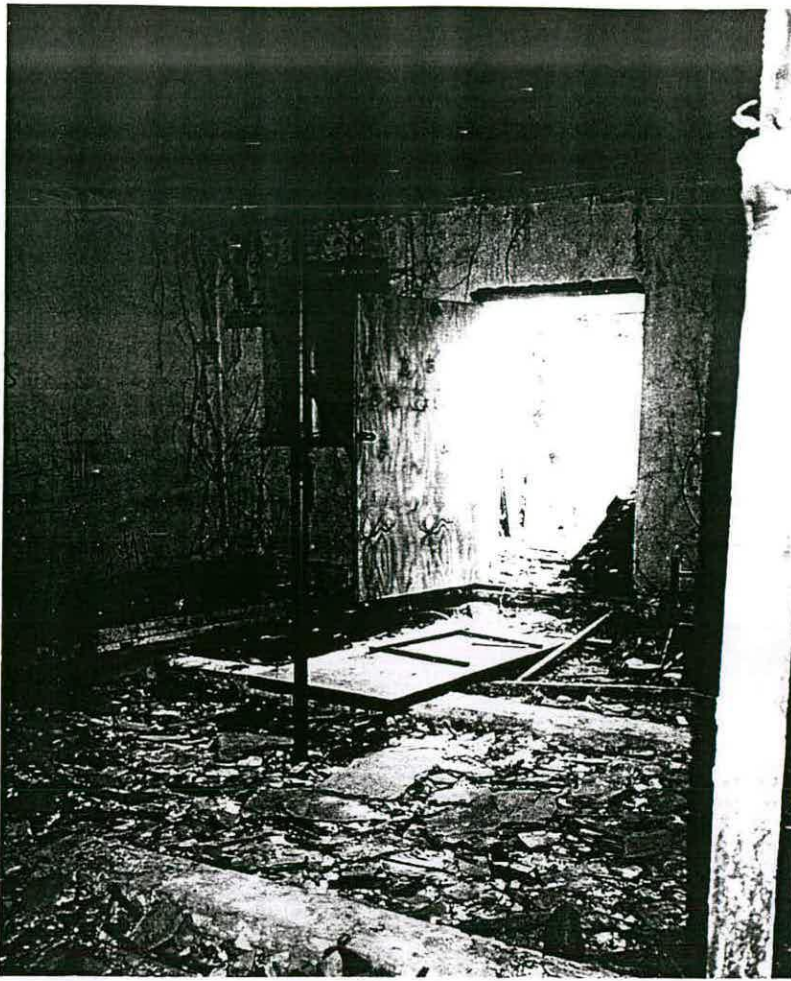
Marchwood: interior of former shifting house, to south
