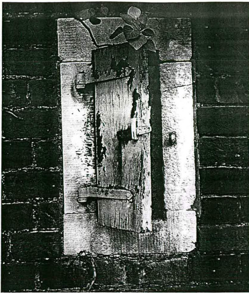
Marchwood: A Magazine, opening to ventilated wall, south side
