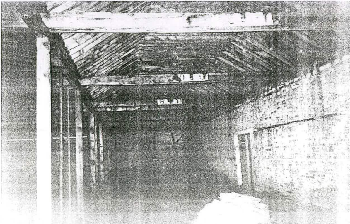
C Magazine: interior to east, showing numbered trusses
