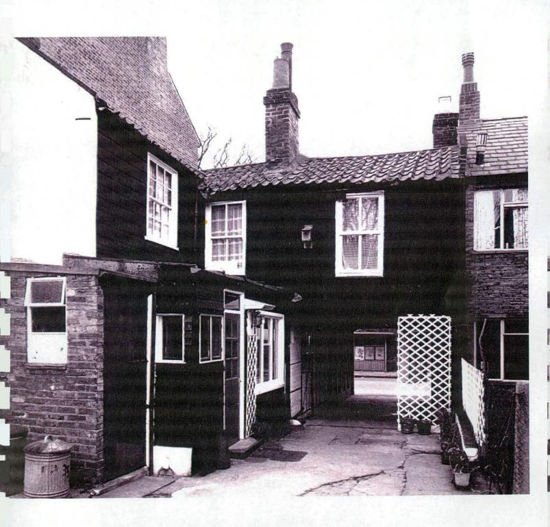
Fig. 5 Rear elevation showing original weather boarding and pan-tile roof 1970
