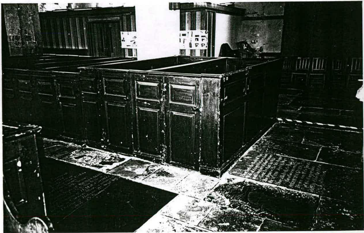
7 View of pews on north side of the nave, to the south-west
