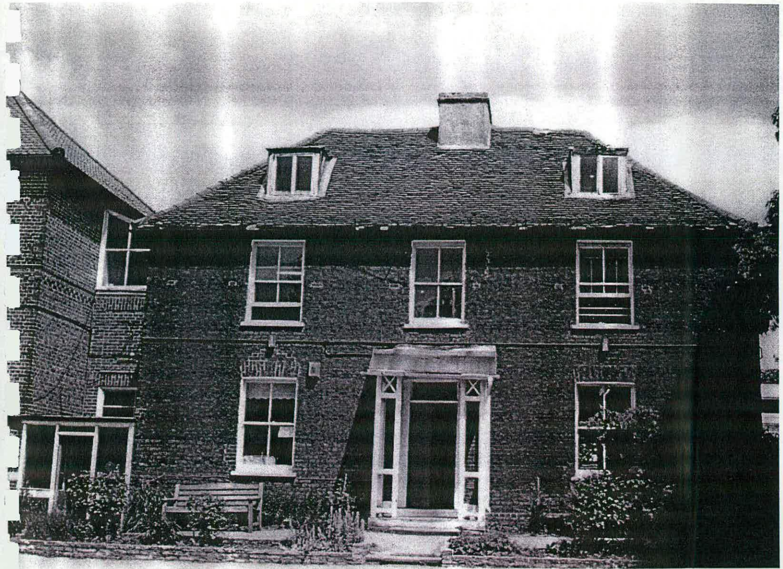
Main front range - elevation to Hale Lane.
