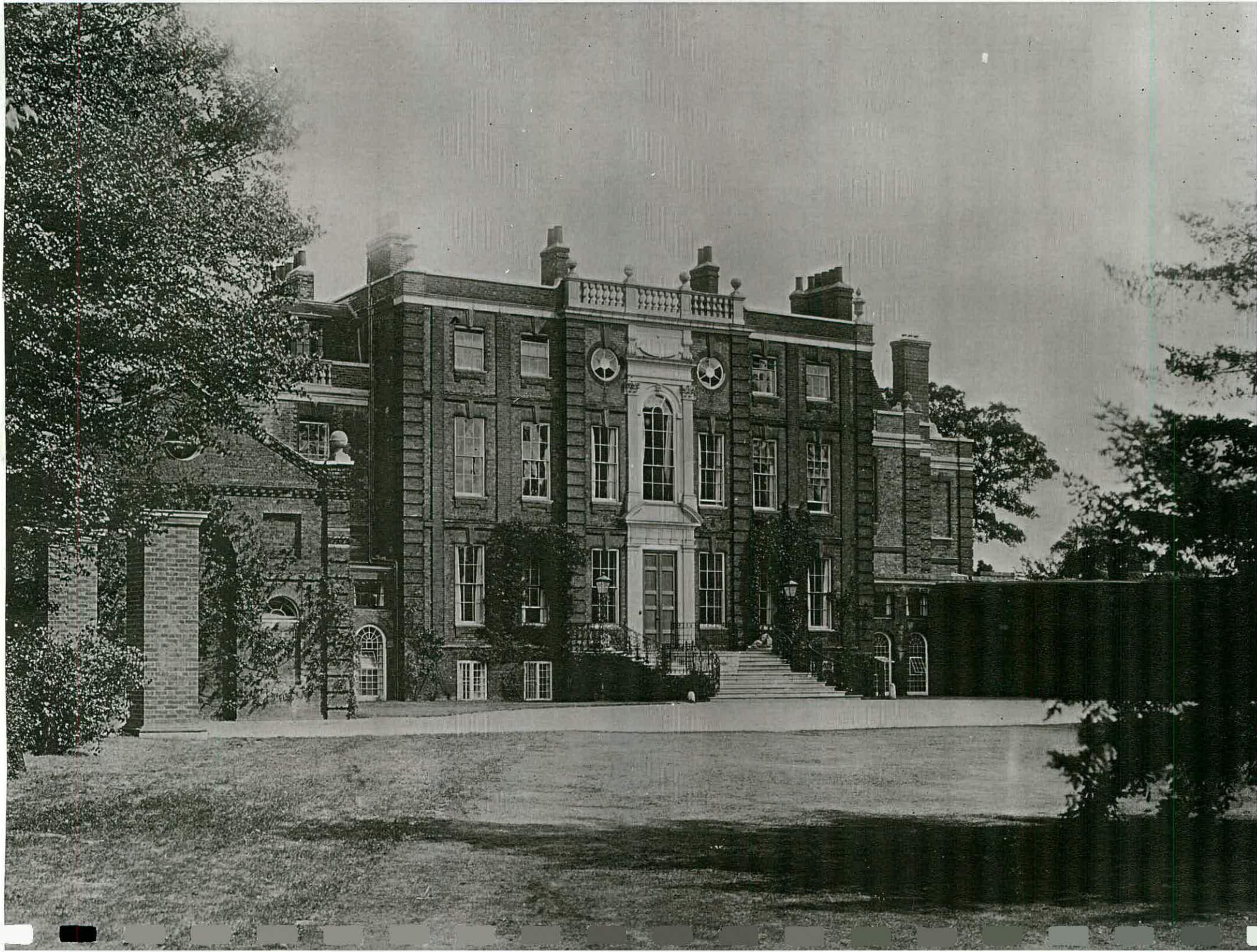
Figure 7. West front of Roehampton House, in c1900. Source: Greater London Record Office, GLC, Historic Buildings Division, photographic archive, F3685.
