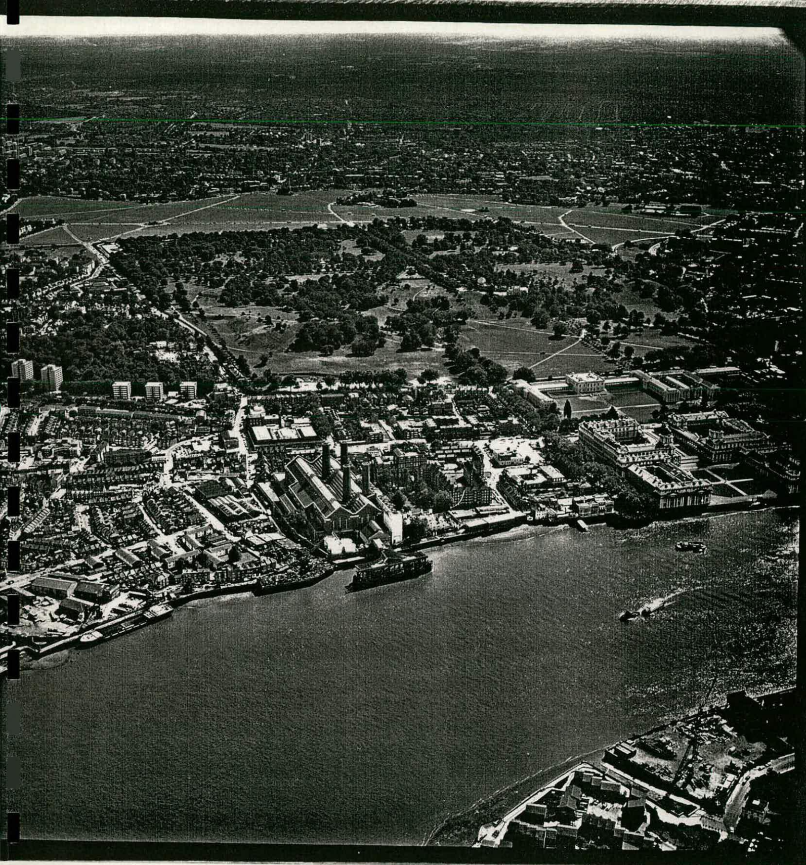
Greenwich Generating Station, aerial view from the north in 1987 (NMR 4007/63, TQ 878/9).
