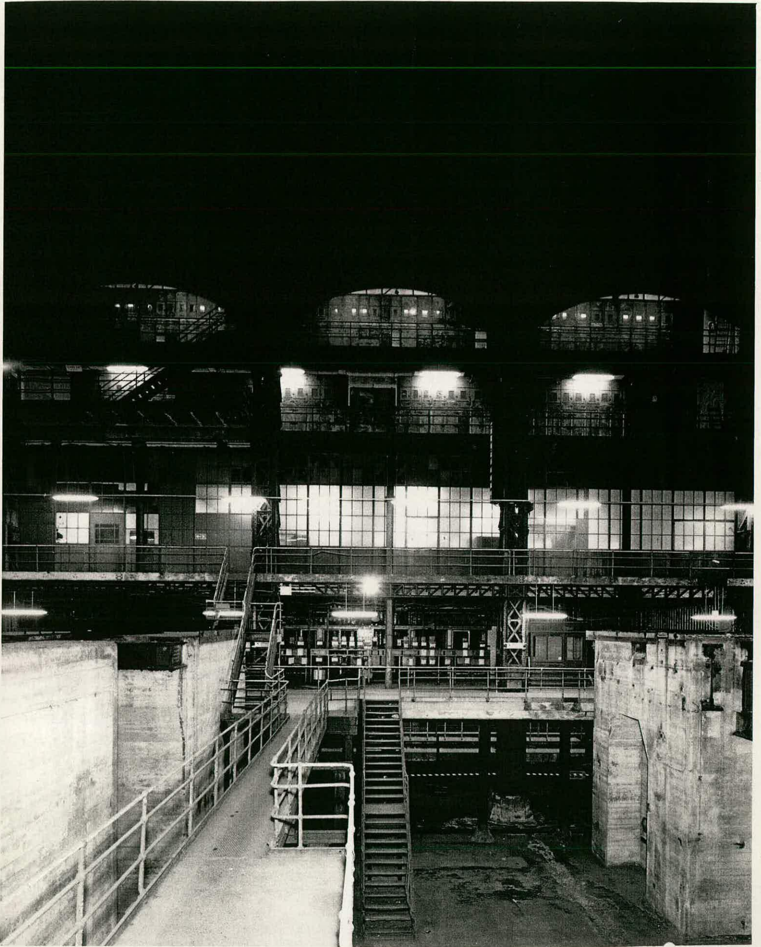
Greenwich Generating Station, view across the former engine room to the switchboard galleries (BB94/11439).
