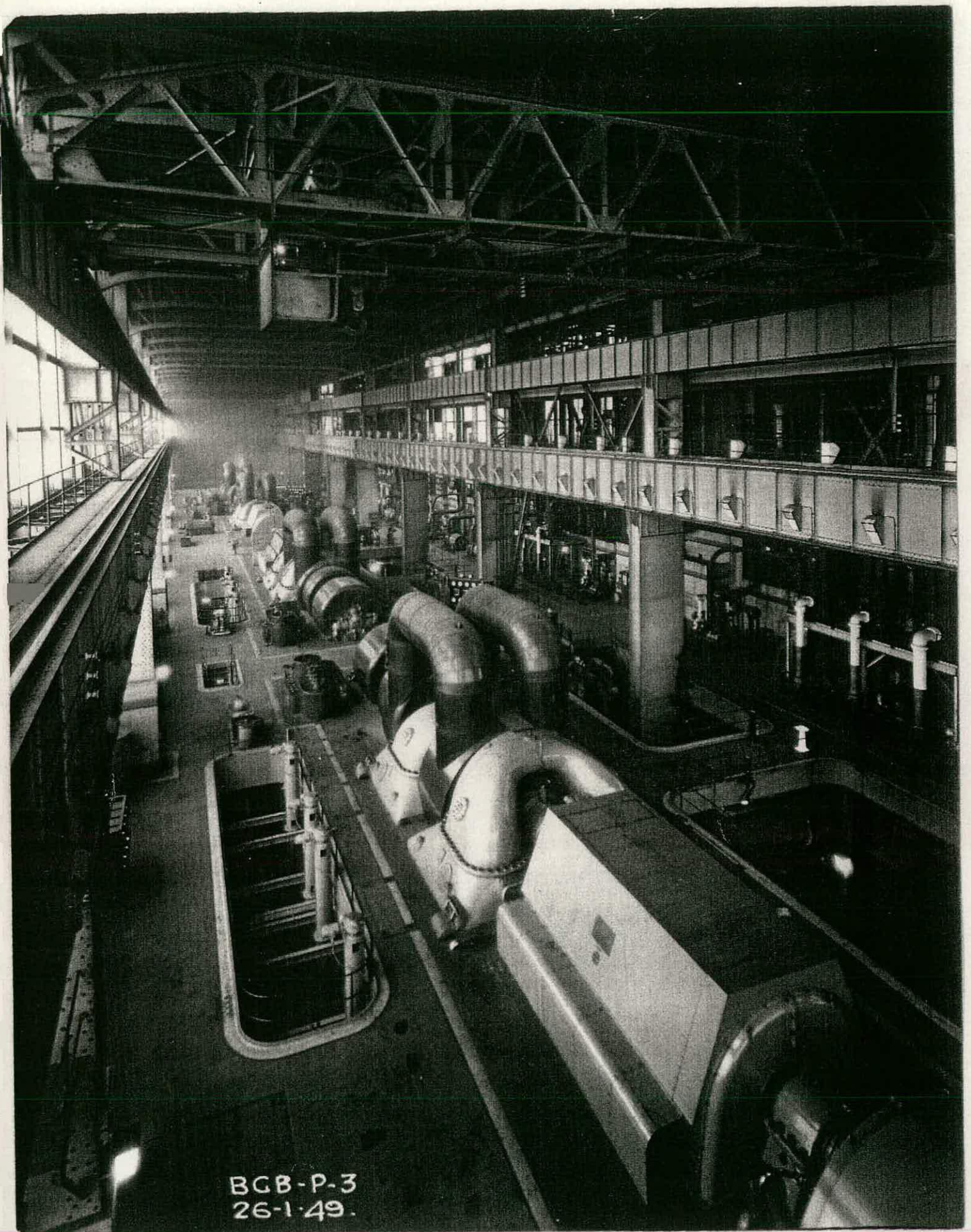
Barking Power Station, "B" Station turbine hall in 1949 (National Power plc).
