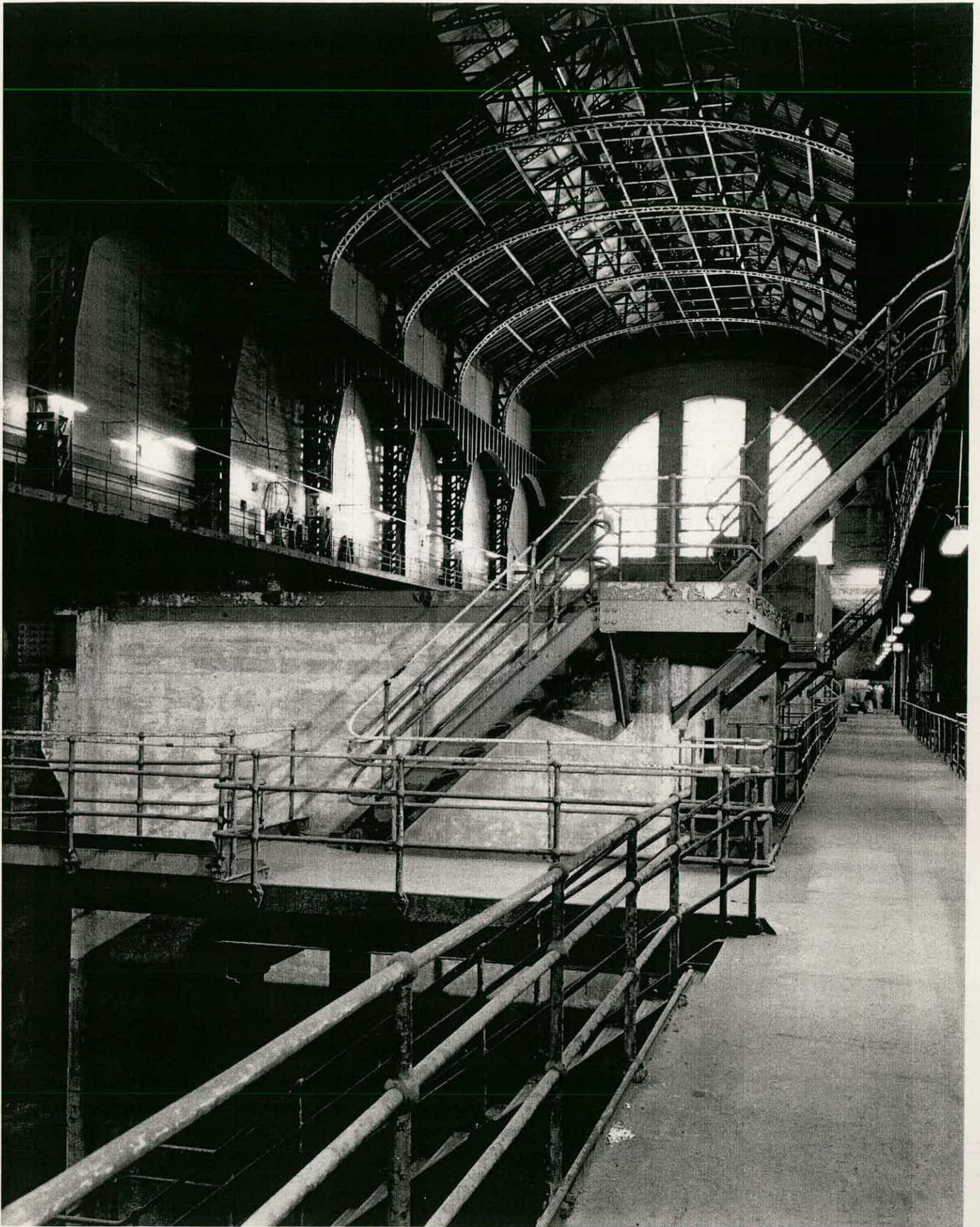
Greenwich Generating Station, the former engine room from the south in 1994 showing steel framing (BB94/11441).
