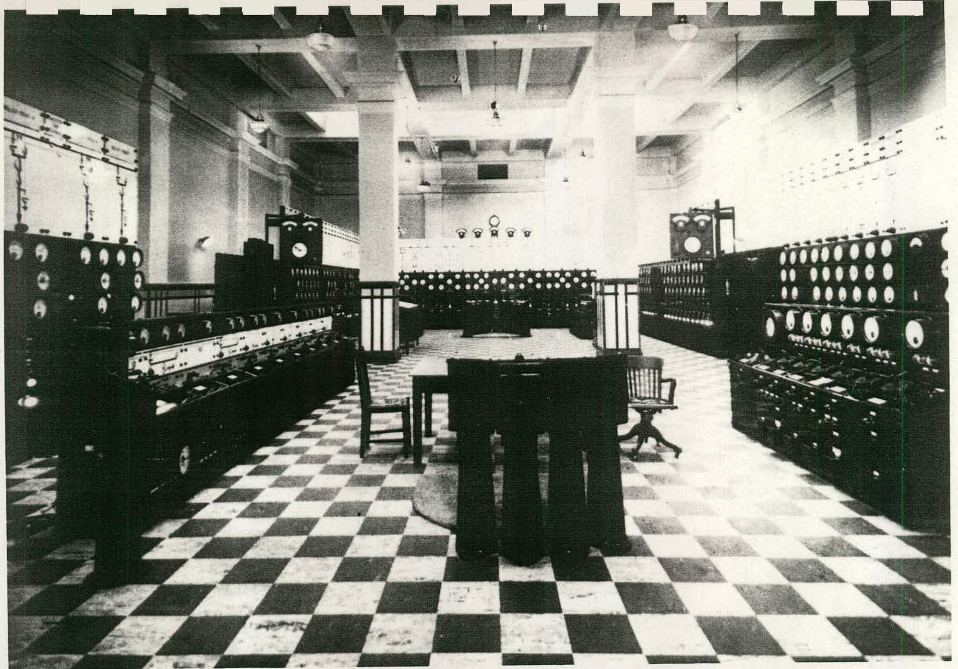
Barking Power Station, "A" Station control room c1928 (National Power plc).
