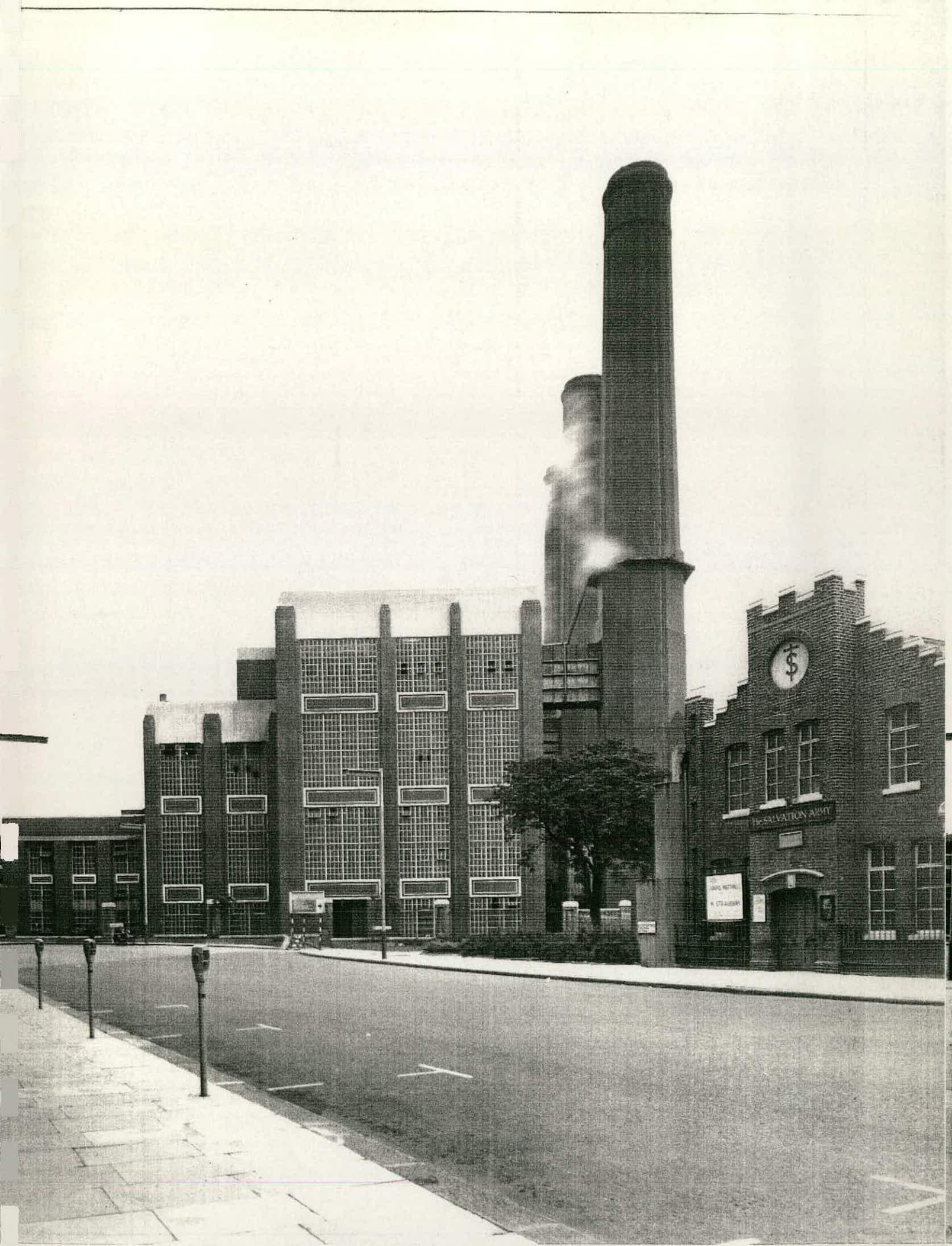
Woolwich Power Station from the south (National Power plc).
