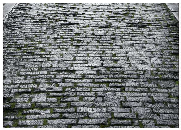
Figure 21: The timber setts in King Street (DP221833)
