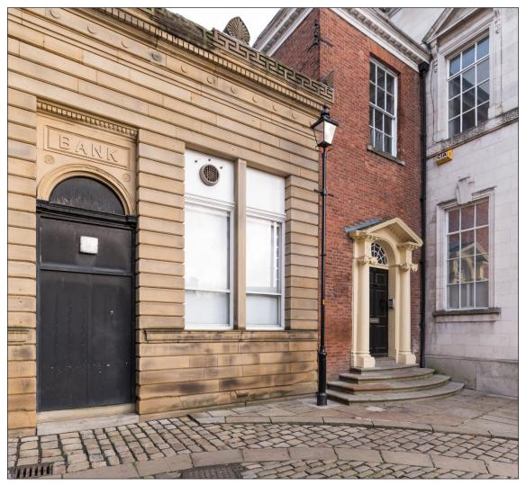
Figure 10: The Royds banking complex comprising the bank extension of 1879 beside the Georgian staircase bay of brick (with the doorcase relocated from the main house), and the corner of the main building which was refronted in Portland stone (DP235543)
